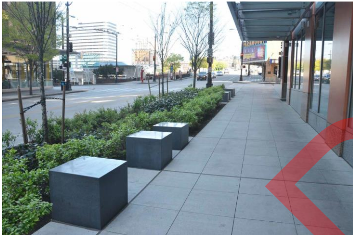
Repaved sidewalks and crosswalks
