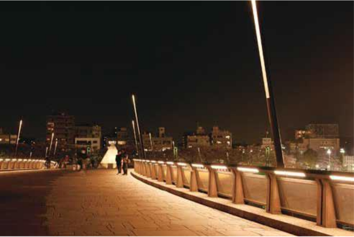
Higher overpass railings with integrated lighting
