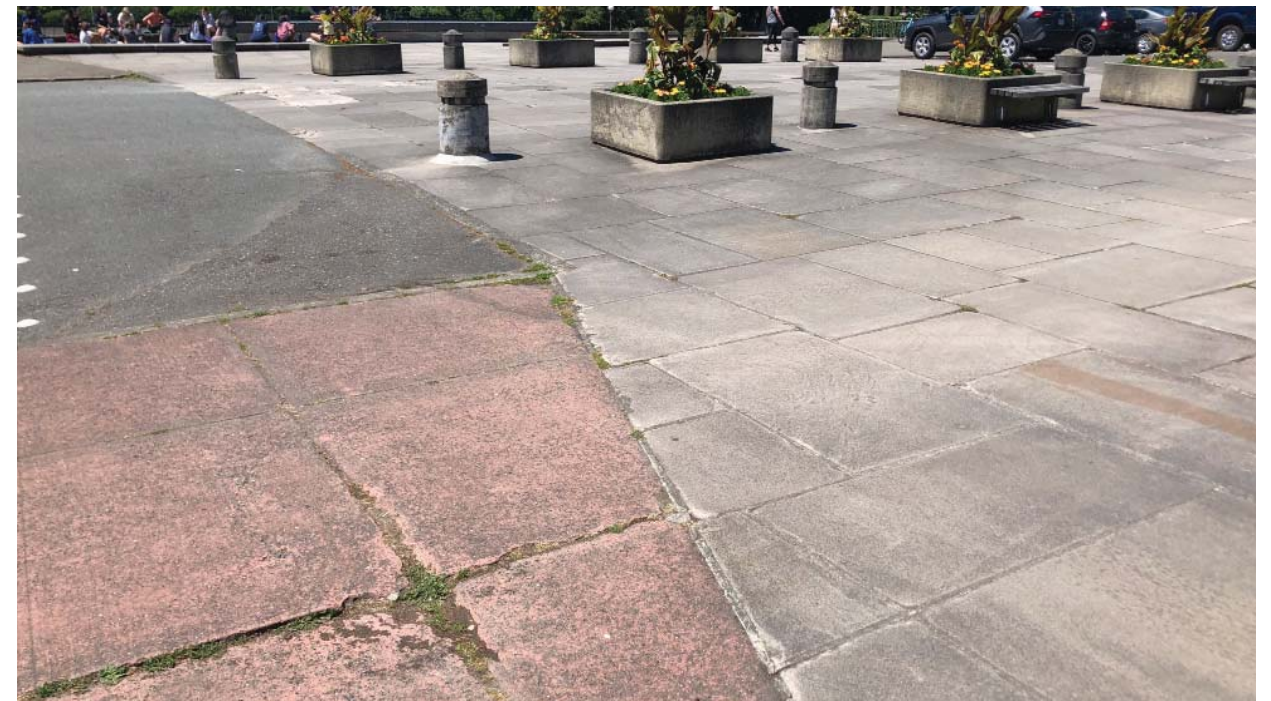
Existing pinkish concrete sidewalk at south edge of stone plaza shown as reference: apparent unsuccessful prior effort to match the pinkish cast in the stone.
