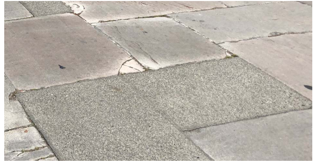
Existing Concete infill within stone paving. A slightly lighter gray color than the existing infill is proposed, with a finer grained etched finish. Note the color variation in surrounding stones.
