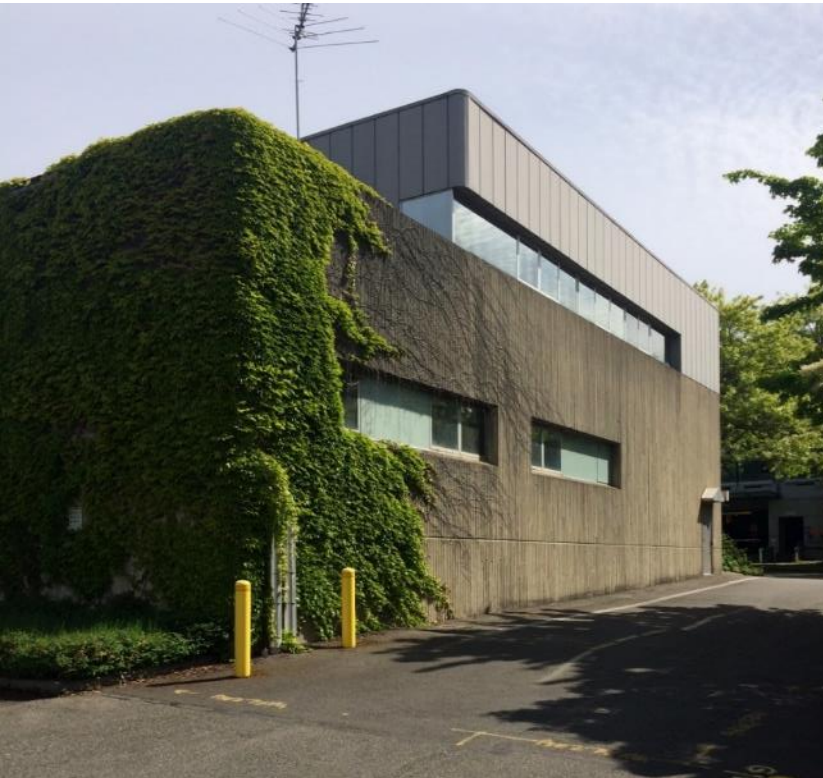
Figure 22. Below, looking northeast at the southwest corner of the building.
