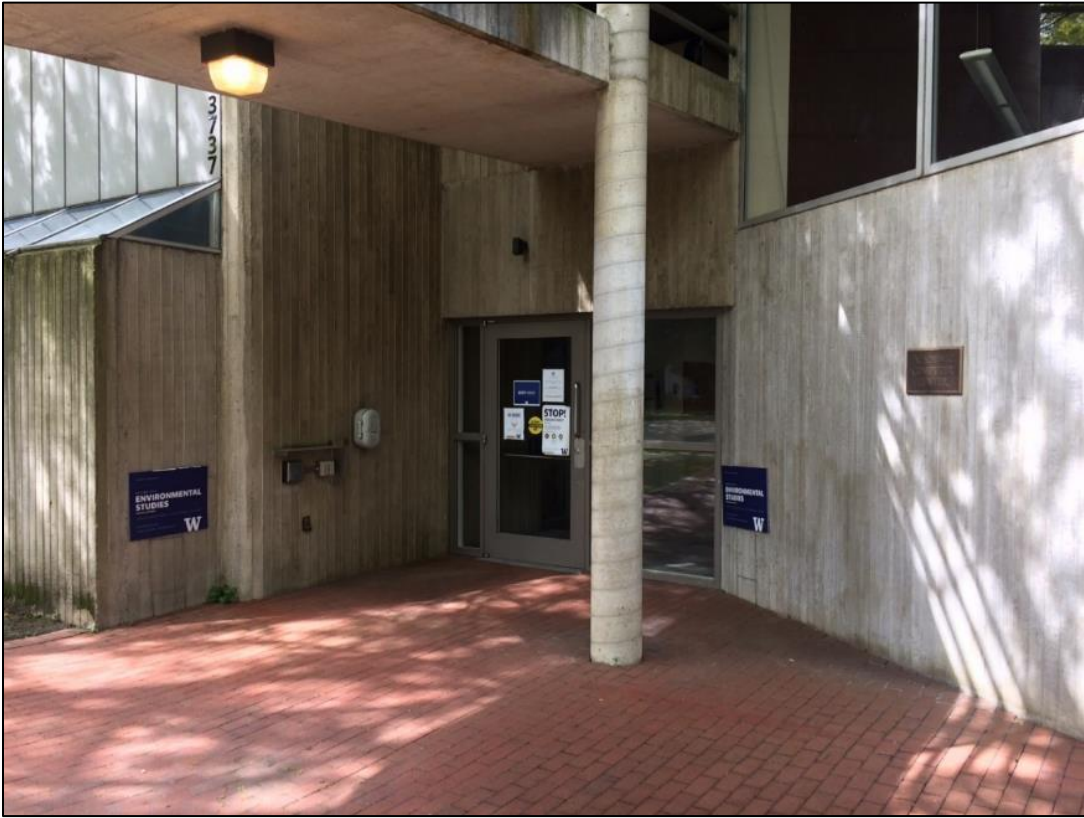
Entry views: Figure 27. Above, looking southwest at the east first floor recessed entry.
