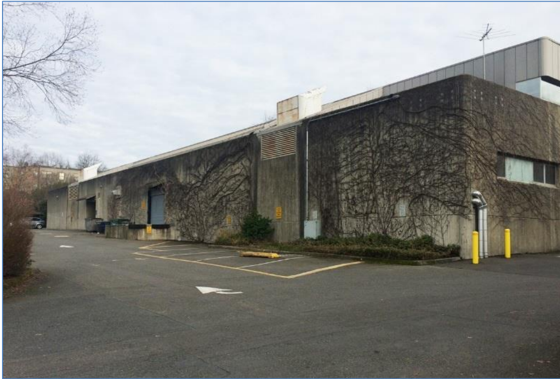
Figure 23. Above looking northeast at the west facade.
