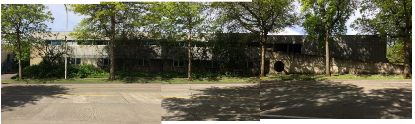
Figure 13. Above, a composite photo looking west at the east facade.
