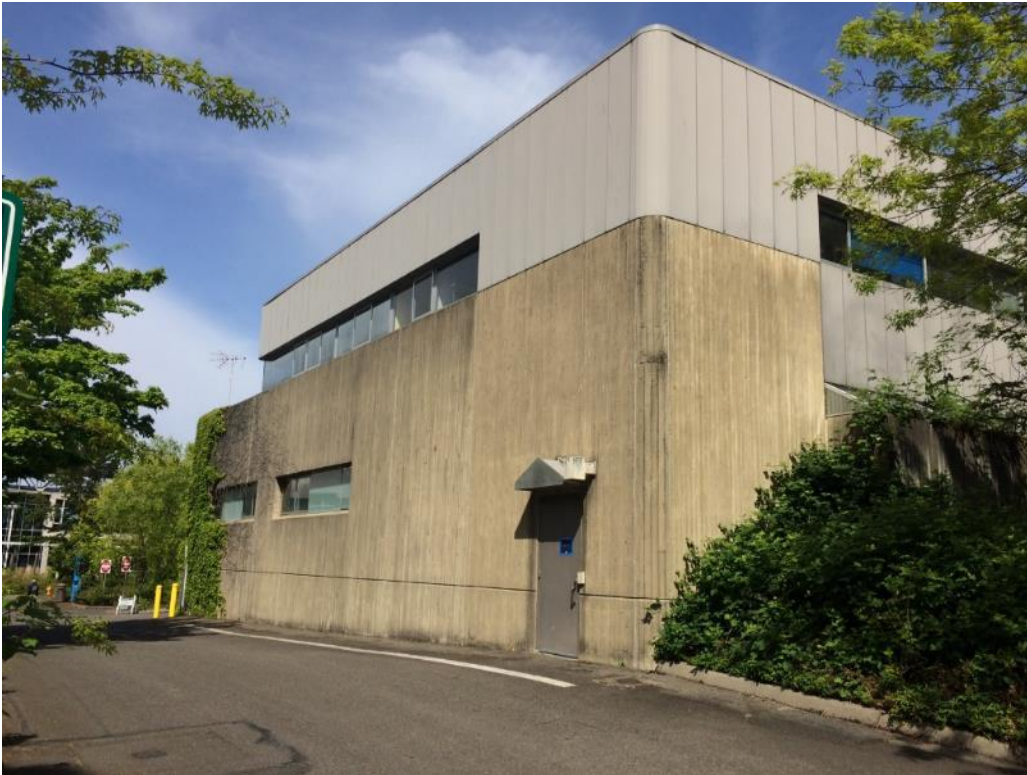
Figure 21. Above, looking northwest at the southeast corner and south façade.
