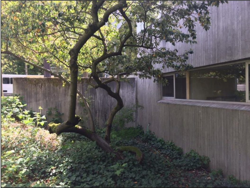
Figure 6. Above, looking eastward along the lower west part of the facade.
