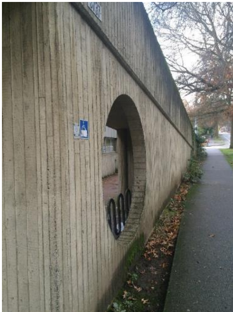
Figure 18 – 20. Ramp and entry views: Above right. East façade the floor entry. Below, the ramp structure and opening in the cast-in-place ramp wall.
