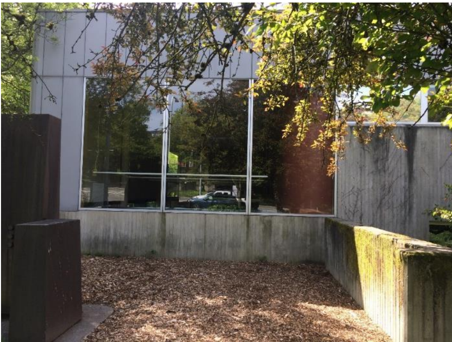
Figures 7. Detail view of windows on the east side of the north façade.
