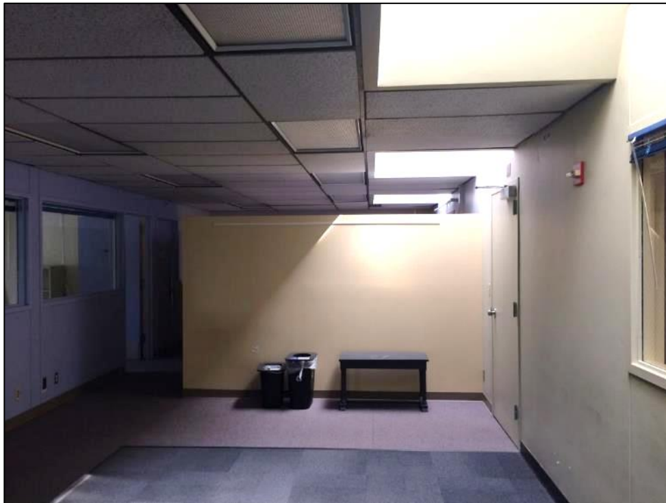
Figure 37. Below, an interior office on the second floor with indirect skylight illumination.
