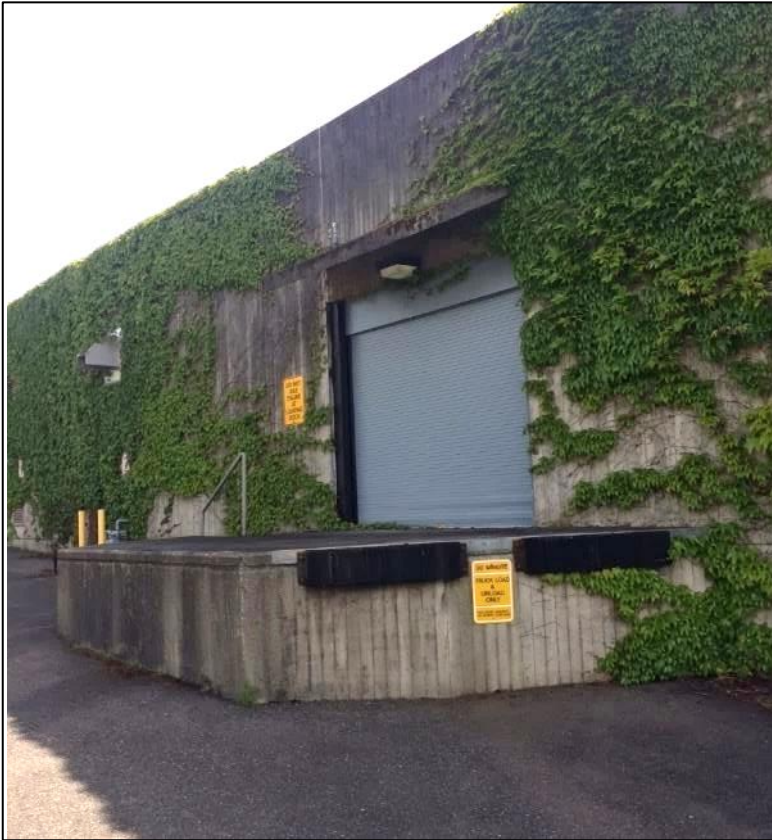
Figure 25. Above, the west loading dock.
