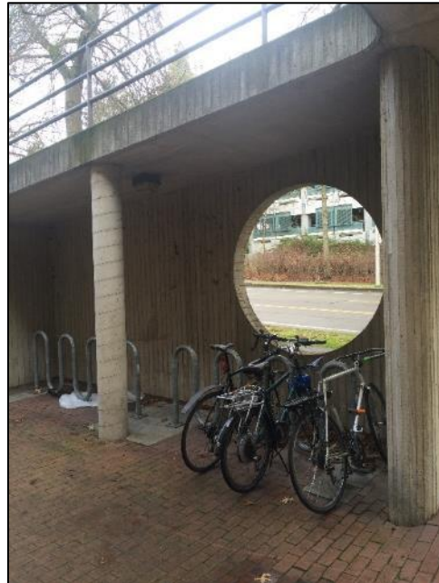
Figure 18 – 20. Ramp and entry views: Above right. East façade the floor entry. Below, the ramp structure and opening in the cast-in-place ramp wall.
