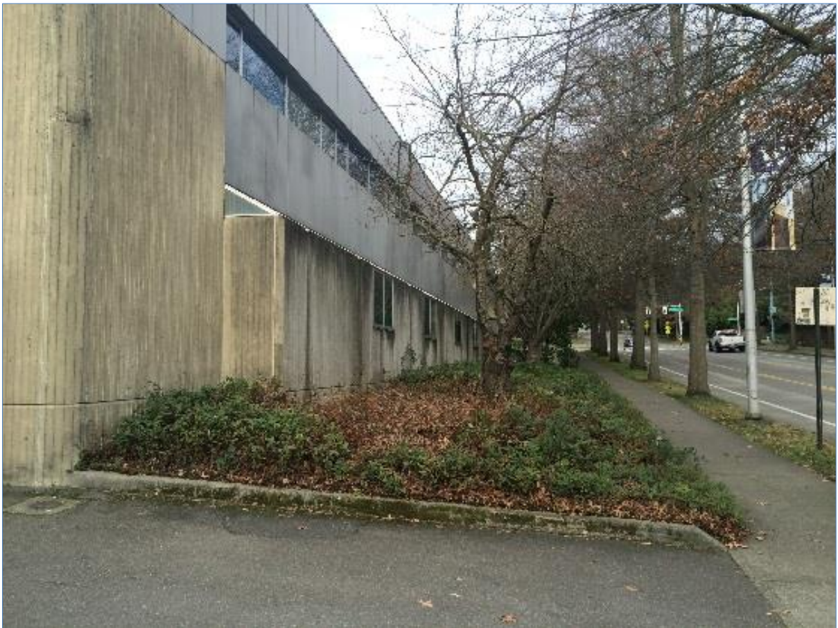
Figures 14. Below, looking north along the east façade, west setback and plant bed and Brooklyn Avenue NE.
