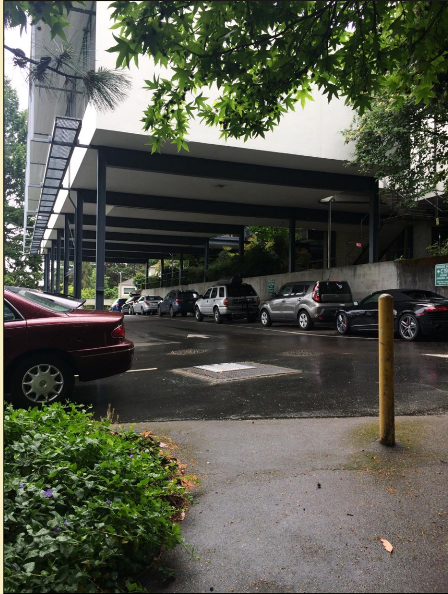
East Parking Area below the Dining Room
