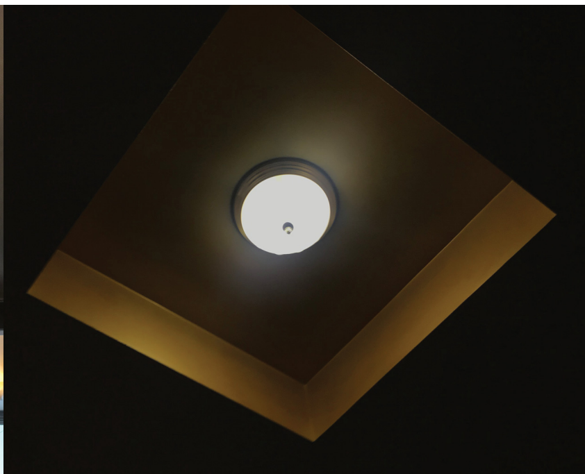
EXISTING CEILING MOUNT FIXTURE IN RECESSED COFFER
