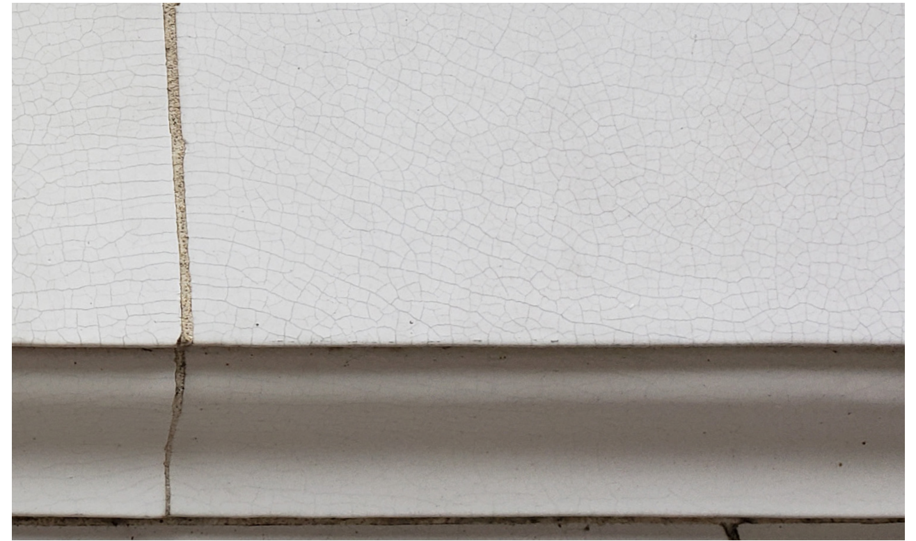
Spiderwebbing: Reglaze to Seal
