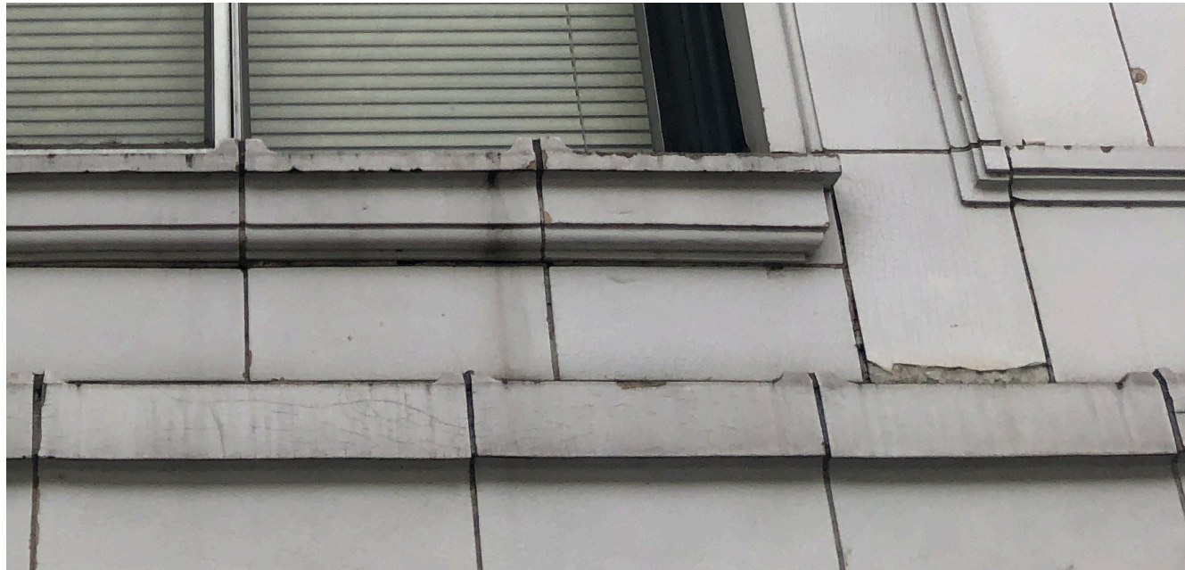
Replace Spalling Terracotta
