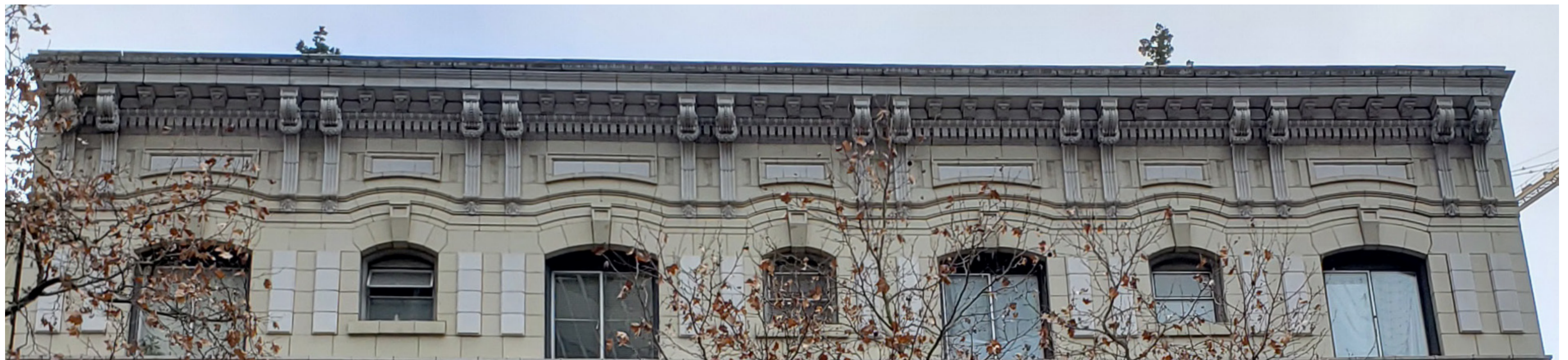
Remove & Resecure Cornice Elements
