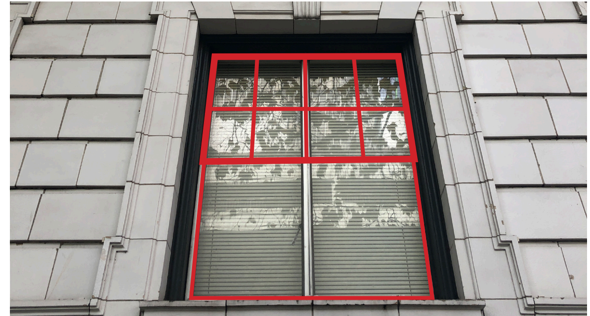
Install Wood Clad True Divided Lite Upper Sash Windows
