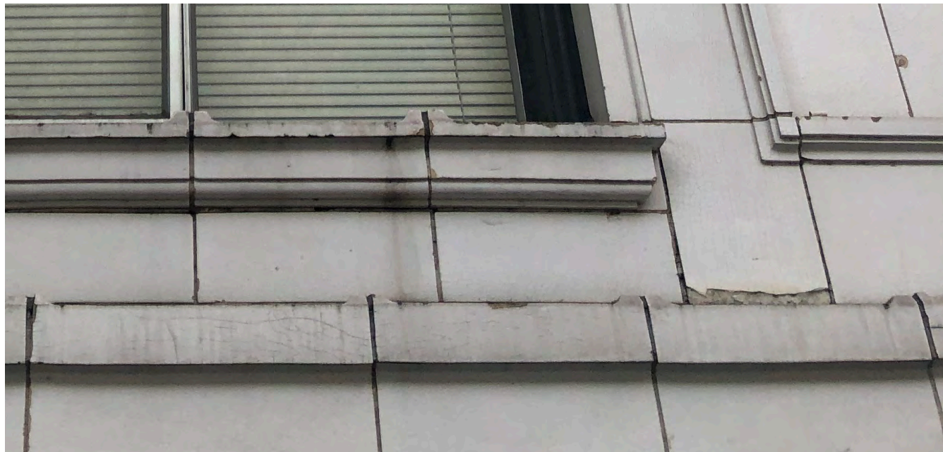
Replace Spalling Terracotta
