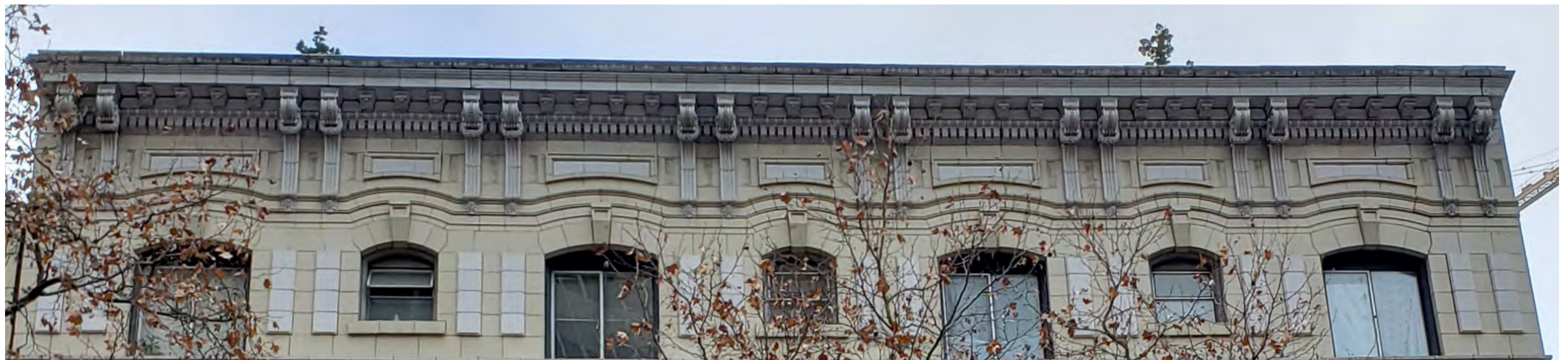
Remove & Resecure Cornice Elements
