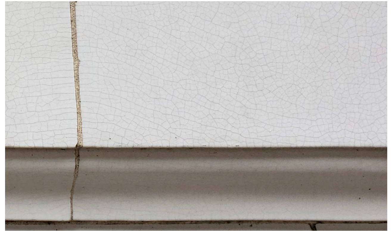
Spiderwebbing: Reglaze to Seal
