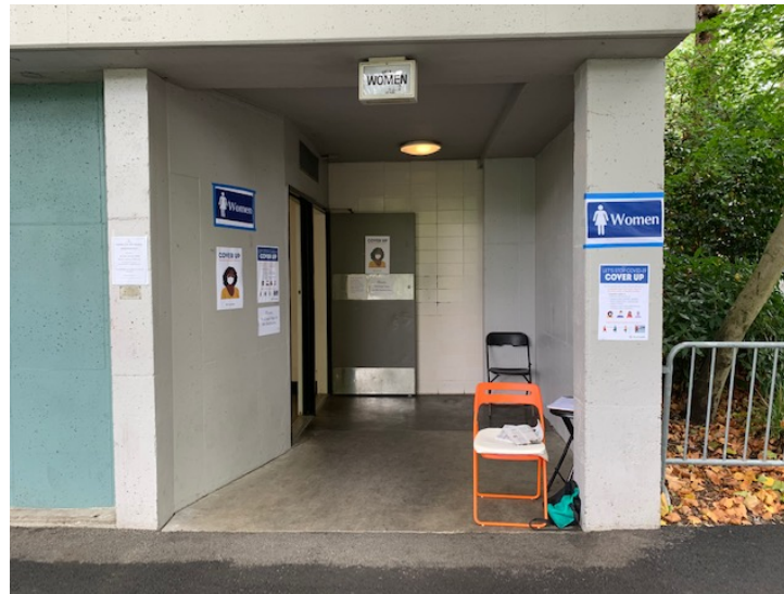
Alki Restrooms – entry alcove
