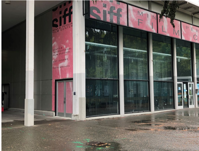
Alki Room/SIFF – SW corner
