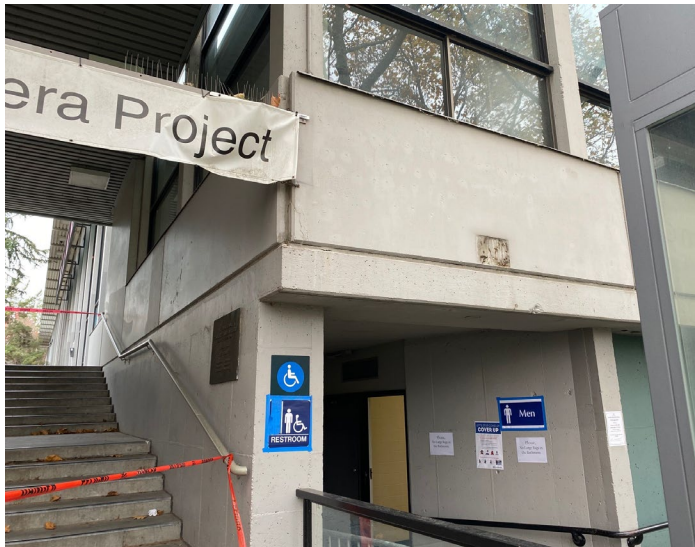
Alki Restrooms – entry alcove
