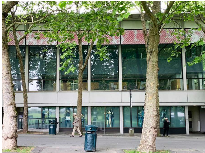
Condition in April 2020, before Pool removal
