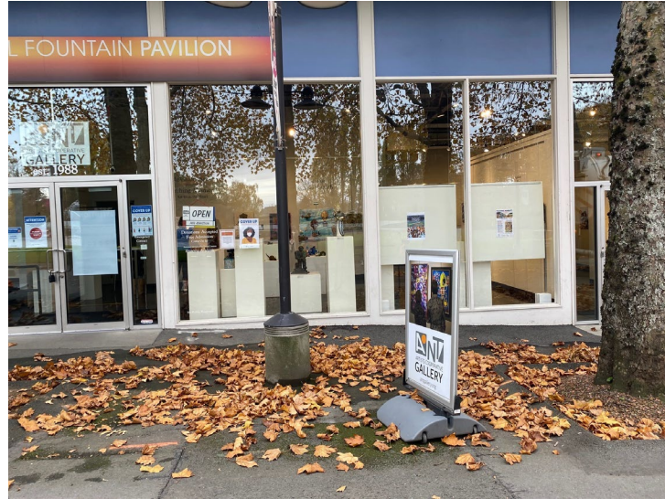
Intl. Fountain Pavilion - A/NT Gallery east side
