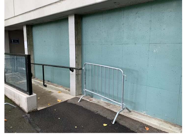
Alki Restrooms front face - detail
