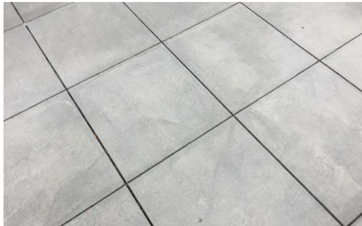
Concrete paving with sawcut joints
