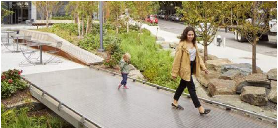
The pedestrian experience at the corner of Eastlake Ave E and Fairview Ave N is enhanced by bioretention planters. The terraced planters detain stormwater from the new parking garage and flow into one another via functional weirs. A grated walkway extends over the first planter in the series of three, providing access to the parking garage and concrete stairs down to Fairview Ave N.
