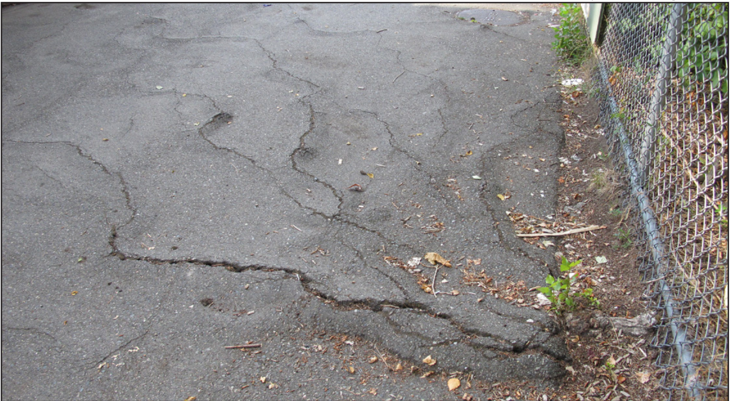
Figure 23 • Kimball Elementary, southern side, detail of root damage to asphalt
