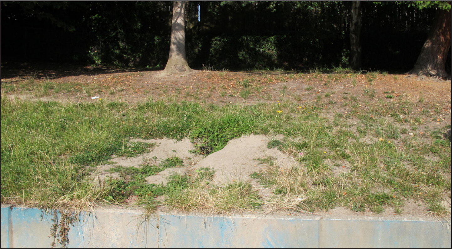
Figure 24 • Kimball Elementary, southern side, detail of water leak area above retaining wall
