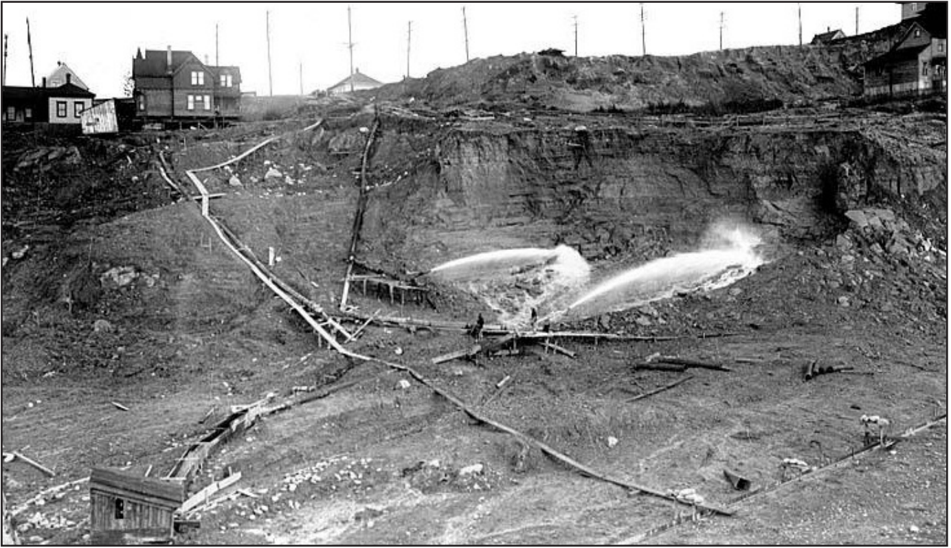
Figure 67 • Sluicing on Beacon Hill using hydraulic giants, n.d.
