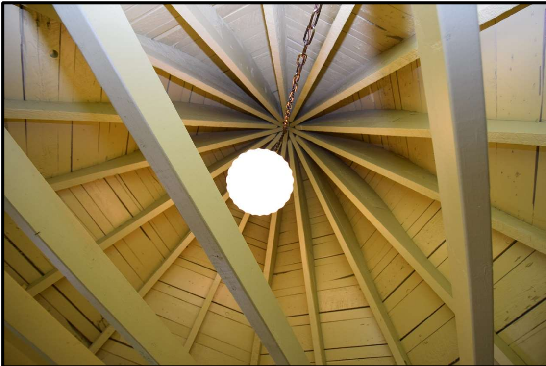
Figure 122: Detail view of framing at turret roof.
