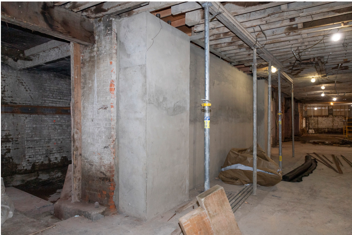
PHOTO 5. After: 2022 basement, Braced Frame 1, concrete portion completed.
