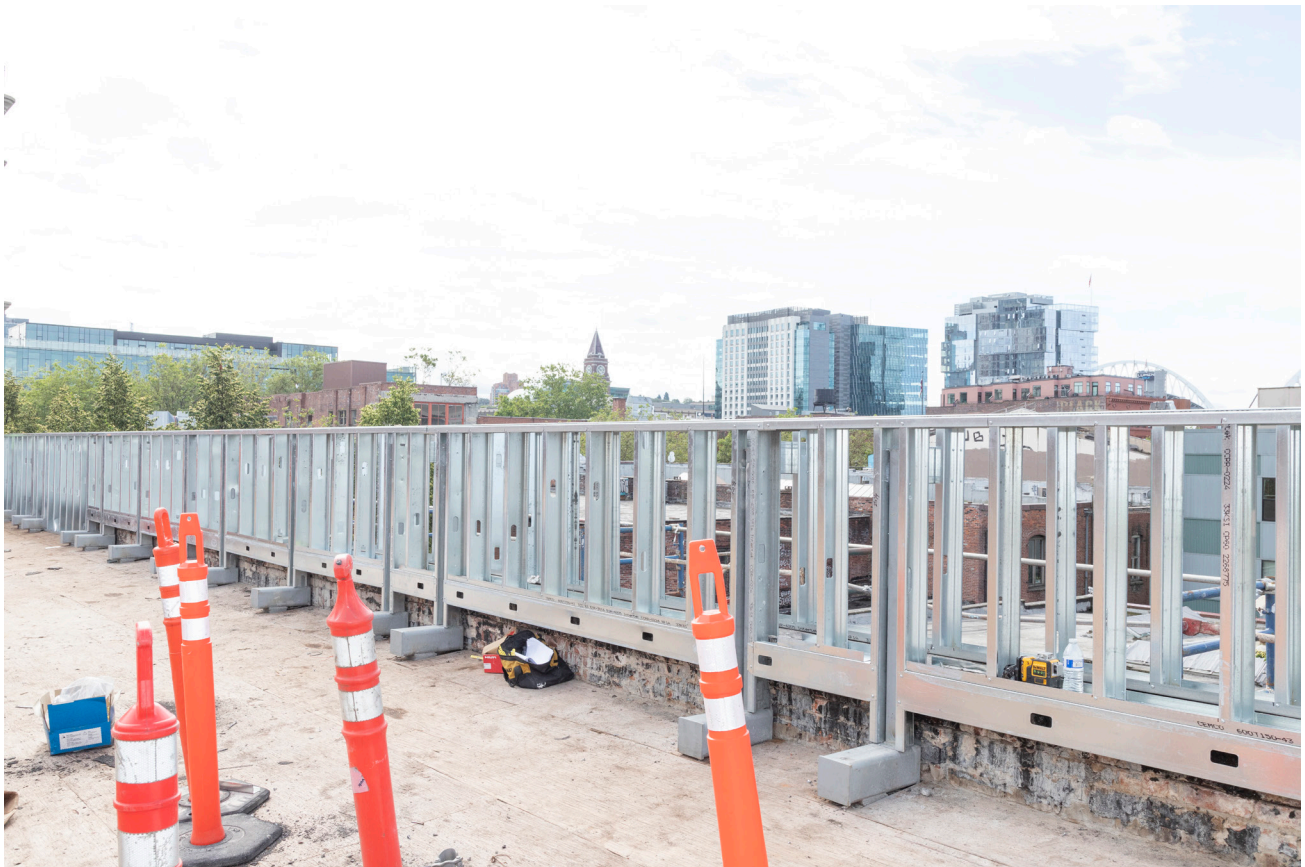
PHOTO 29. After: 2022 roof, showing metal framing completed for parapet reconstruction.
