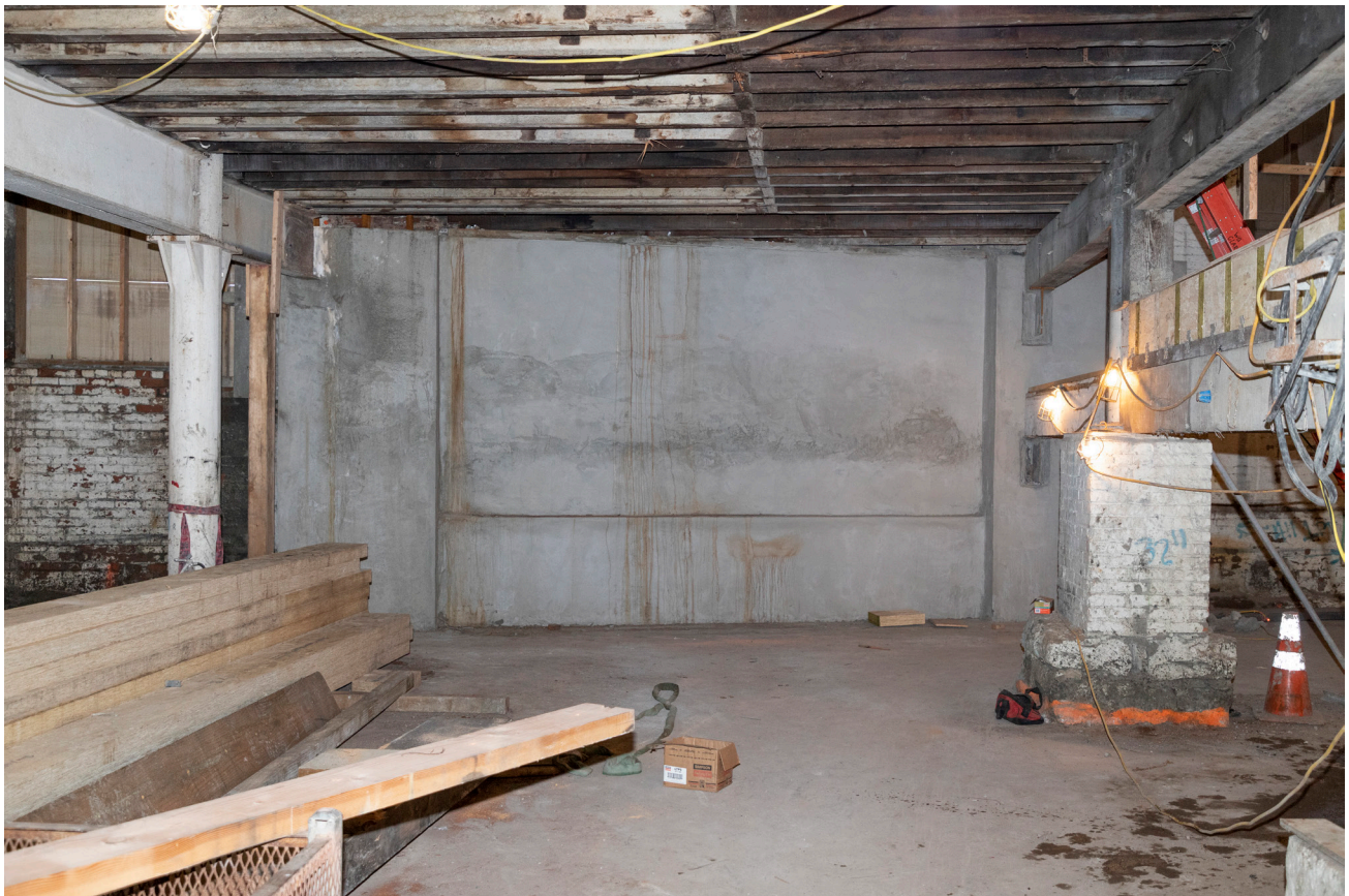
PHOTO 7. After: 2022 basement, Braced Frame 2, concrete portion complete.
