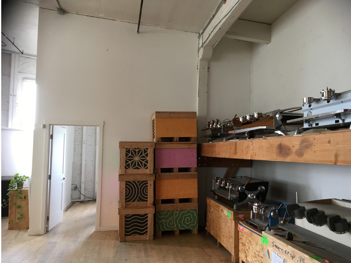
PHOTO 24. Before: 2020 third floor, office space, looking west. Source BuildingWork.
