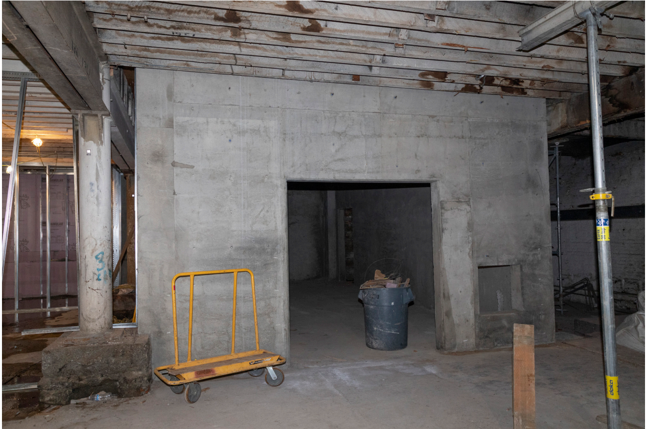
PHOTO 6. After: 2022 basement, electrical vault complete.
