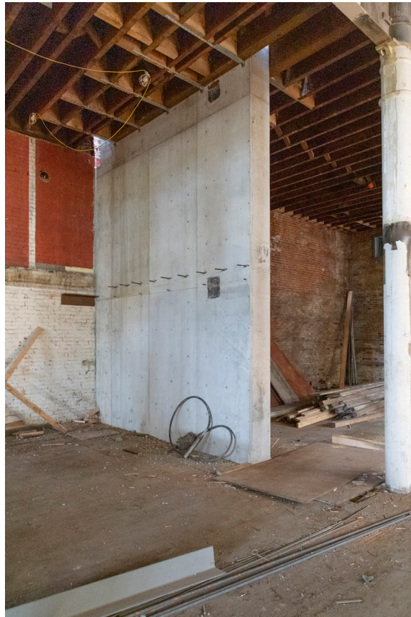
PHOTO 13. After: first floor, 2022, completed Shear Wall 2.
