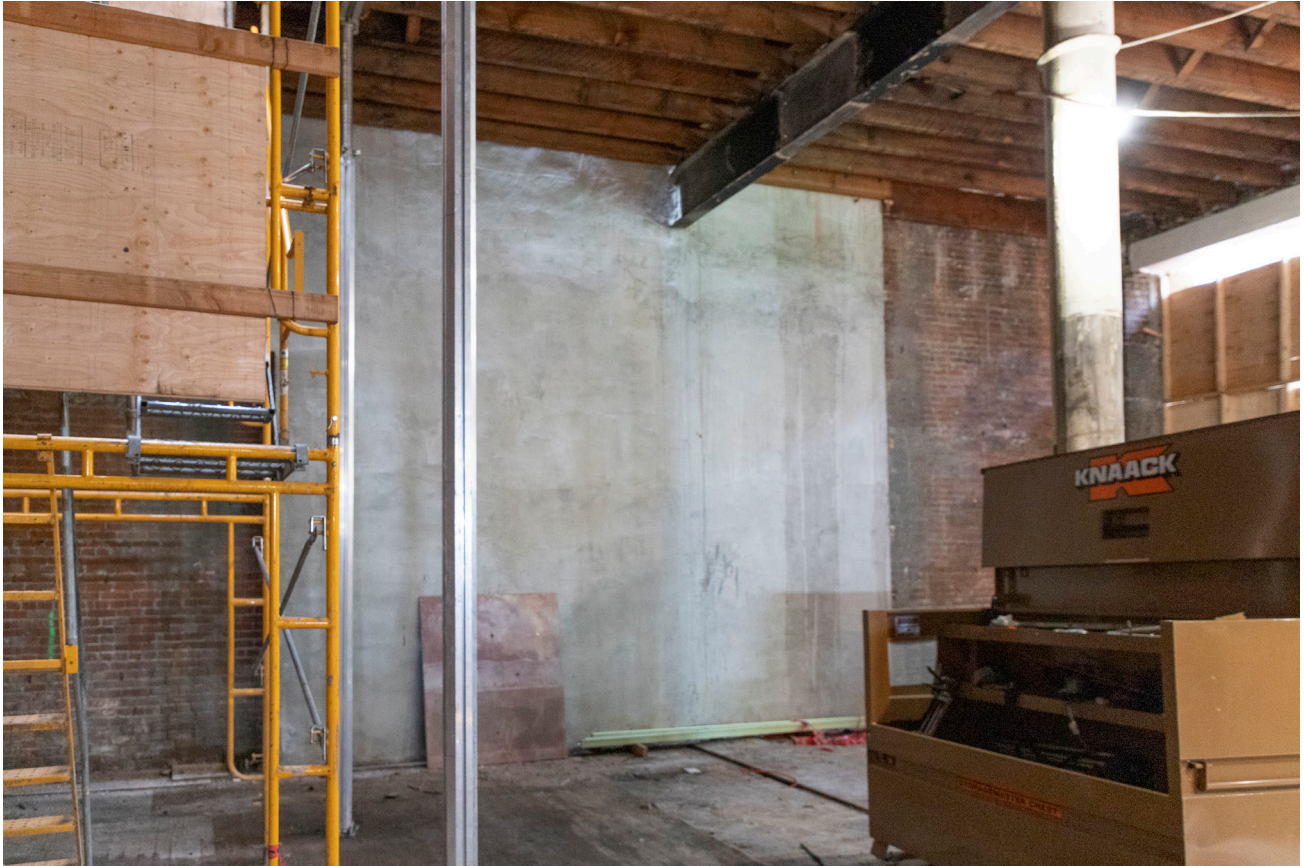
PHOTO 14. After: first floor, 2022, completed Shear Wall 1.
