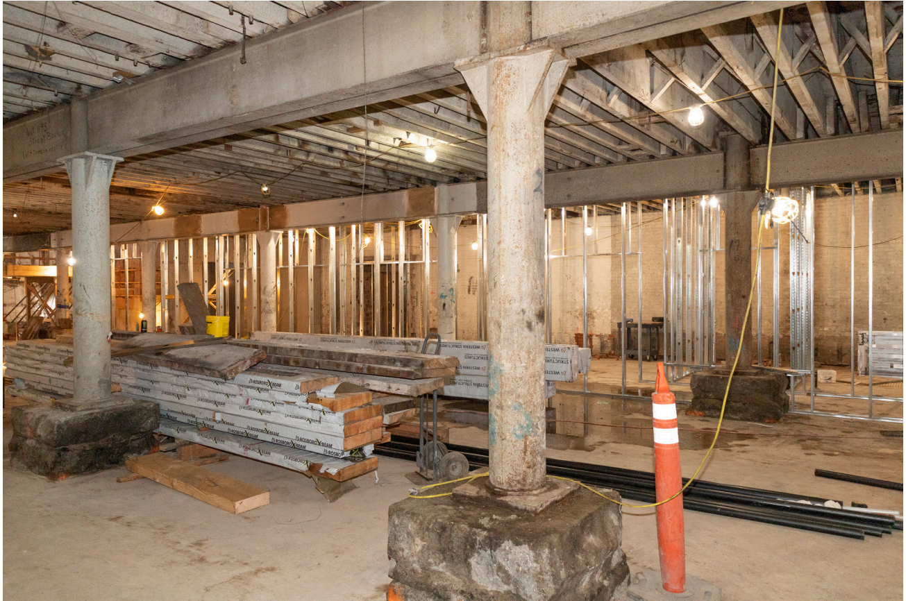
PHOTO 8. After: 2022 basement, selective demolition complete, interior framing in progress.
