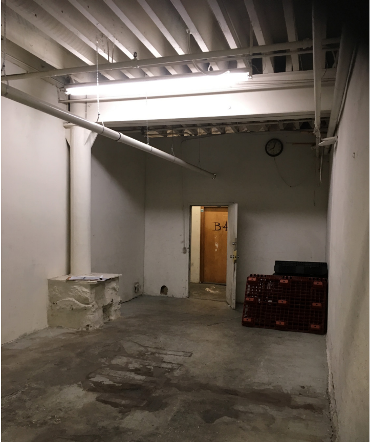
PHOTO 3. Before: 2020 basement, storage space, looking north, showing stone plinth below cast iron column. Source BuildingWork.
