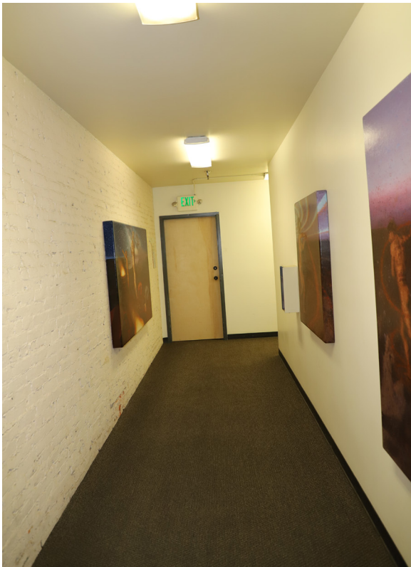
PHOTO 18. Before: 2020 second floor, north corridor, east end.
