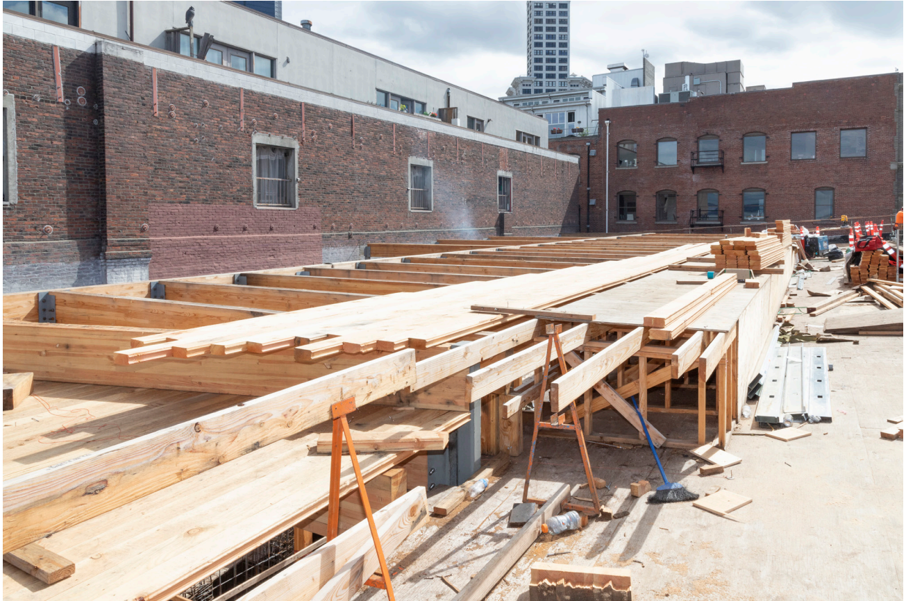
PHOTO 28. After: 2022 roof, showing roof portion removal and roof framing in progress.
