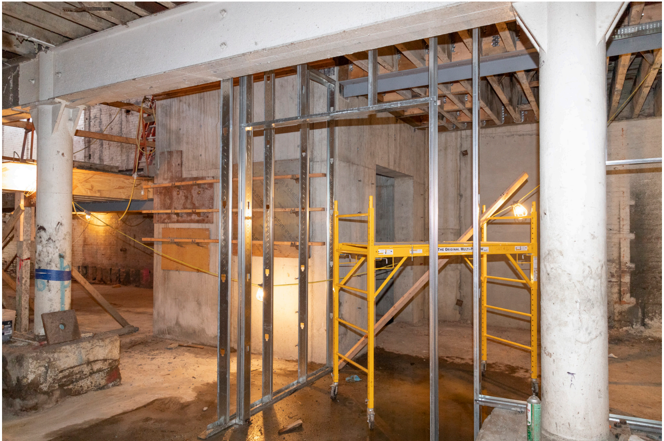
PHOTO 9. After: 2022 basement, elevator core and shear walls 3-6, concrete completed.
