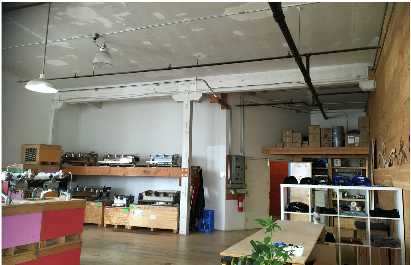
PHOTO 25. Before: 2020 third floor, office space, looking north. Source BuildingWork.
