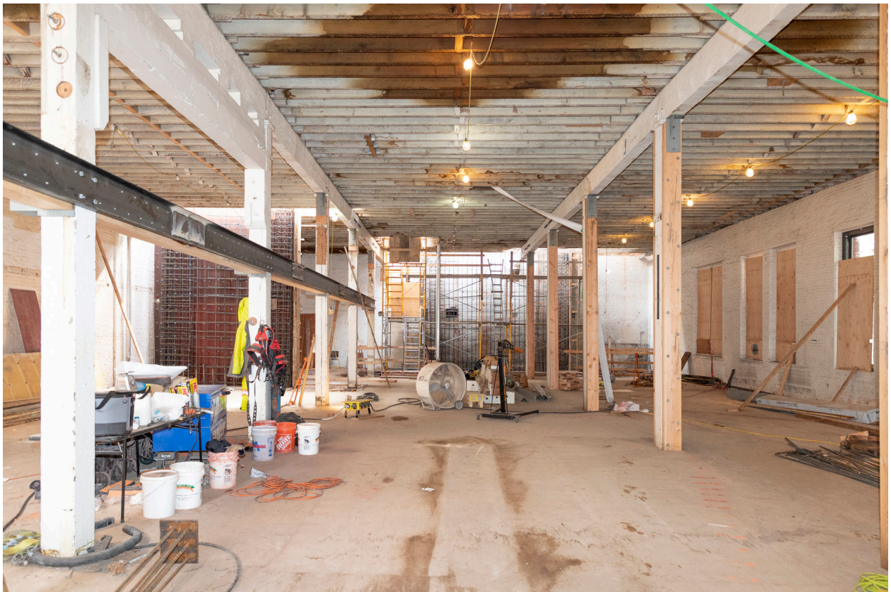
PHOTO 23. After: 2022 second floor, steel seismic reinforcing attached to columns.
