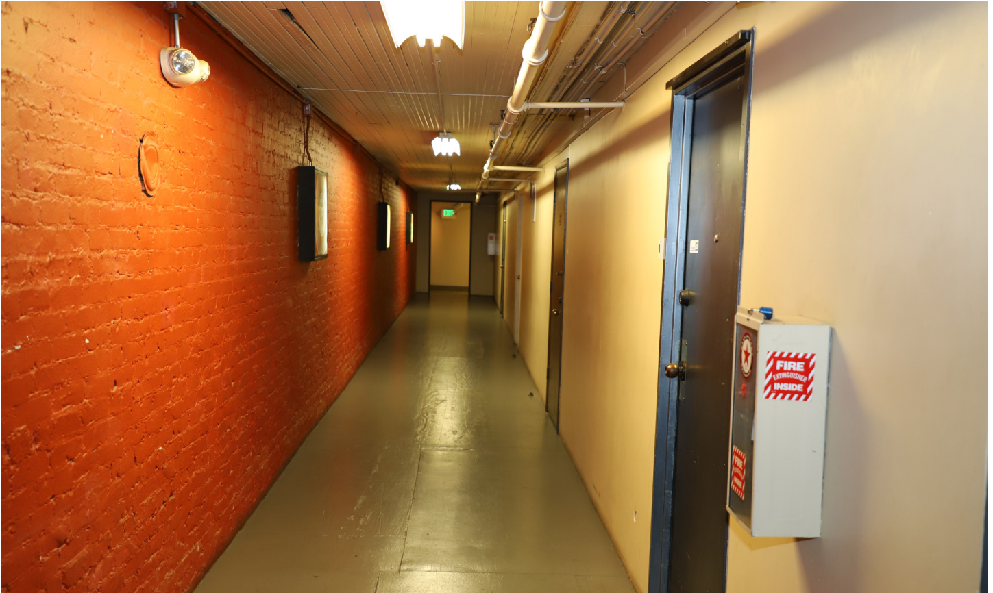
PHOTO 10. Before: 2020 mezzanine, looking south along the north corridor.
