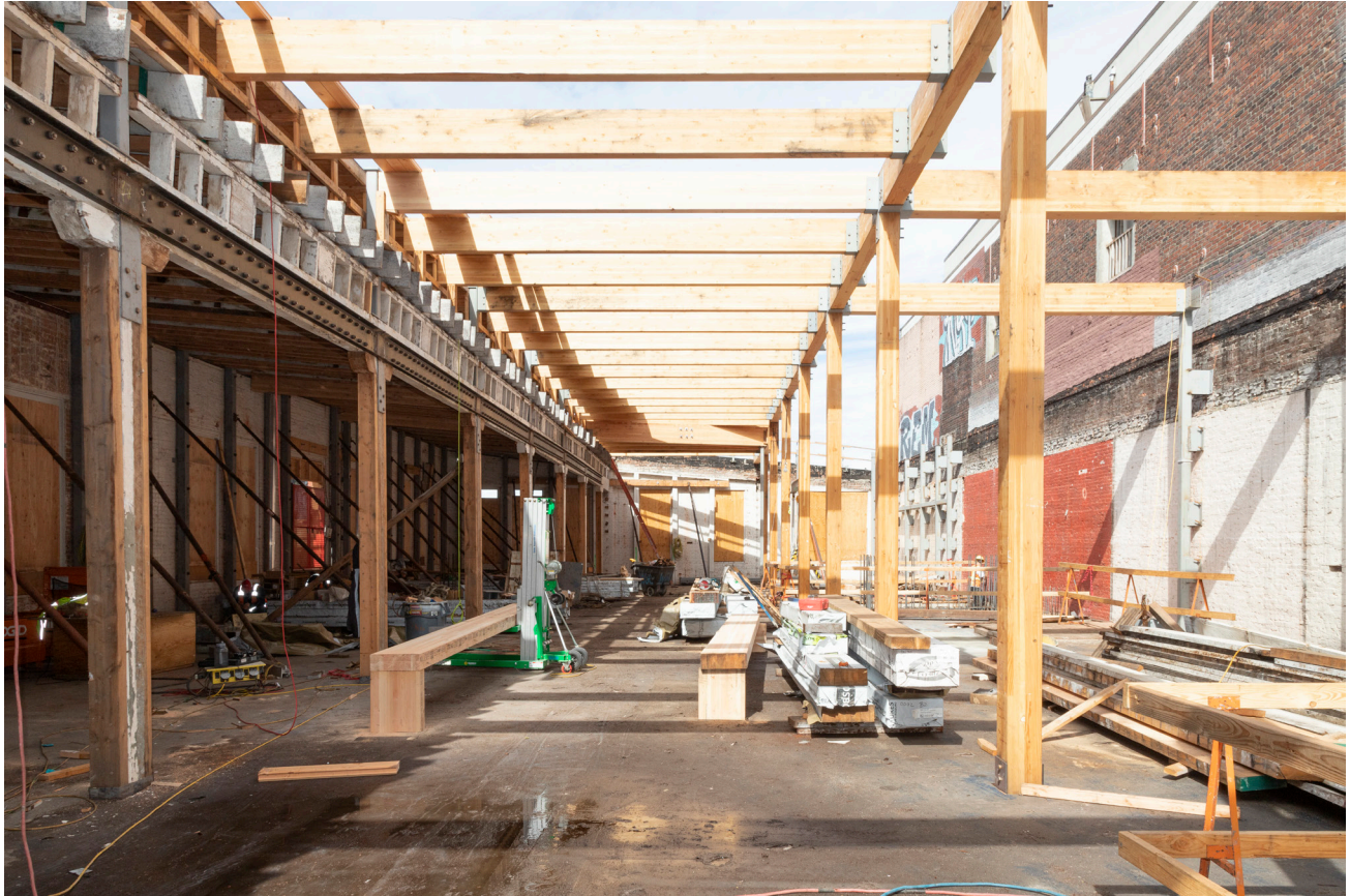
PHOTO 26. After: 2022 third floor, showing roof framing in progress.
