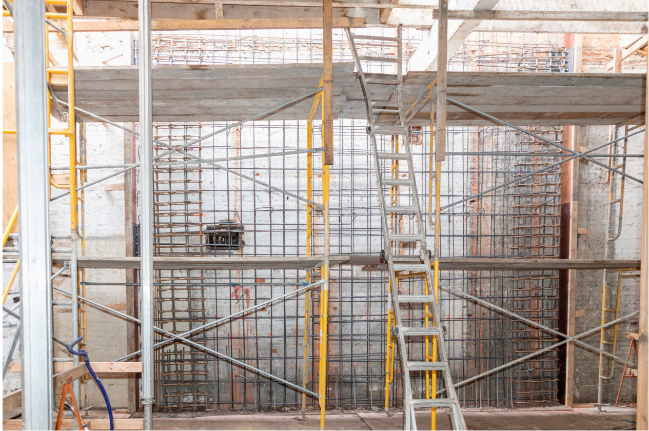
PHOTO 20. After: 2022 second floor, Shear Wall 1 steel placed.
