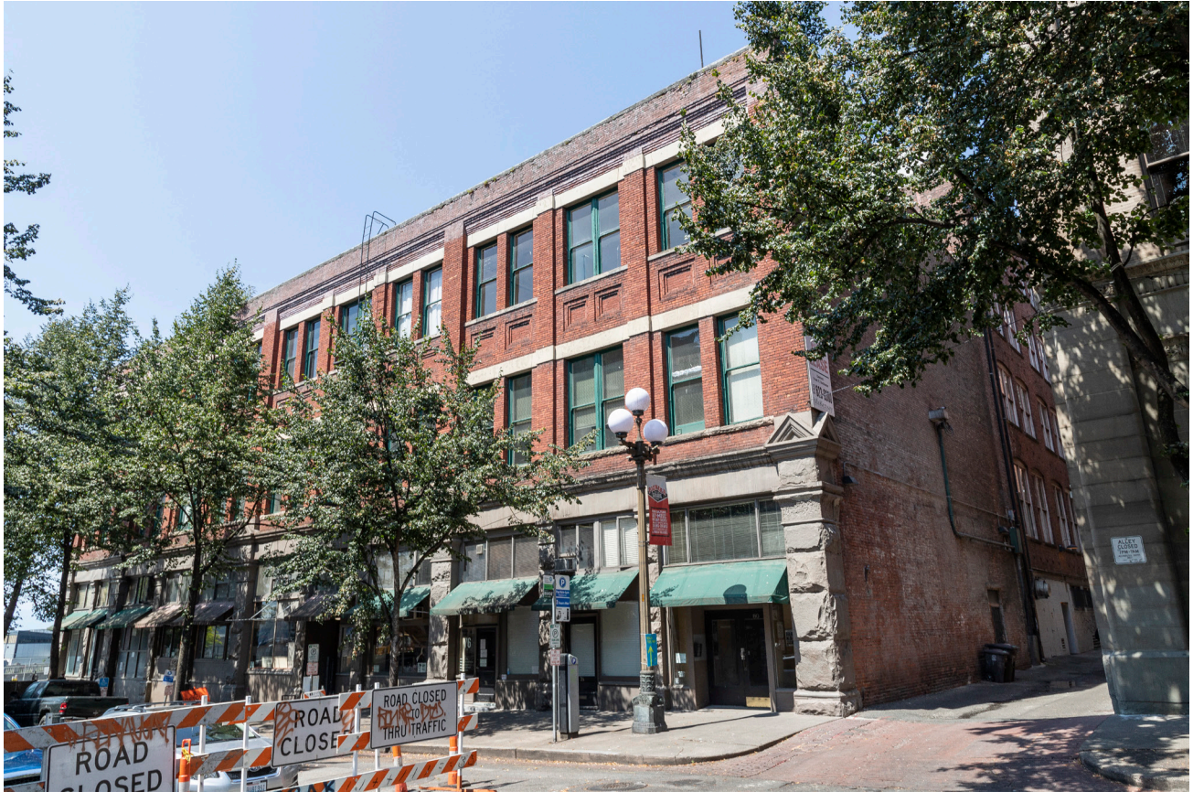
PHOTO 1. Before: 2020 site, southeast corner looking northwest across S Washington Street. Alley at right.
