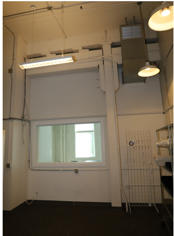
PHOTO 19. Before: 2020 Second floor, office space, looking south.
