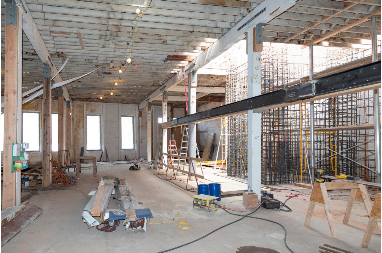
PHOTO 22. After: 2022 second floor, elevator core and Shear Walls 3-6 steel placed..
