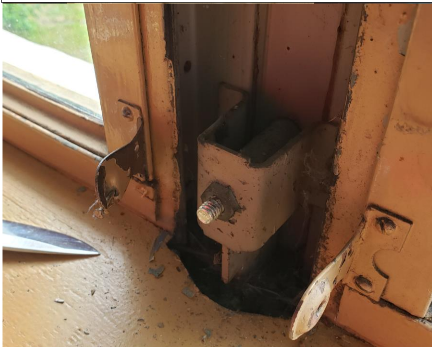
Photo-3 above depicts the concealed brackets used to connect the steel windows at the base of the existing jambs. Note: The brackets are secured to the building structure (embedded in concrete) at only the head and sill of the windows. Intermediate brackets between windows are also located every 16-to-20-inches running vertically between the windows.
