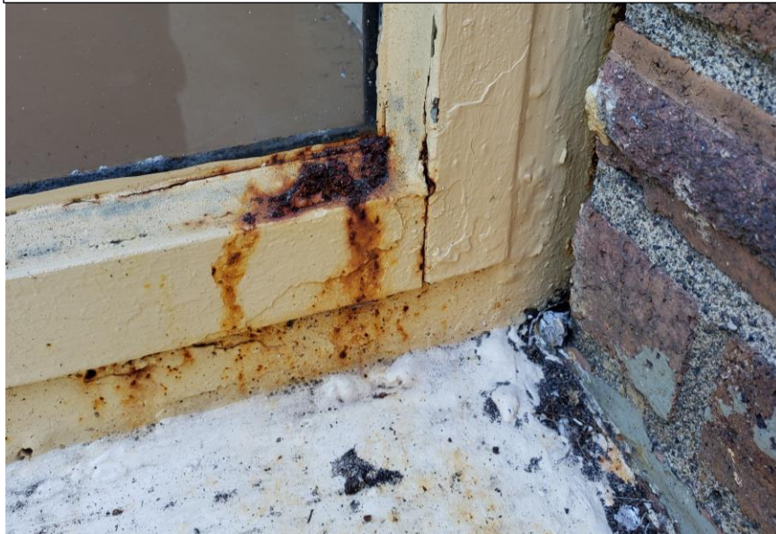
Photo-11 below depicts a close up view of the corrosion found at the lower corners of in-swing hopper windows.
