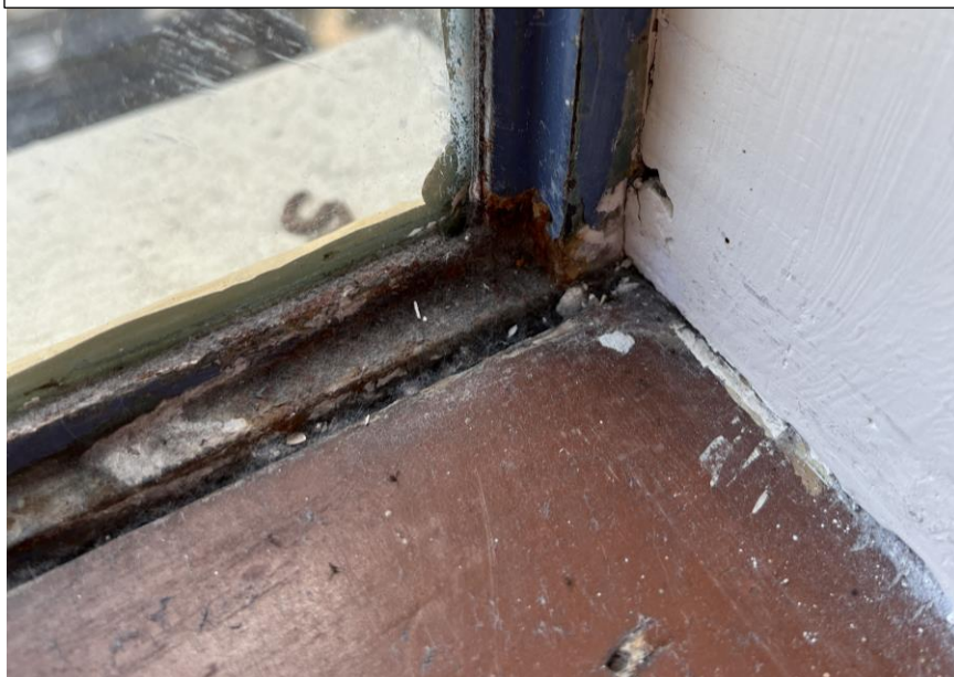
Photo-12 below depicts corrosion on the interior side of a fixed window.
