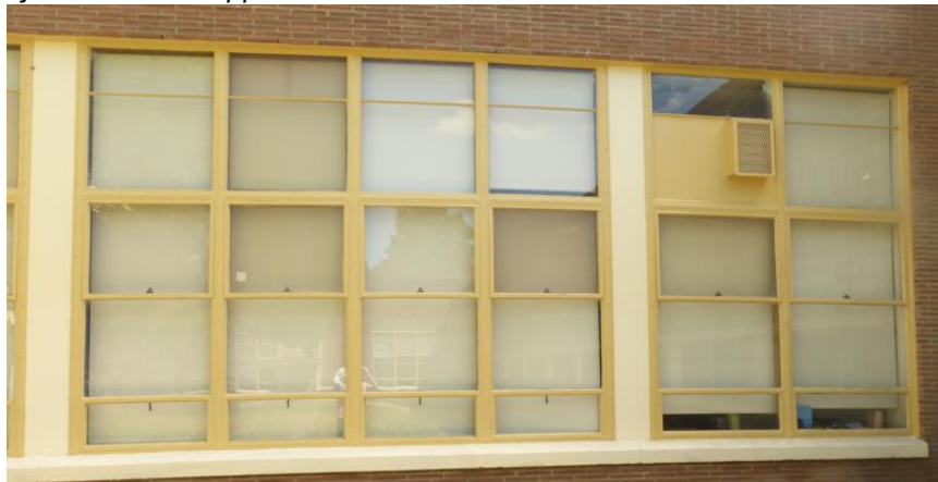
Photo-13 above depicts three distinct glazing colors over a series of adjacent windows as well as an example of a glazing panel that was infilled for an exhaust vent.
