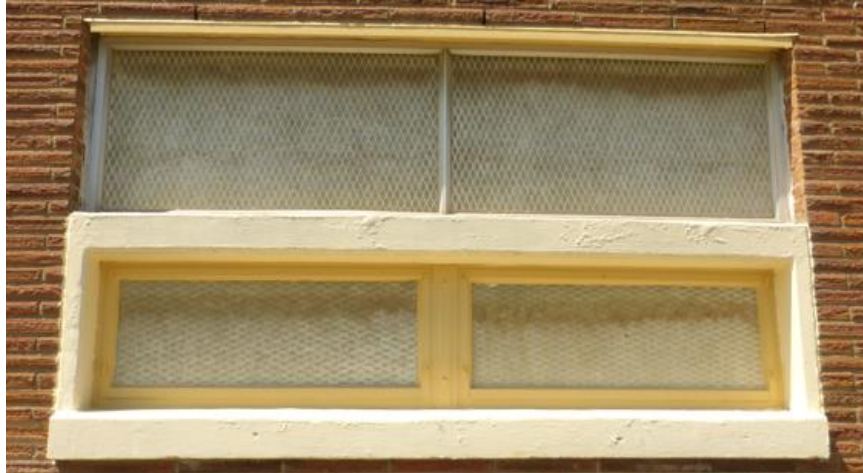
Photo-14 above depicts window glazing that has been replaced with fiberglass/expanded steel mesh panels.
