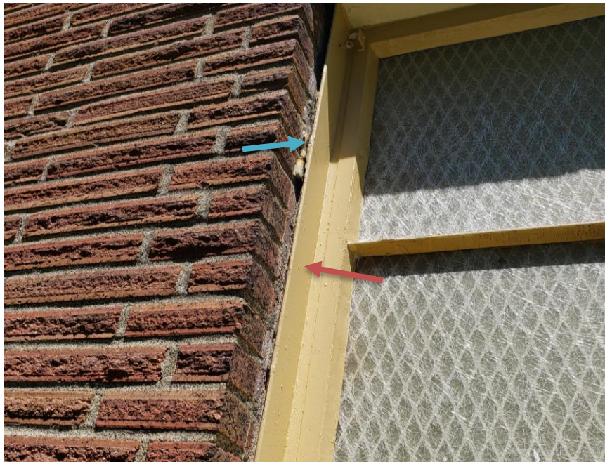
Photo-4, Red arrow above points to a painted steel plate used to secure the flange at the jamb of an original window. Blue arrow points to asbestos containing sealant. This photo also shows an example of how the original glazing has been replaced in many locations with reinforced fiberglass panels
