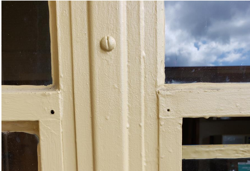
Photo-2 above is an up close view at the intersection between lower operable awnings and the fixed portion of the window.
