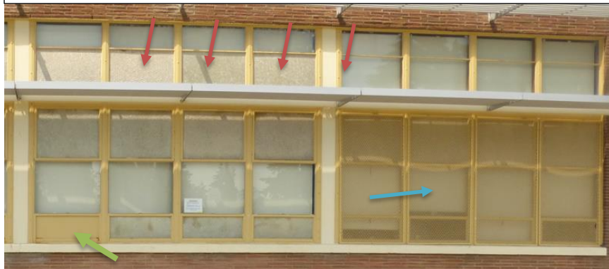
Photo-15 above depicts window glazing that has been replaced with fiberglass/expanded steel mesh panels (red arrow), where the glazing of a lower in-swing hopper has been replaced with a painted sheet metal panel (green arrow), and where a painted steel screen is installed over a section of windows (blue arrow).
