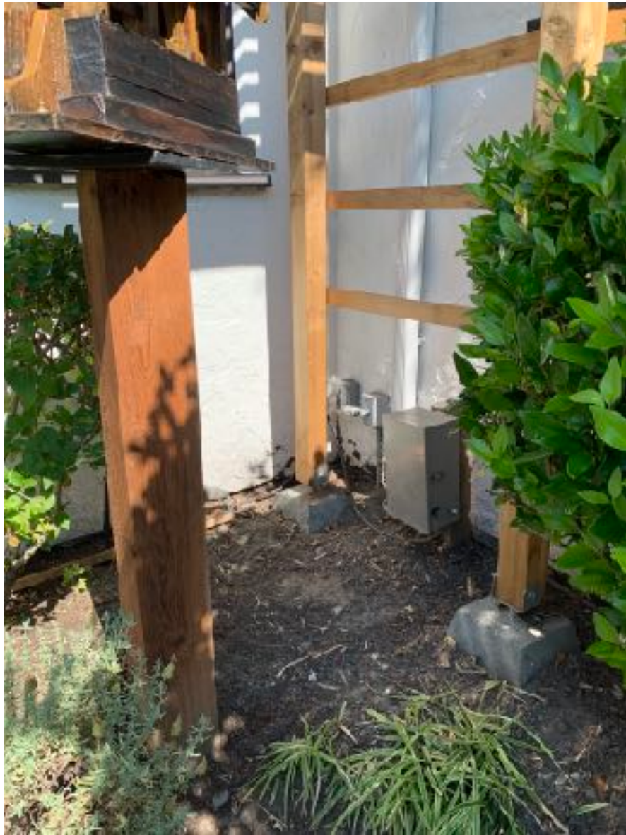
Posts bolted to 8" x 8" x 8" Piers for stability in wind
