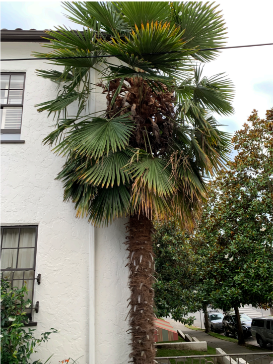
Top of tree against building and through power line
