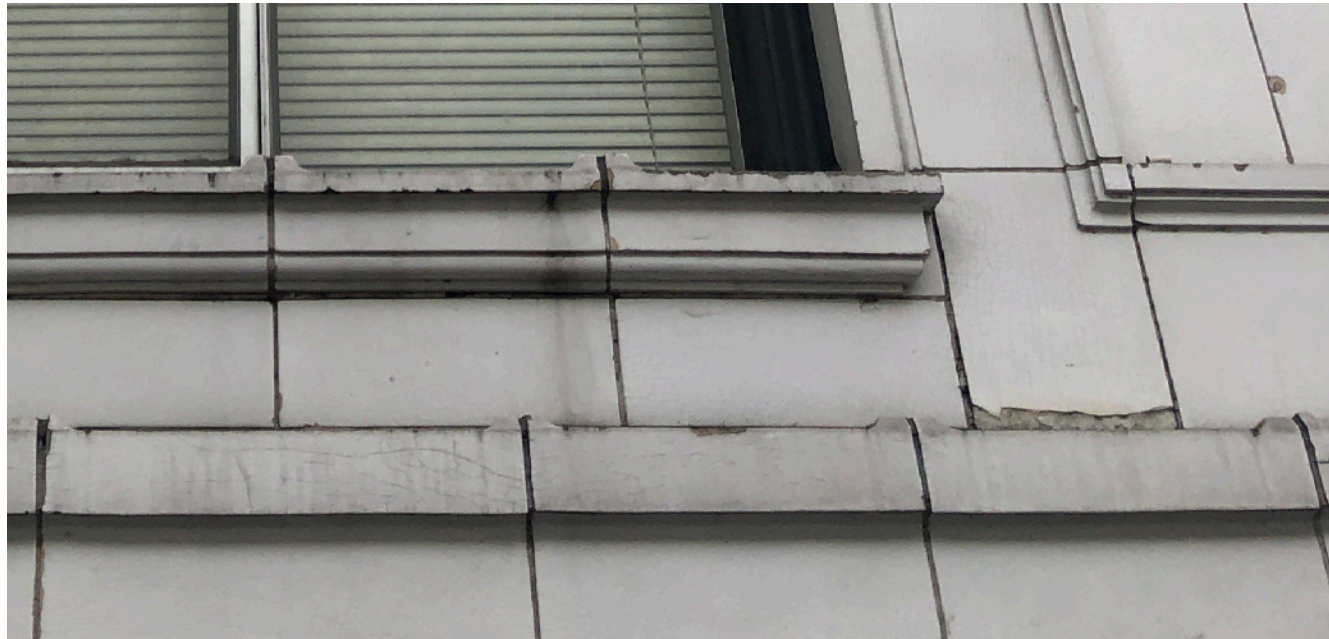
Replace Spalling Terracotta
