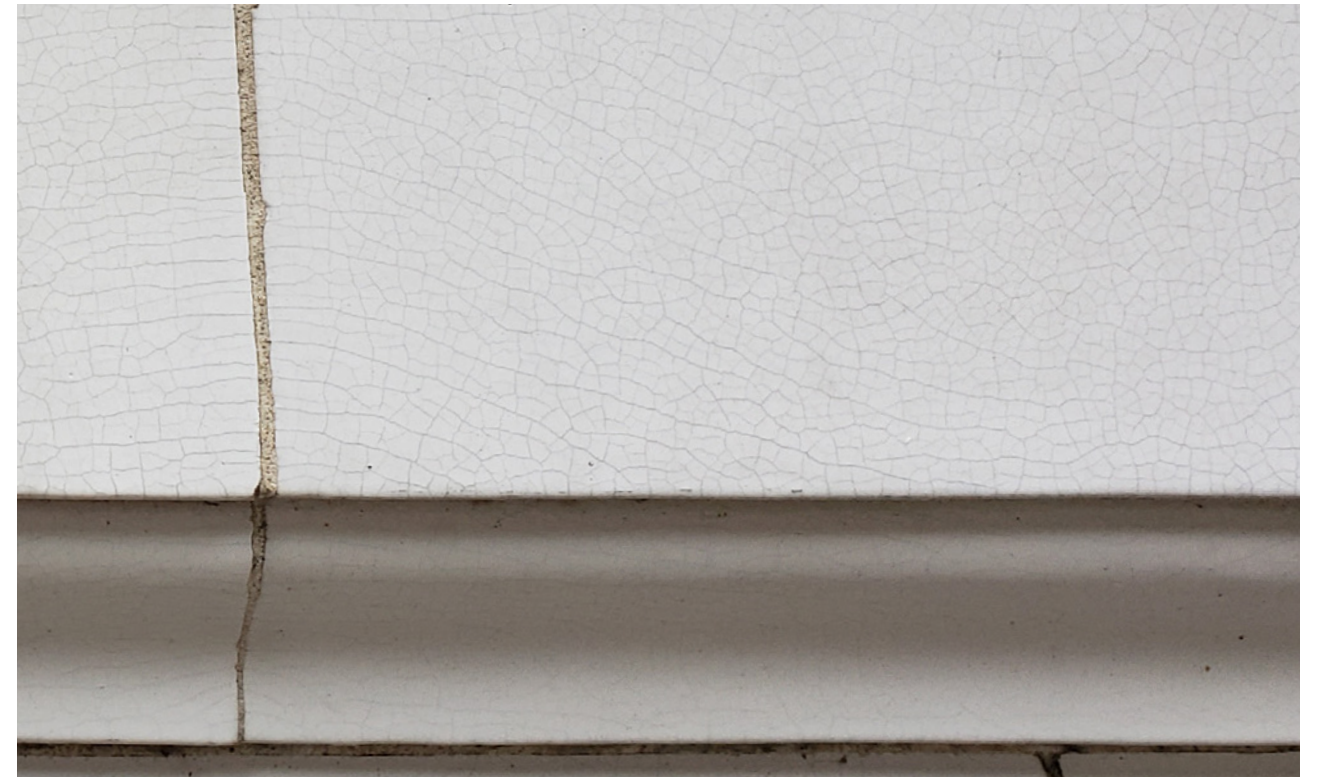
Spiderwebbing: Reglaze to Seal
