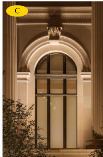
Canopy mounted linear uplight to highlight arch
