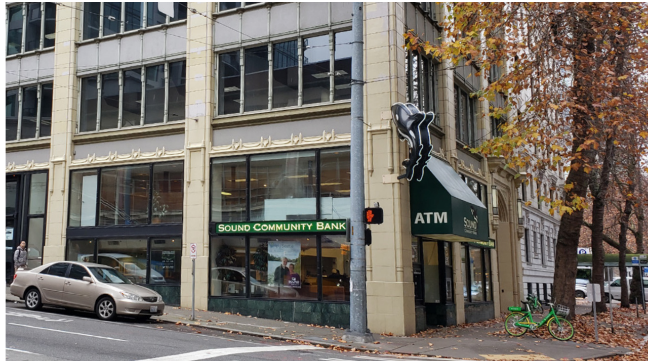
Remove Modern Signage & Canopies
