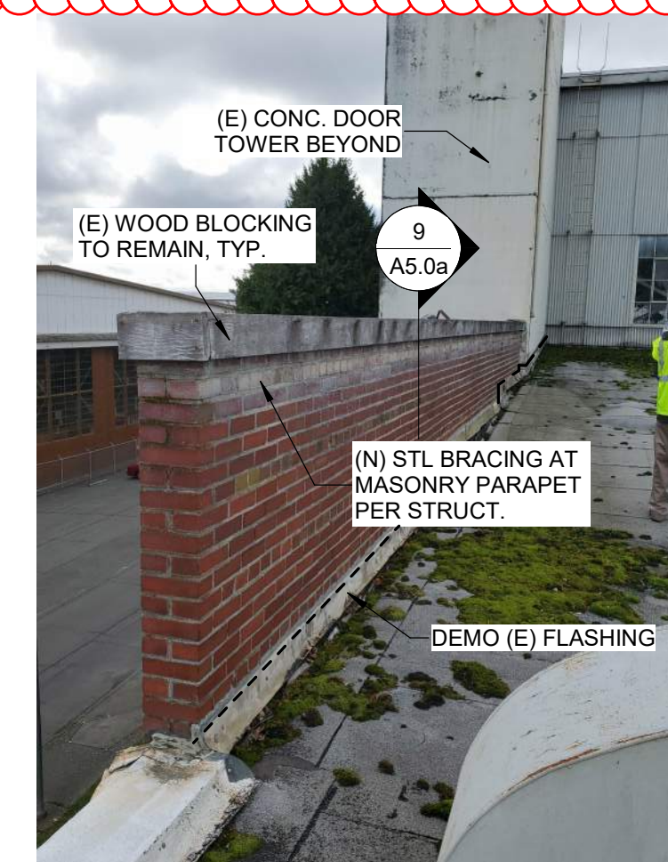
13 URM AT PARAPET D5.0a NTS
