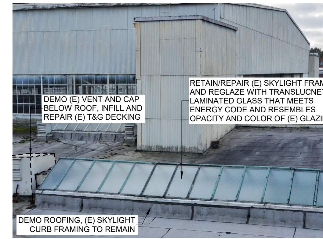
7 EAST AT DOOR TOWER D5.0a NTS
