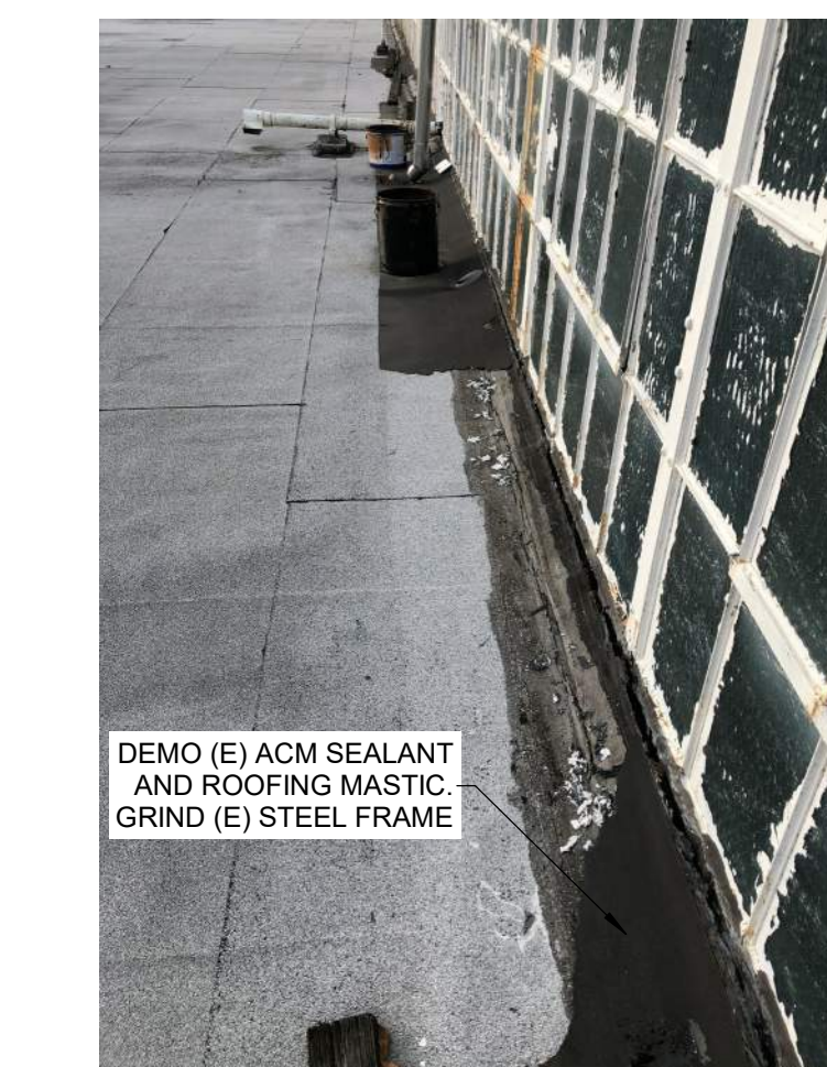
24 BASE AT N. CSTRY D5.0a NTS
