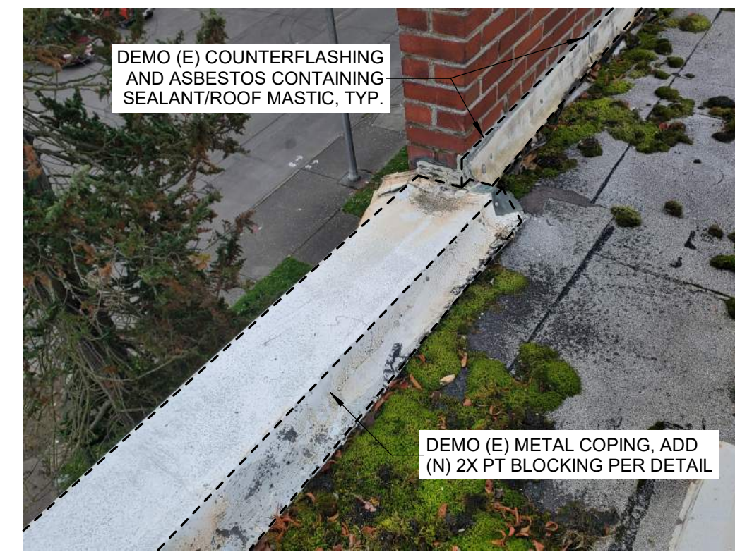
3 STEP AT EAST PARAPET D5.0a NTS
