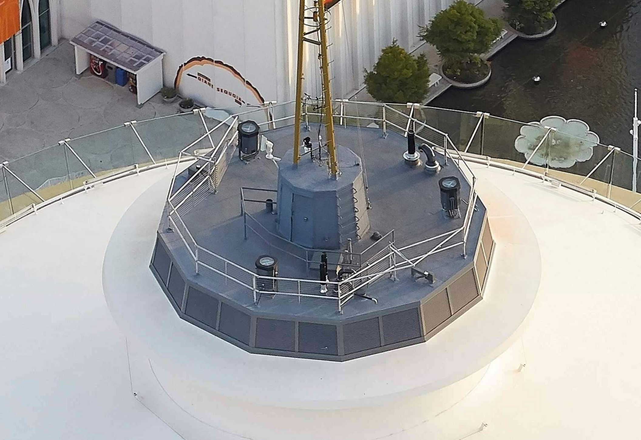
Existing roof equipment
