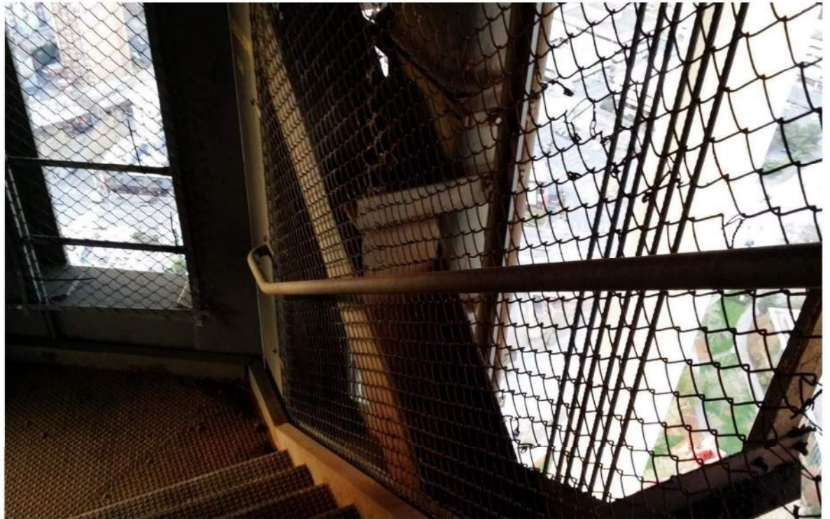
Existing stair chainlink enclosure
