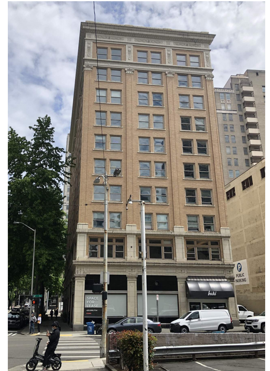
6th Ave facade of the Lloyd Building with non-historic storefronts
