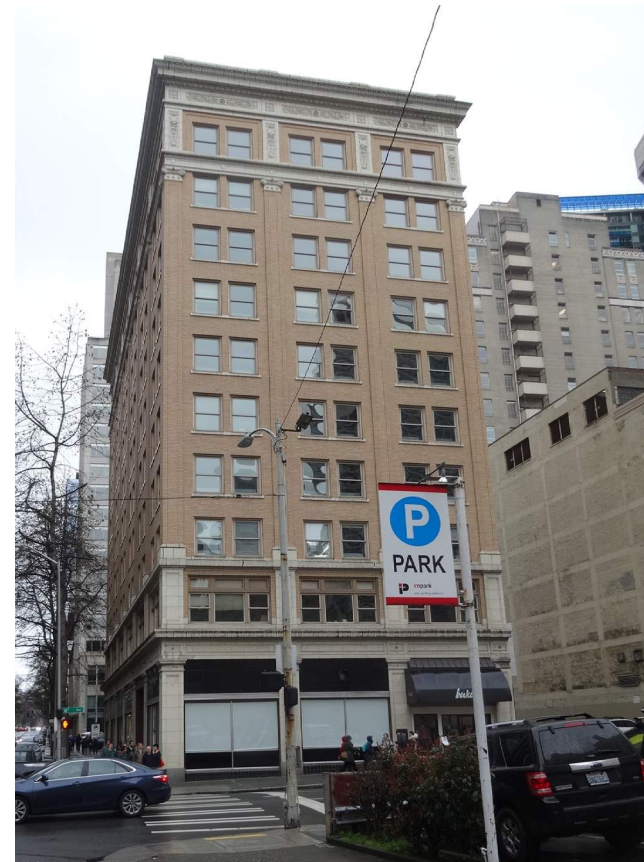
6th Ave. Facade
