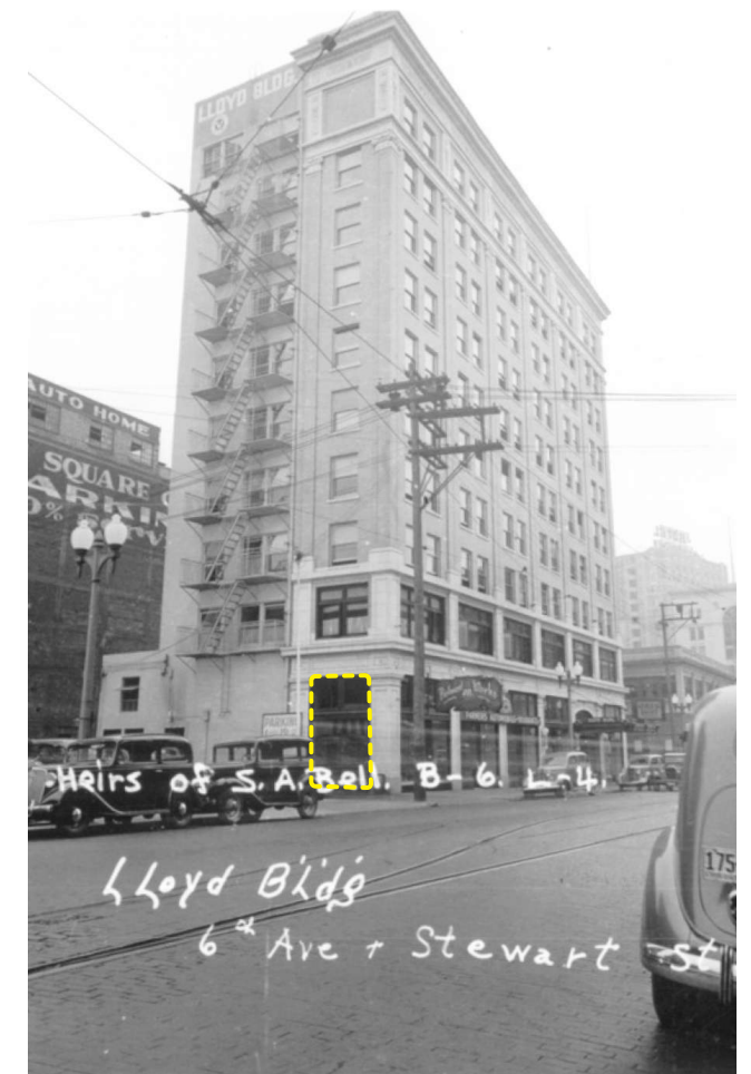
The Lloyd Building in 1937. The original storefront design is partially visible.
