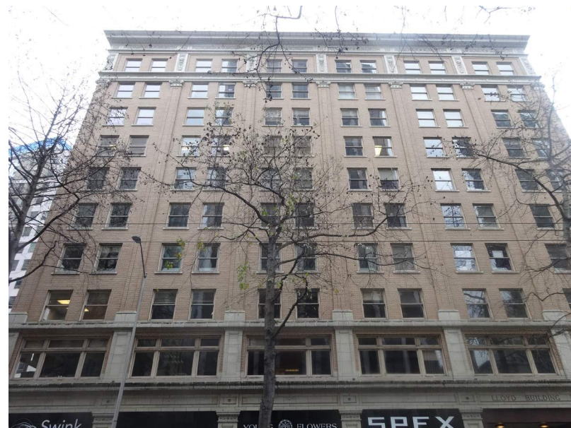
Stewart St. Facade
