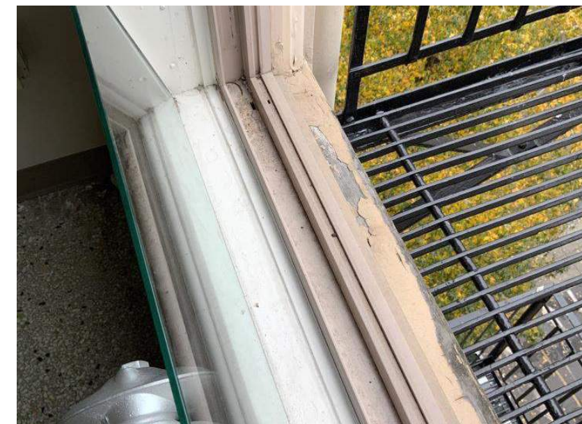
Typical existing non-original vinyl insert window
