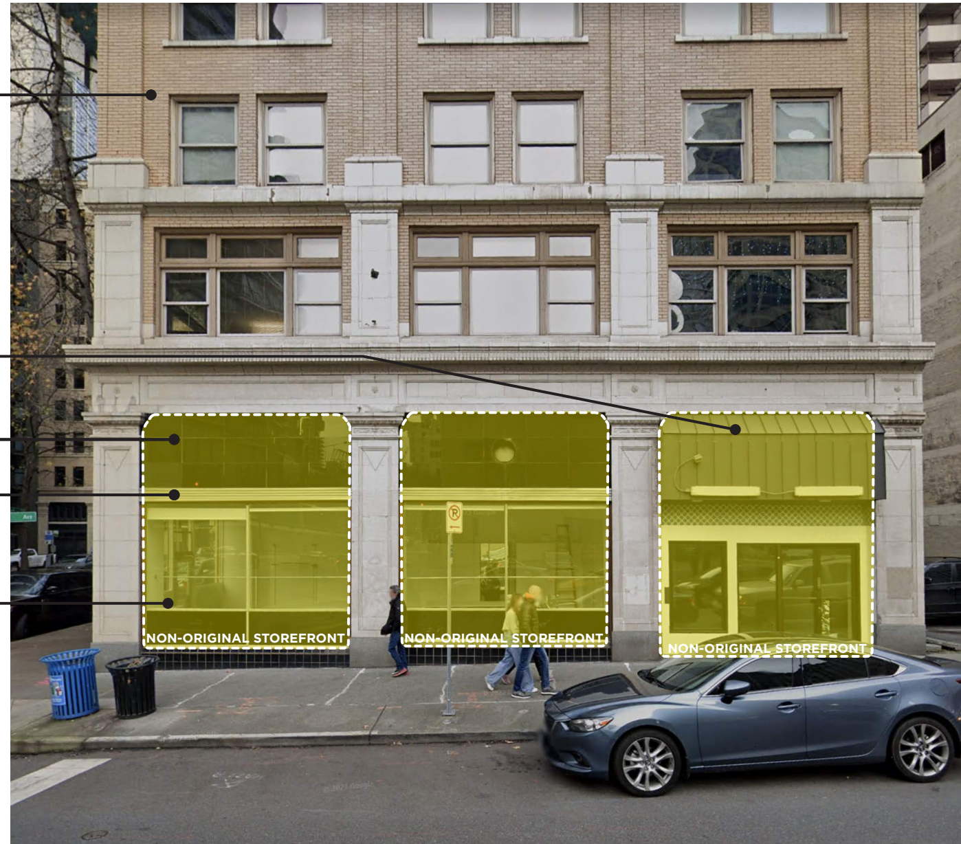
Existing non-original storefront along 6th Ave
