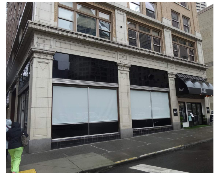
Ground level retail on 6th Ave.
