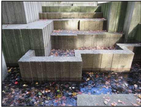
Rough, board-formed concrete
