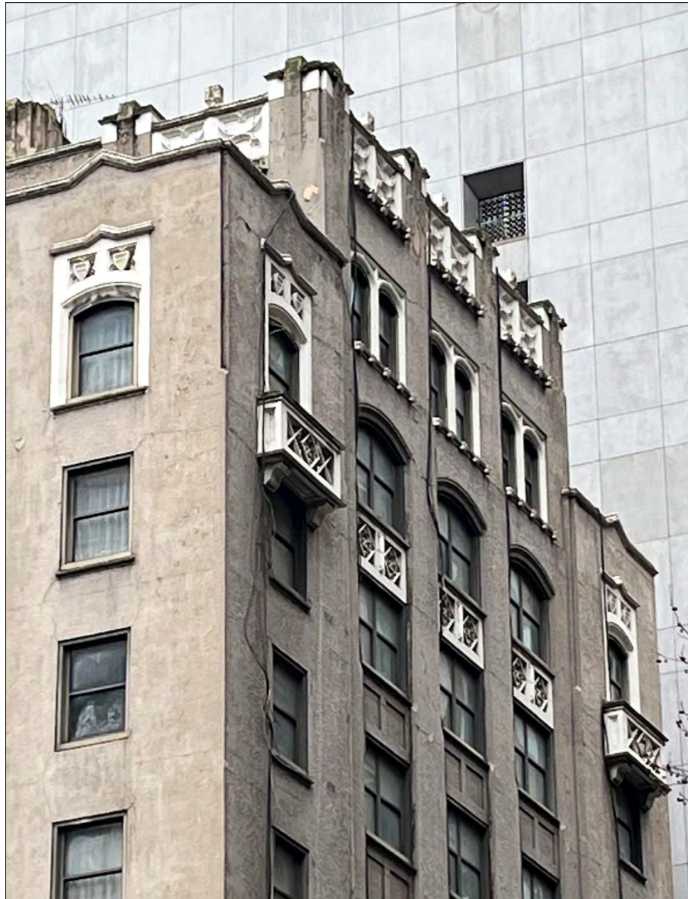
Current Photos: Terra Cotta & Stone Cladding
