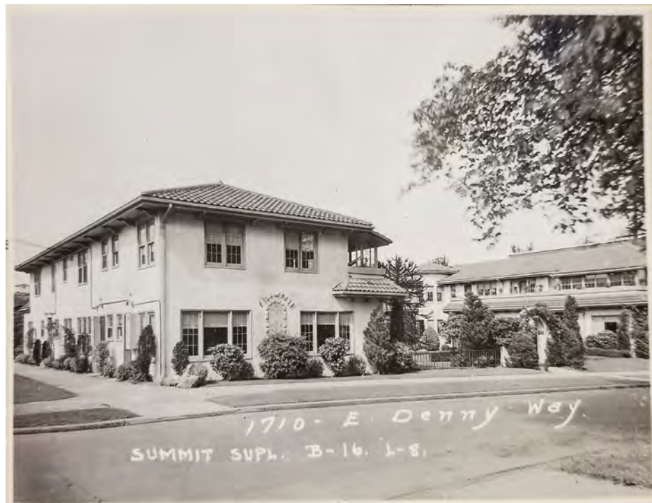
Figure 111. Ca. 1937 view, southwest corner. Source: Puget Sound Regional Archives, property record card.
