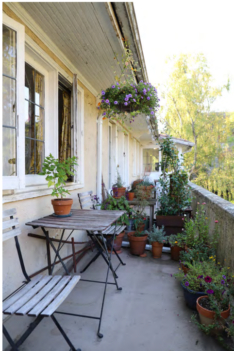
Figure 57. Second floor balcony, looking south.
