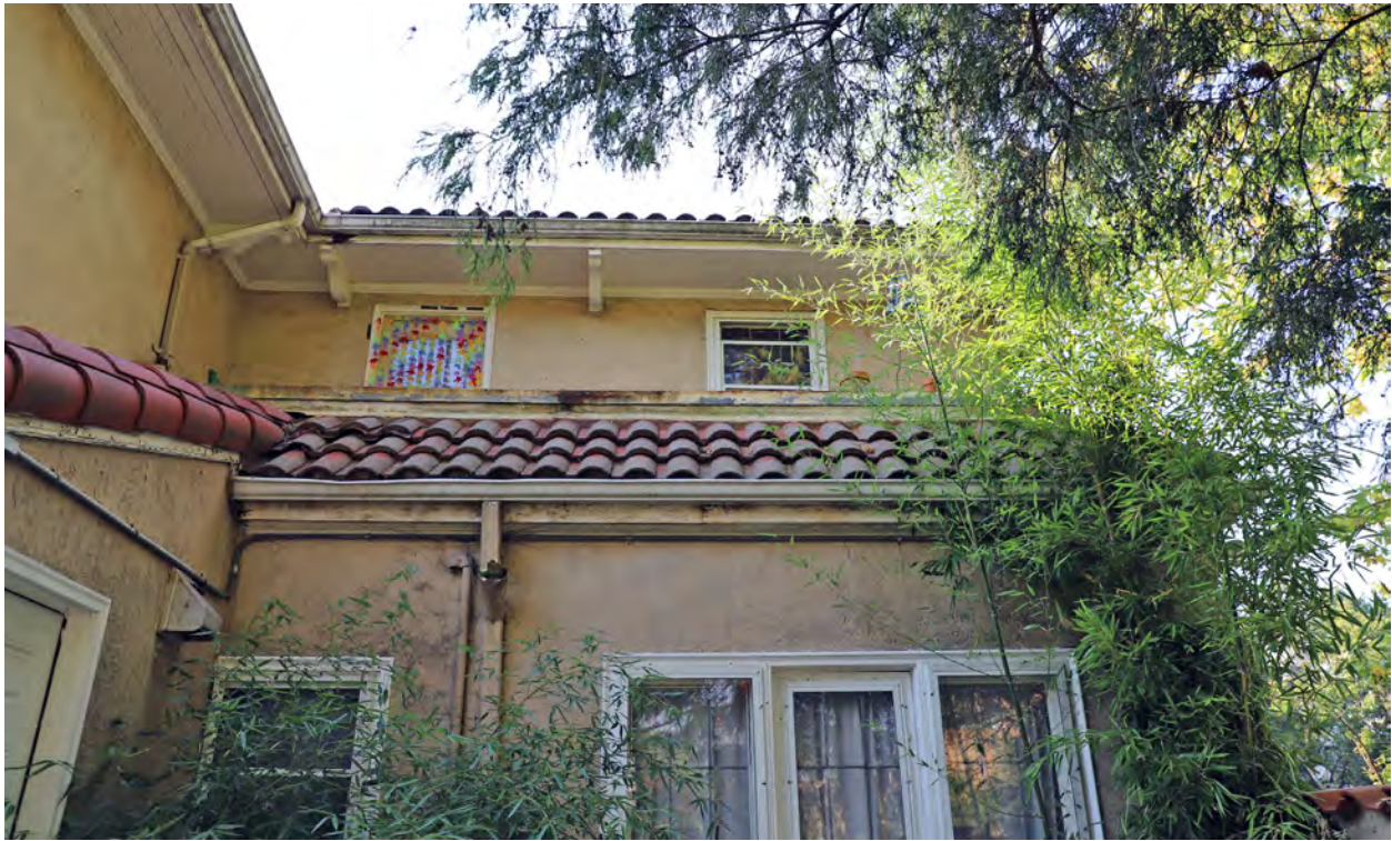
Figure 34. Balcony, northwest corner, looking south.
