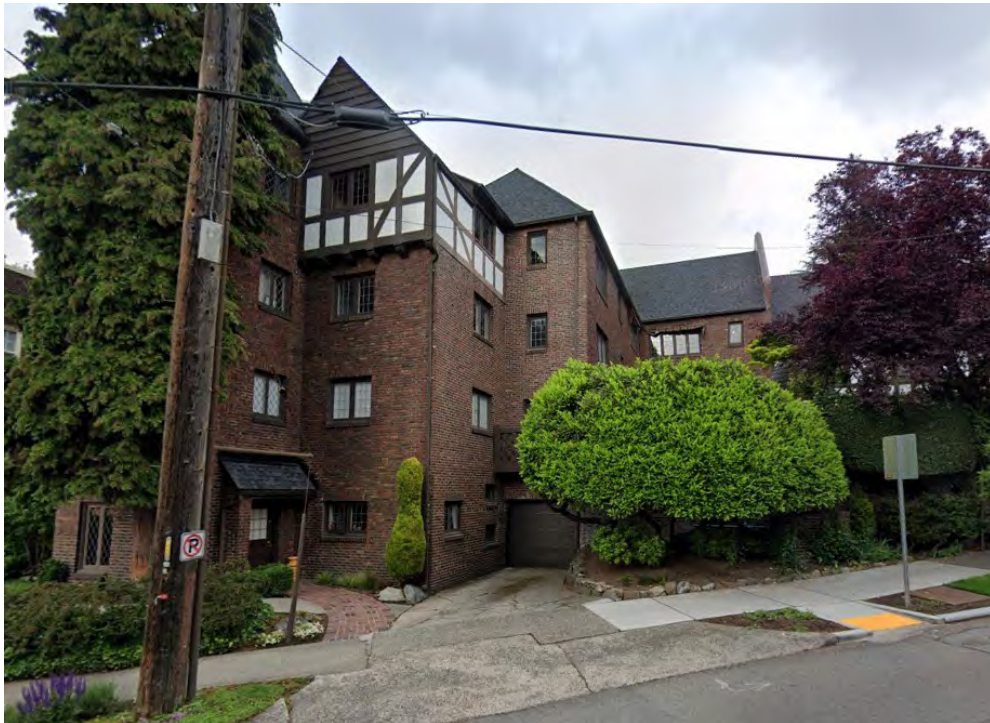
Figure 145. 750 Belmont Ave E, (built by Anhalt) and contributing to the Harvard-Belmont Landmark District. Source Google Street View.
