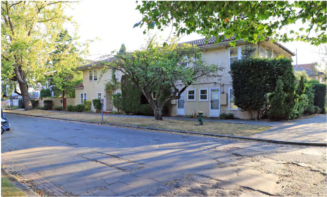
Figure 16. Exterior, west facade, looking northeast.
