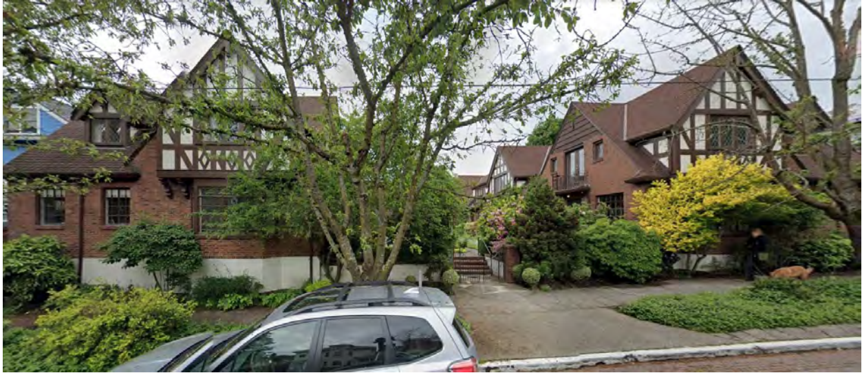
Figure 141. 111 14th Avenue E, (built by Anhalt). Source Google Street View.
