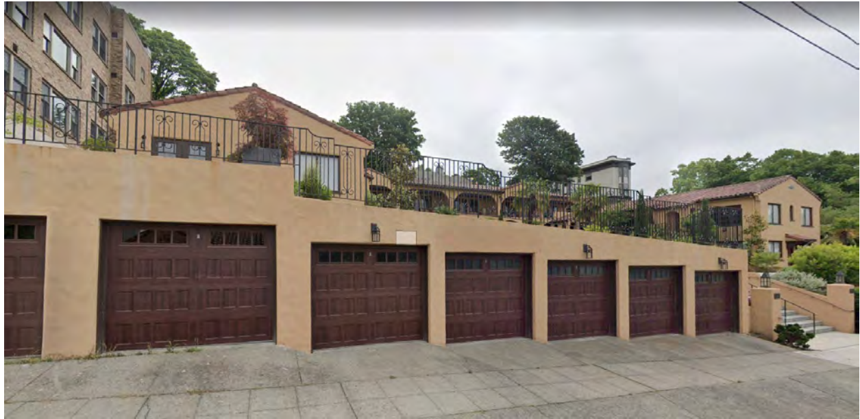
Figure 122. 1108 9th Avenue W, northwest corner along Ninth Avenue W. Source: Google Street View.
