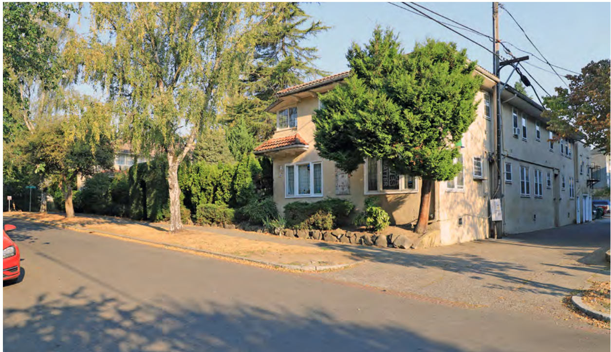
Figure 21. Exterior, southeast corner.
