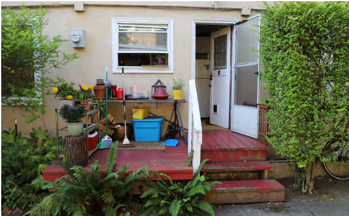
Figure 84. Backyard entrance crossing the basement stairwell. Wood deck at left is built out over the stairwell.
