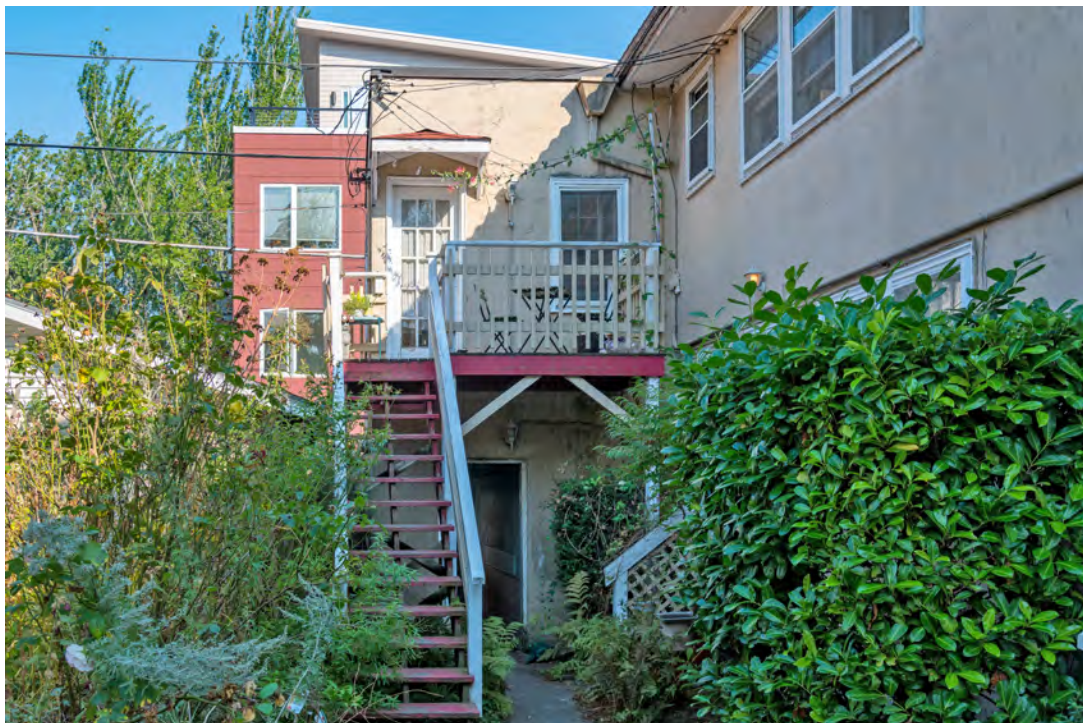
Figure 78. Studio apartment entrance. The deck is pressure treated wood. Photographer: Jesse L. Young, Seattle.
