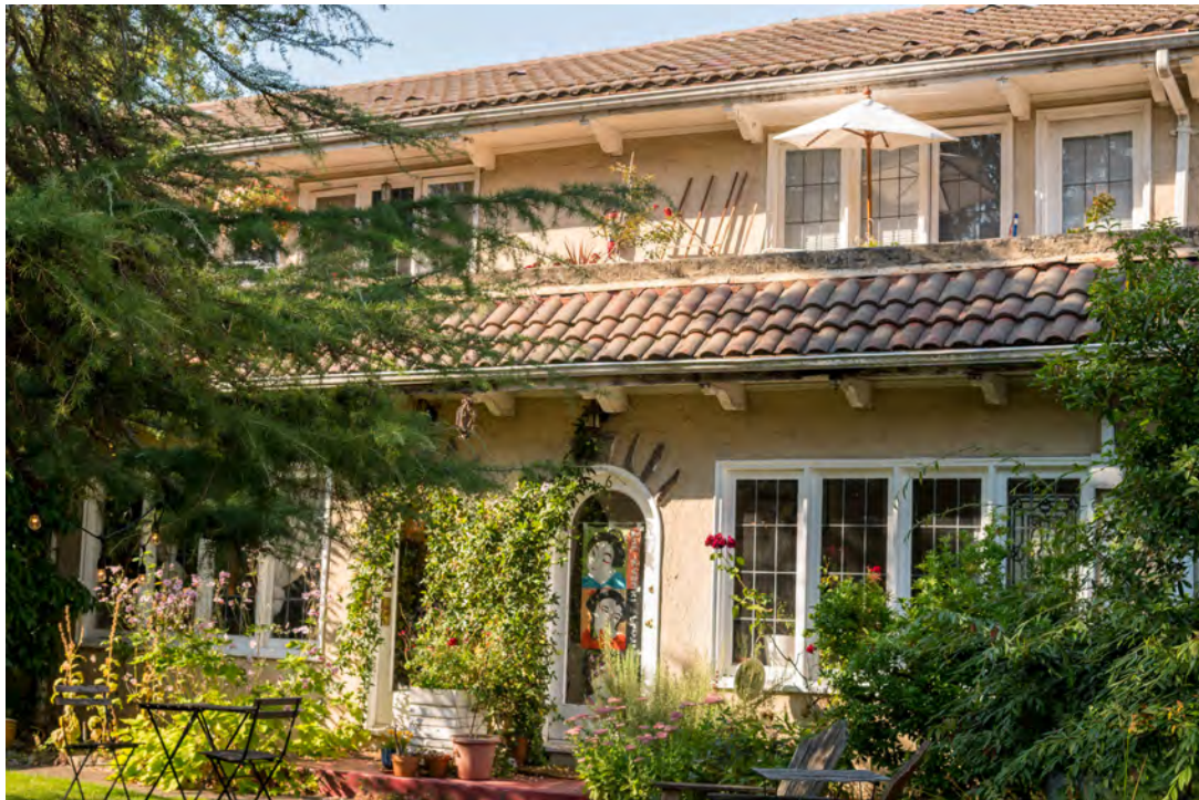
Figure 35. Roof, looking north. Photographer: Jesse L. Young, Seattle.
