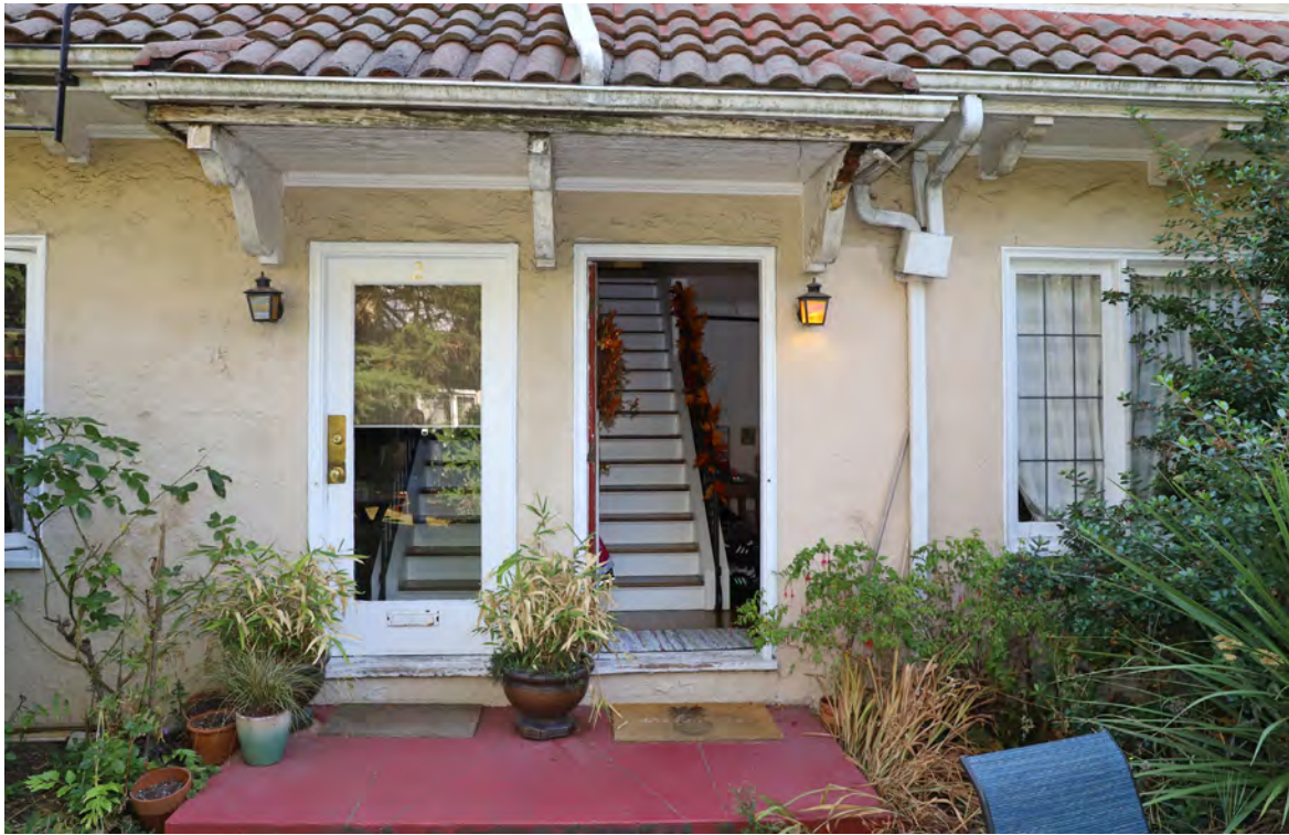
Figure 90. Courtyard entrance for units at south end of east wing.
