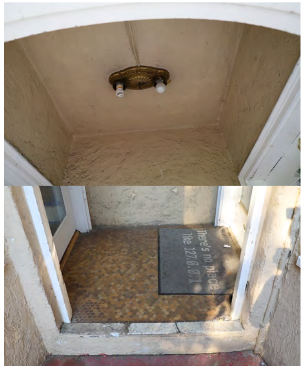
Figure 81. Vestibule detail, showing tile floor and ceiling.
