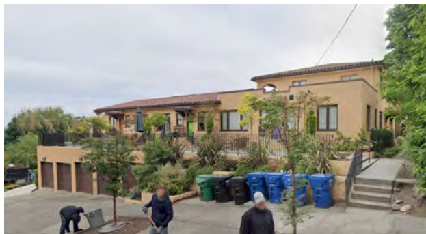
Figure 123. 1108 9th Avenue W, southeast corner along W Prospect Street. Source: Google Street View.
