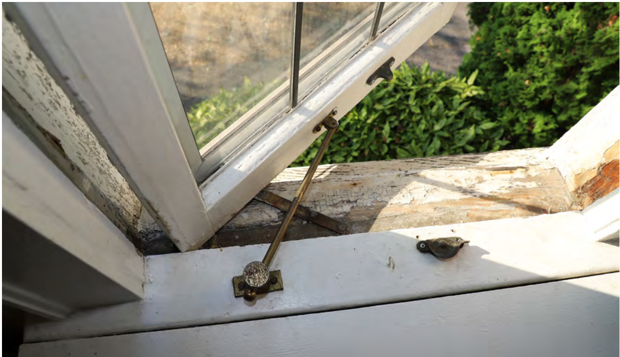
Figure 39. Window, sash stay and lock detail.
