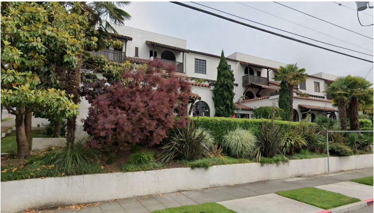
Figure 128. 348 W Olympic Place, Villa Costella (condominiums, Seattle Landmark) built ca. 1929 south facade. Source Google Street View.
