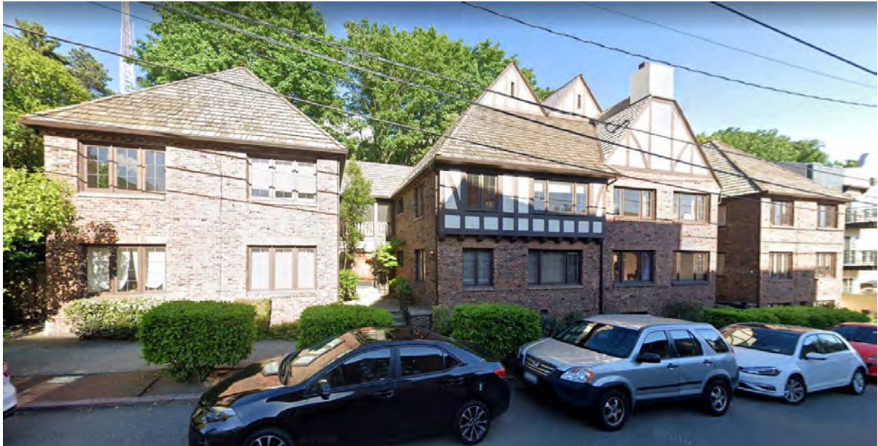
Figure 149. 1320 Queen Anne Avenue N, (built by Anhalt). Source Google Street View.
