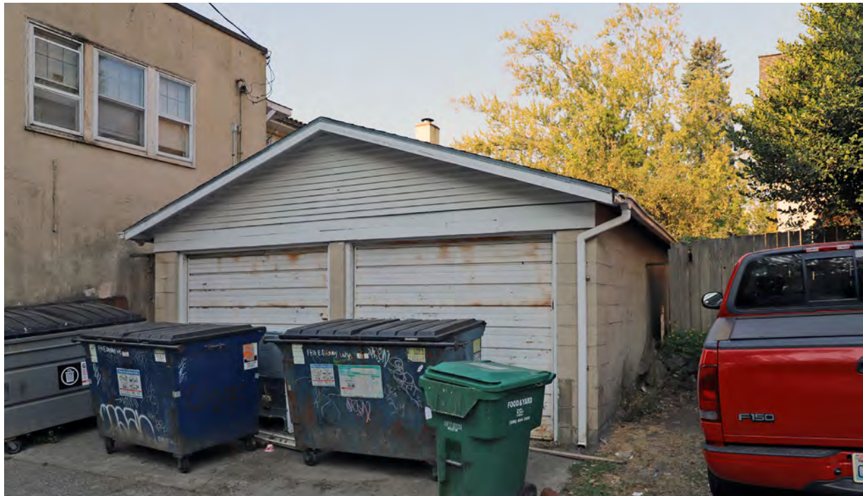
Figure 23. 1950 detached garage, northeast corner.
