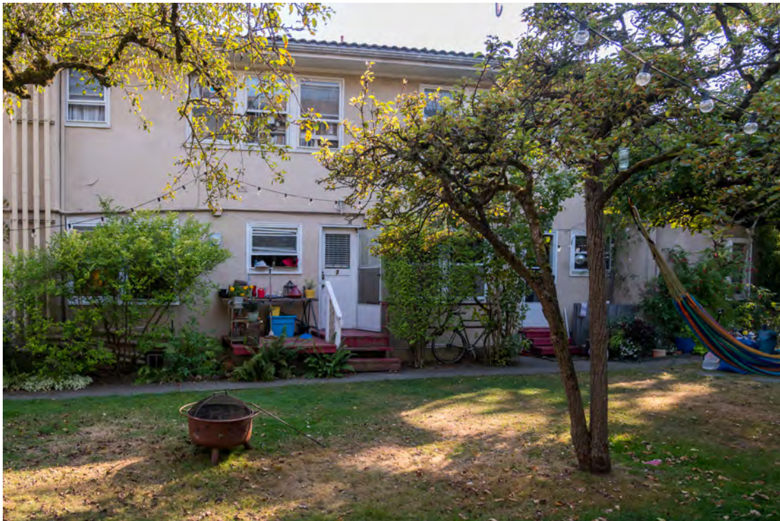
Figure 18. Exterior, north facade, east portion. Photographer: Jesse L. Young, Seattle.
