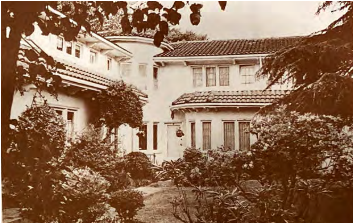
Figure 113. Undated (ca. 1978 based on the book's first publishing date) view of the courtyard at the La Quinta Apartments Source: Larry Kreisman, 1982, Apartments by Anhalt , (Seattle: Kreisman Exhibit Design), 25.
