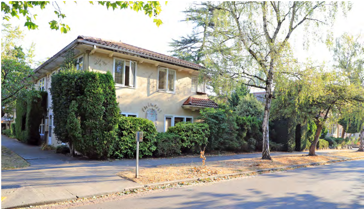
Figure 15. Exterior, southwest corner.
