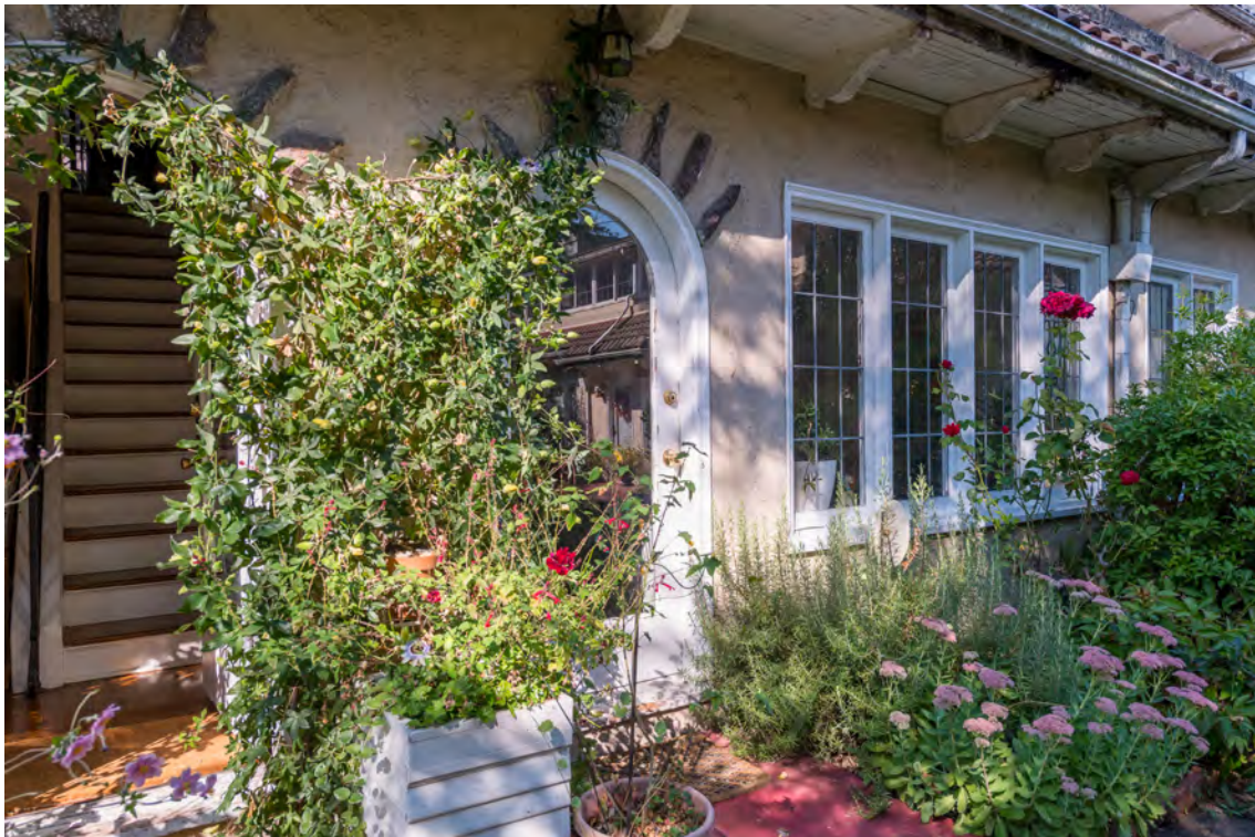
Figure 42. North unit entrance. Photographer: Jesse L. Young, Seattle.
