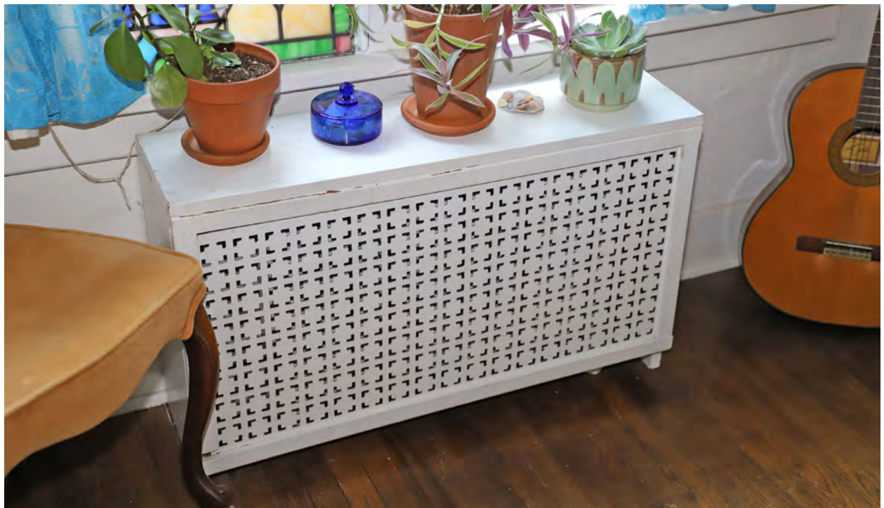
Figure 60. Radiator cabinet, typical of other units.
