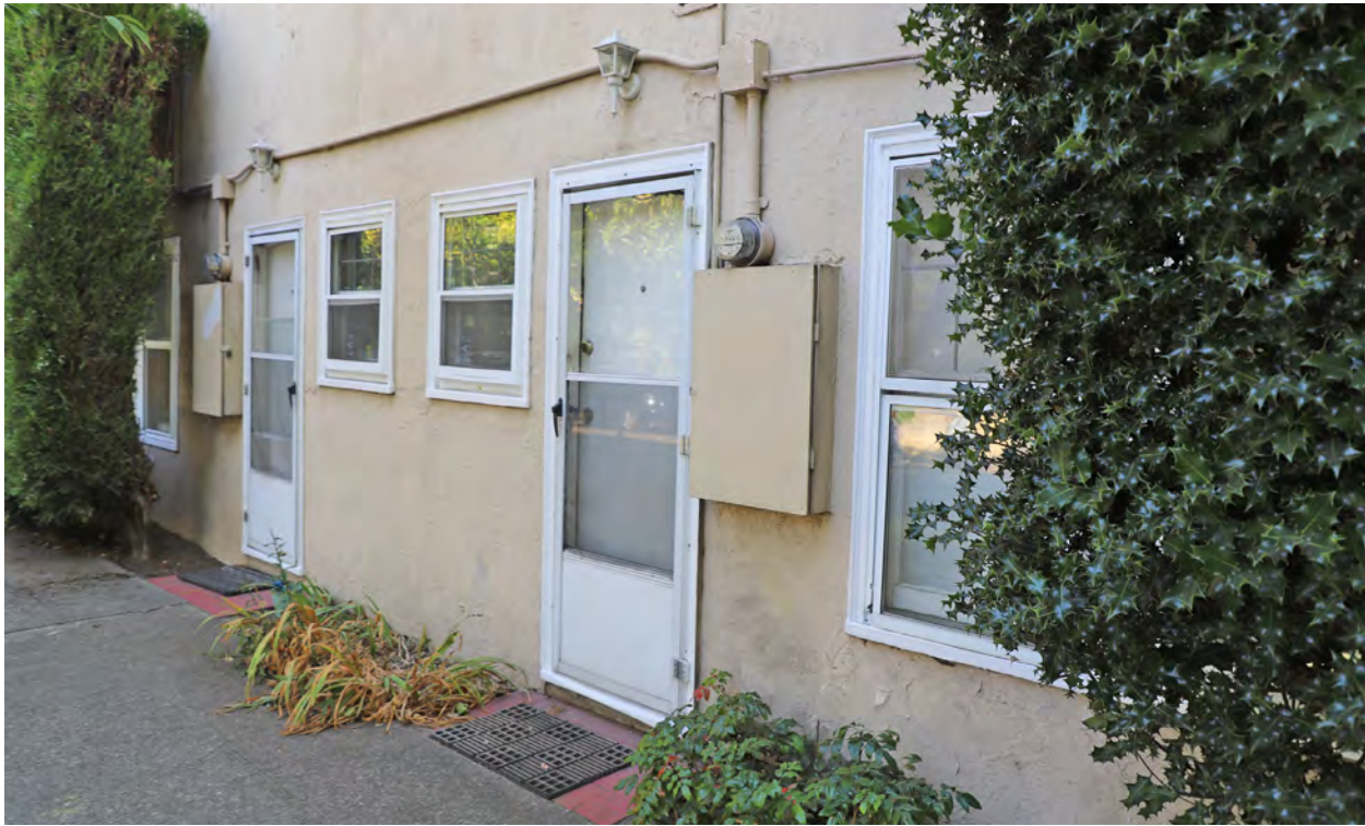
Figure 86. 17th Avenue E entrances, looking northeast.
