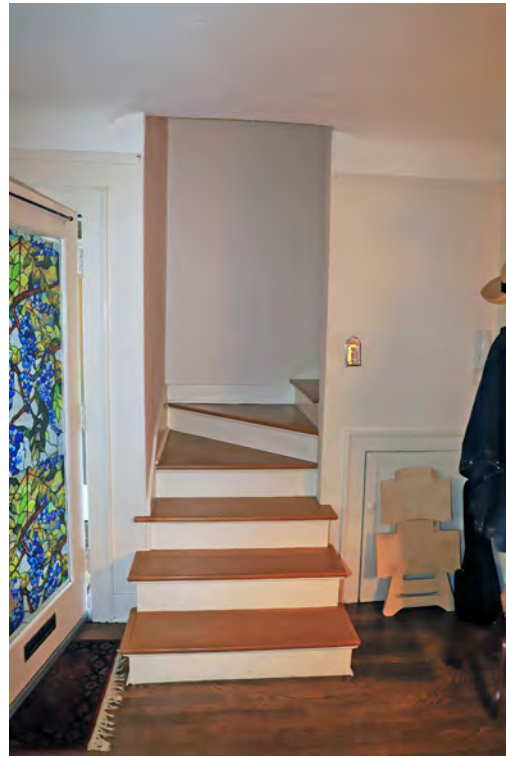
Figure 54. Stairway to second floor.
