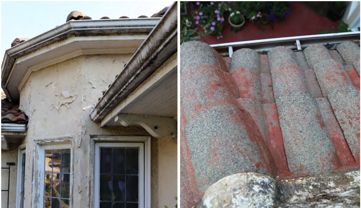
Figure 37. Roof details. Tower and boxed eaves (above left) and concrete tiles painted red with flat valleys (above right).
