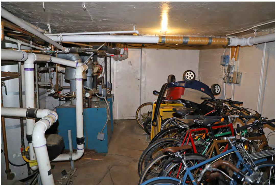
Figure 76. Basement, looking east.
