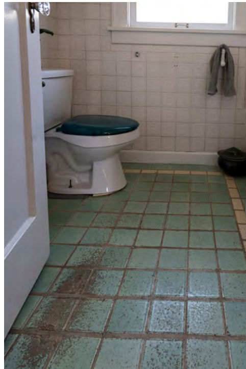
Figure 47. Second floor bathroom. Photographer: Jesse L. Young, Seattle.
