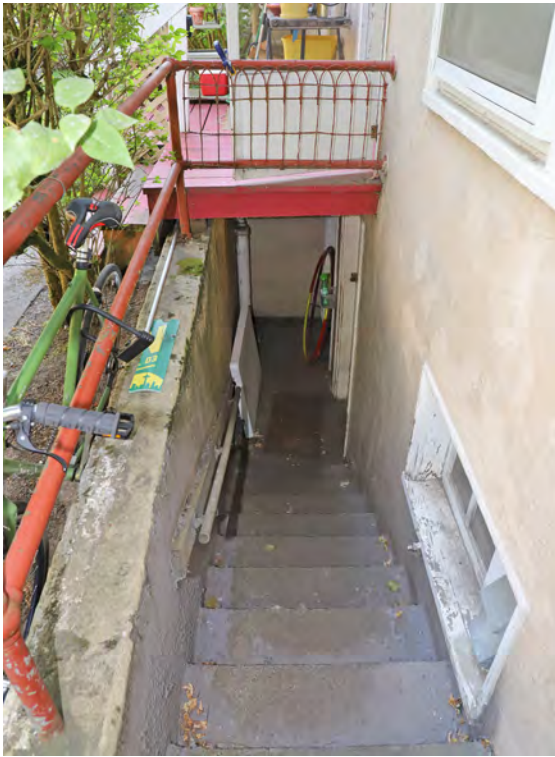
Figure 83. Basement entrance, looking east.
