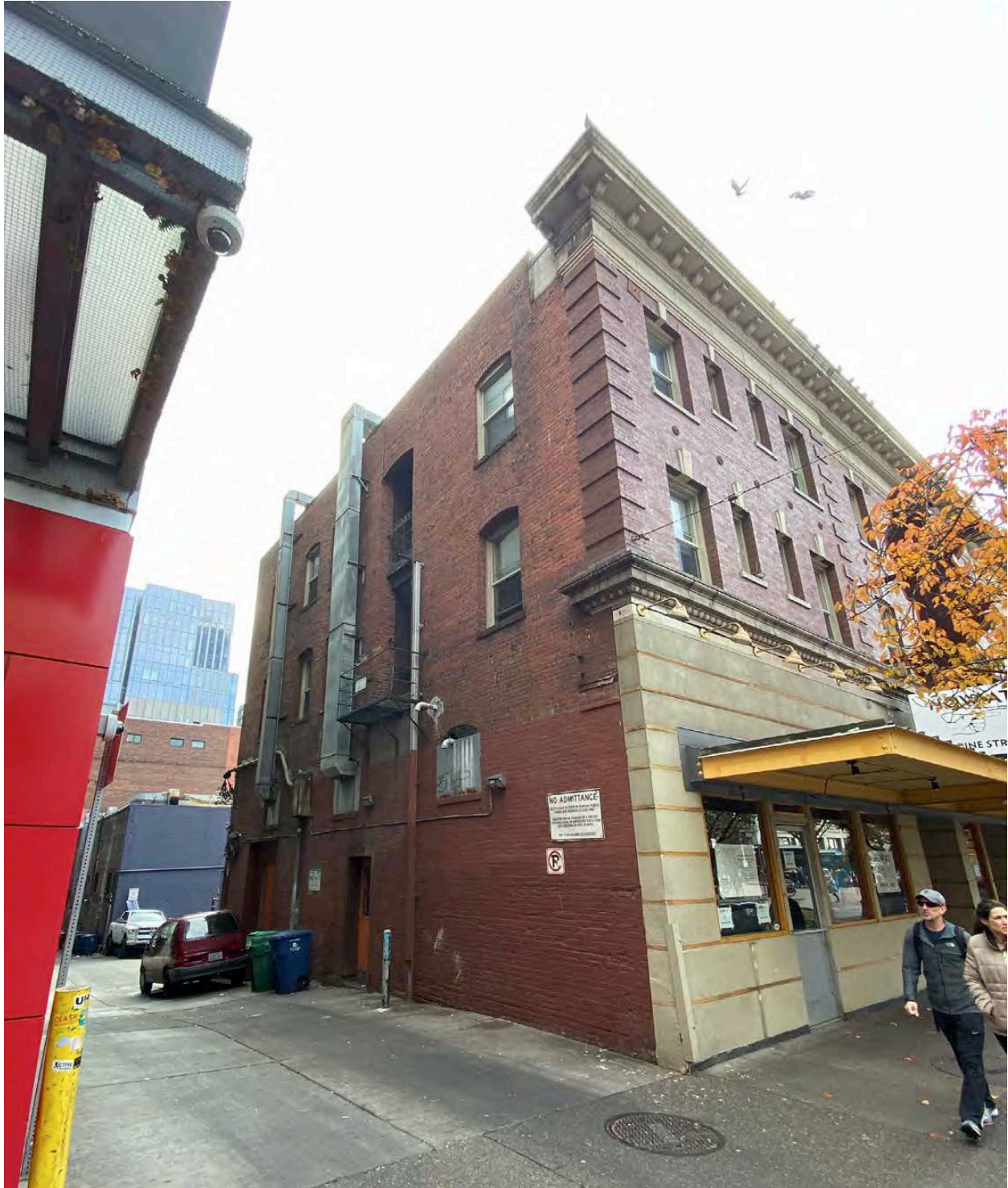
Figure 33: Eastern alley facade, showing EIFS detailing at cornice and storefront.
