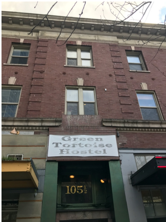
Figure 32: Entrance to Green Tortoise Hostel from Pike Street showing missing pedimented arch from original structure.
