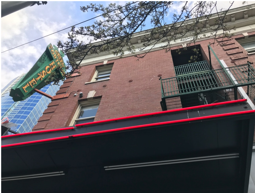
Figure 27: Detail of EIFS cornice at west facade.
