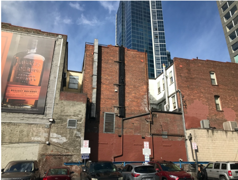
Figure 26: South facade at parking lot.
