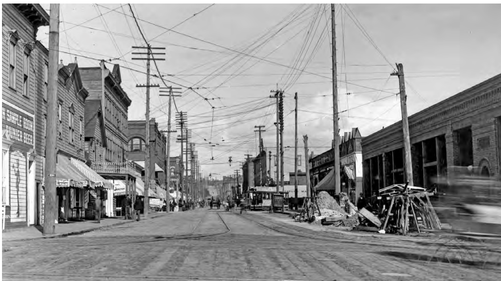
Figure 6: Original Hahn building under construction, c.1897.
