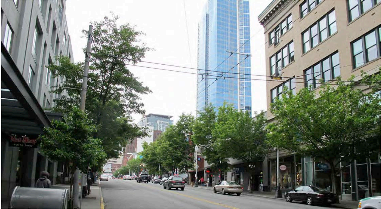
Figure 42: View looking north on First Avenue.
