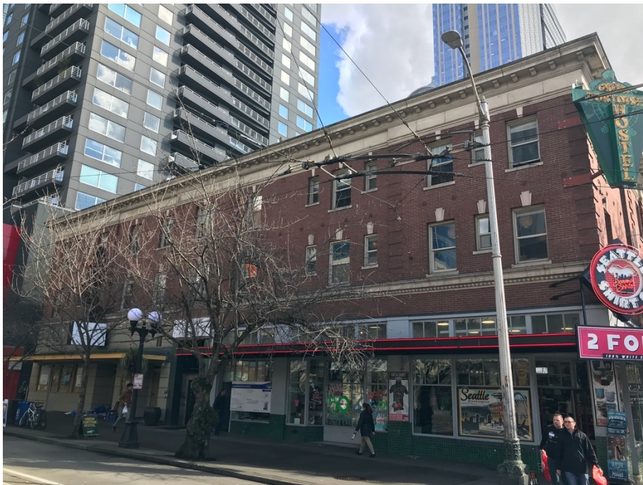
Figure 25: North facade of Hahn building.
