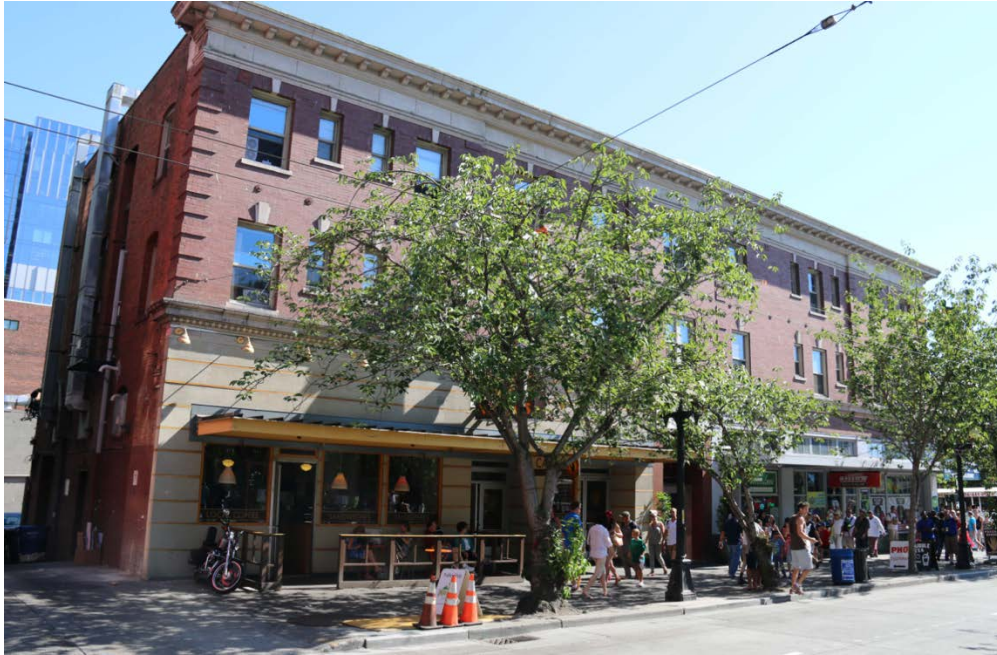
Figure 28: North facade showing EIFS detailing and storefront alterations.
