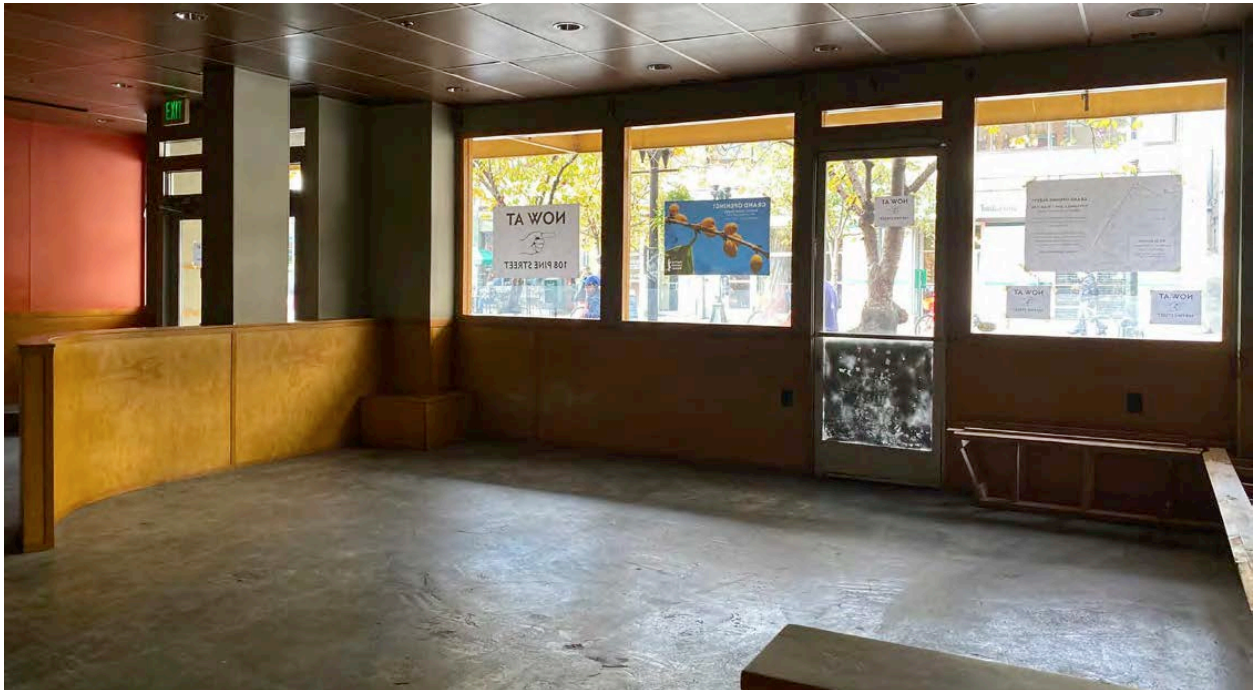
Figure 37: Interior of former restaurant (from TJP report, 2014).
