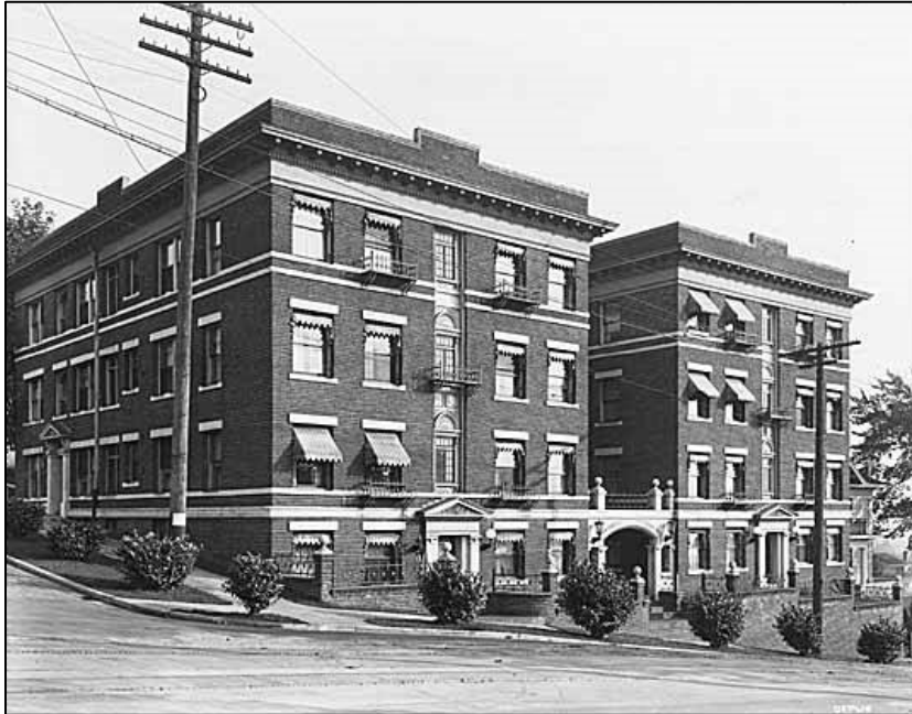
Browne-Cassel Apartments, now Castle Court (1915) 844 Queen Anne Avenue N
