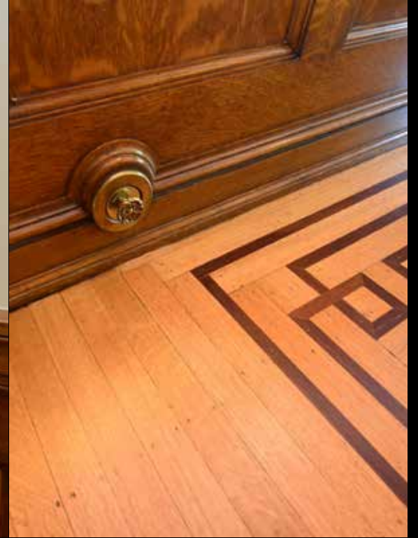
Tuc central vacuum cleaning system port and detail of wood floor.
