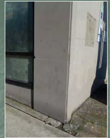
Cement Board Corner Wrap
