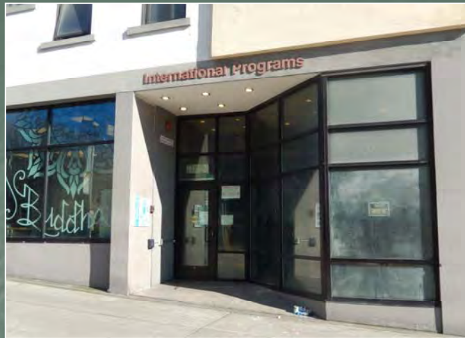
Bronze Storefront at Southwest Corner
