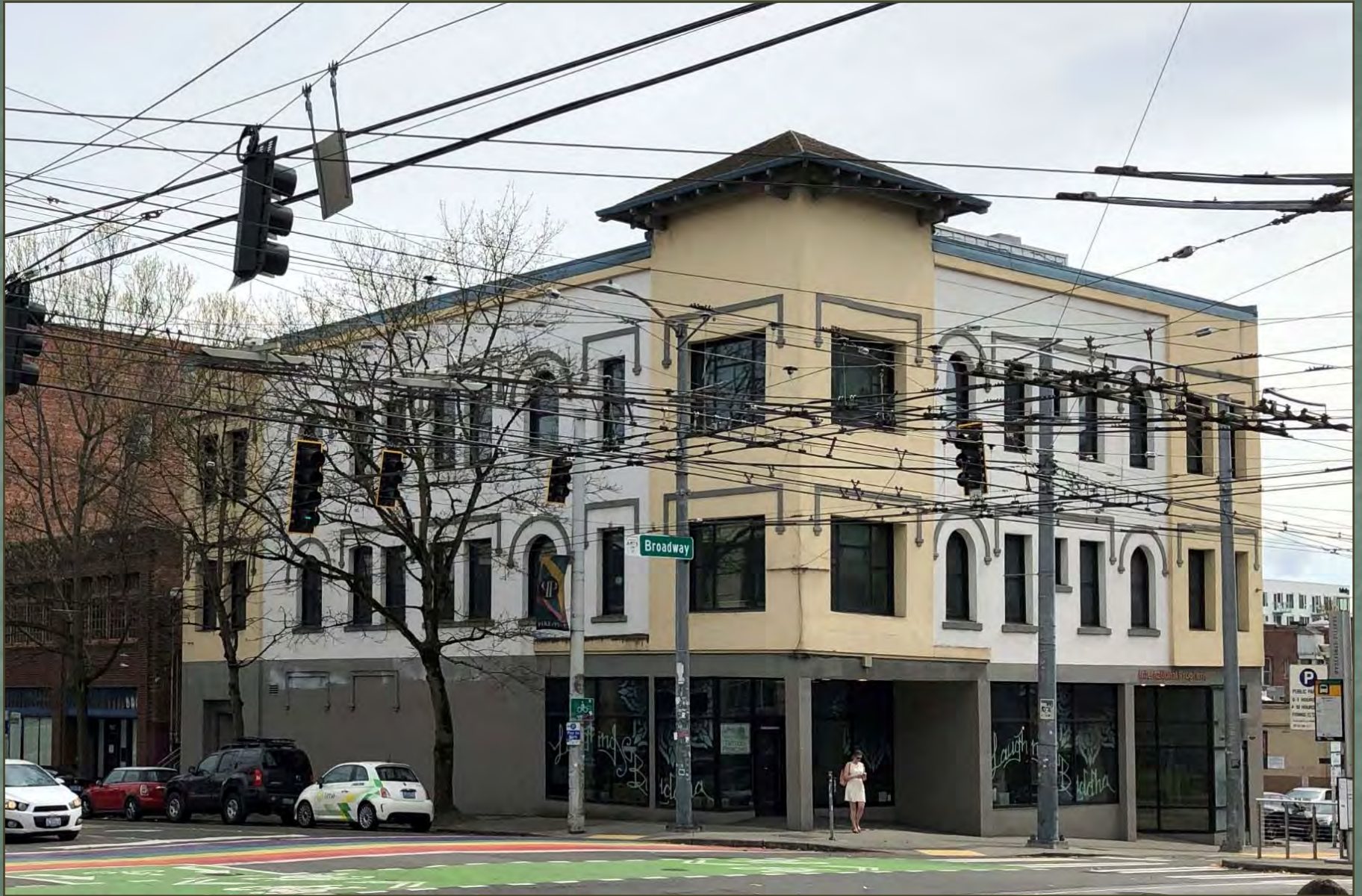
Booth Building (1906) Landmark Designation YouthCare & Capitol Hill Housing
