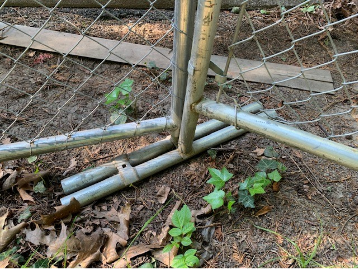
Temporary security fence footings as installed.
