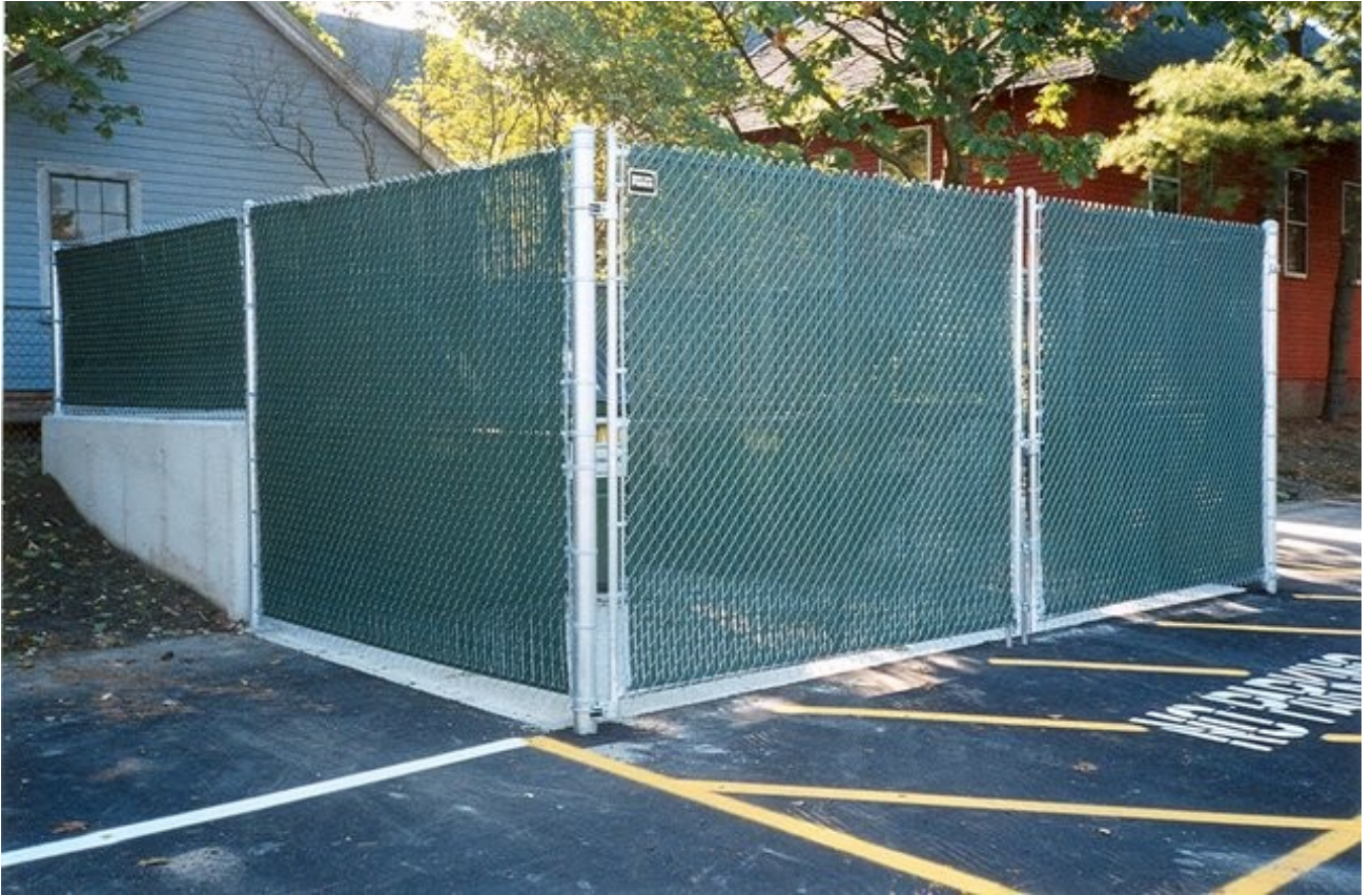
Example vinyl screening planks installed in chain link fence
