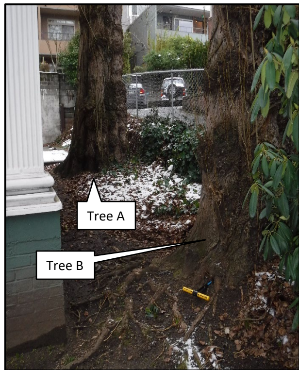
Photo 2. Base of tree B with 40-inch steel probe fully inserted into cavity at base. This photo was taken in January 2020, during the first visit we performed to evaluate the trees for risk.
