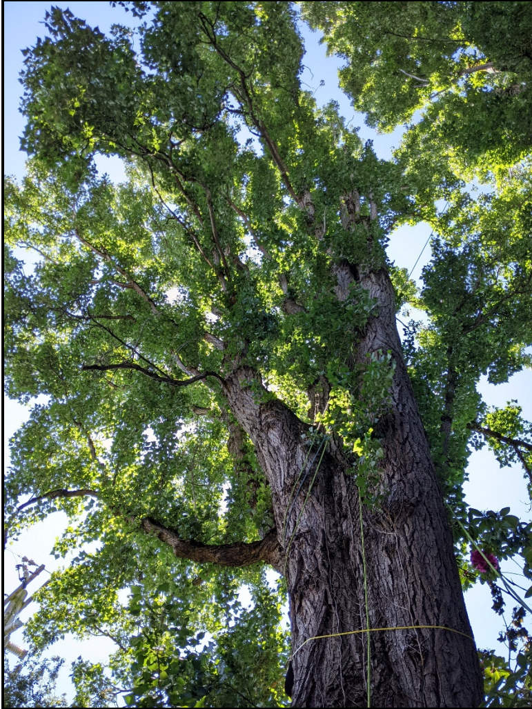
Photo 7. Tape around trunk of tree D indicates level at which test 6 was conducted (see Figure 16). The results of this test showed just over two inches of sound wood; this test result was the most concerning of all in our opinion because of how much tree material is supported by the weakened trunk of this tree.
