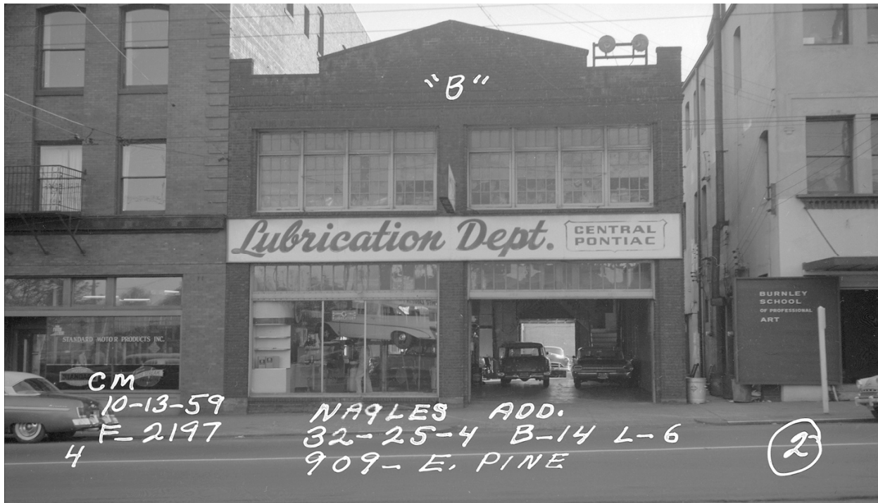
Fig 41 This 1959 tax record photo shows the building following storefront changes. Note the east storefront has been replaced with a large fixed unit. (Puget Sound Regional Archives)
