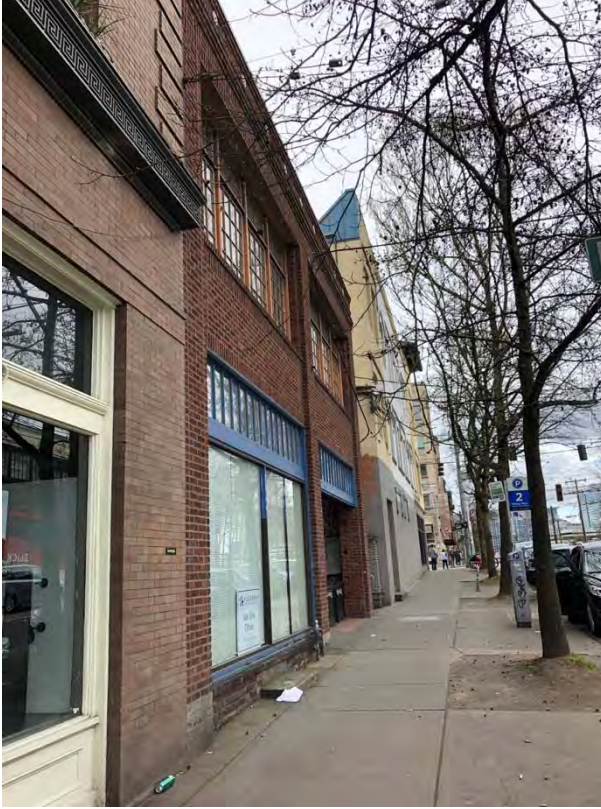
Figs 15 & 16 Two storefront views. Left, note the remaining step that indicates where the original storefront entry was located. Right, infill and contemporary storefront behind the original transom.
