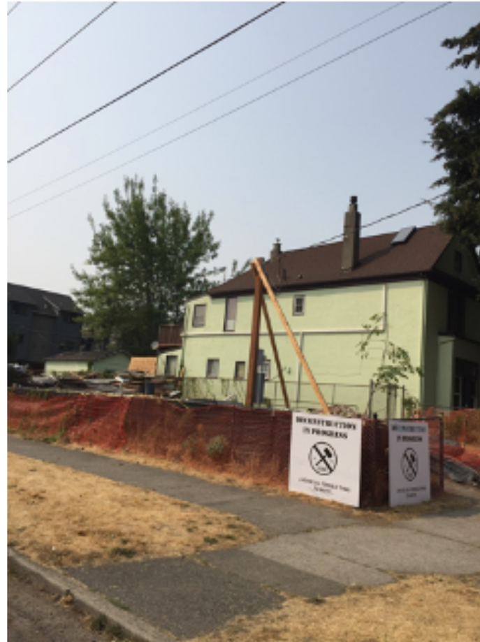
"Deconstruction in Progress / A House is a Terrible Thing to Waste"
