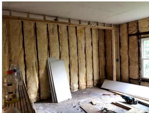
Master Closet Framing and Insulation
