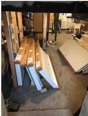
New basement electrical, framing, and doors for upstairs
