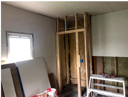
Bedroom 2 Framing and Drywall
