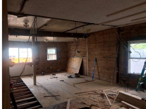
2 Bathroom and Pantry Demo to become Dining
