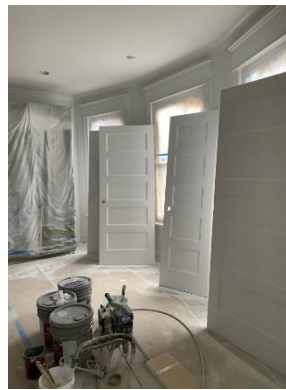
Trim, Paint, and Doors
