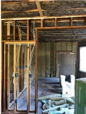
Unit 1 Framing + Electrical
