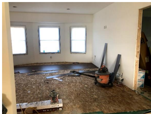
Floor Sound Insulation and Plywood
