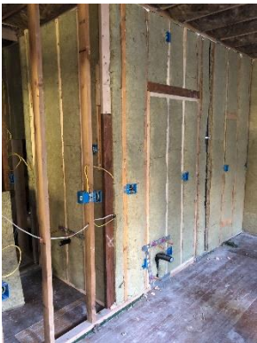
Unit 1 Kitchen & Bathroom Plumbing, Electrical, & Unit Barrier Insulation
