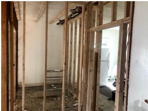
Bedroom 3 and Laundry Framing
