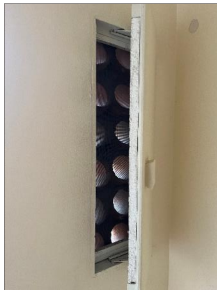
Figure 121: Anhalt (1-bedroom unit) – Interior view of bedroom window ventilation system (Unit 72, Camera facing Southeast)
