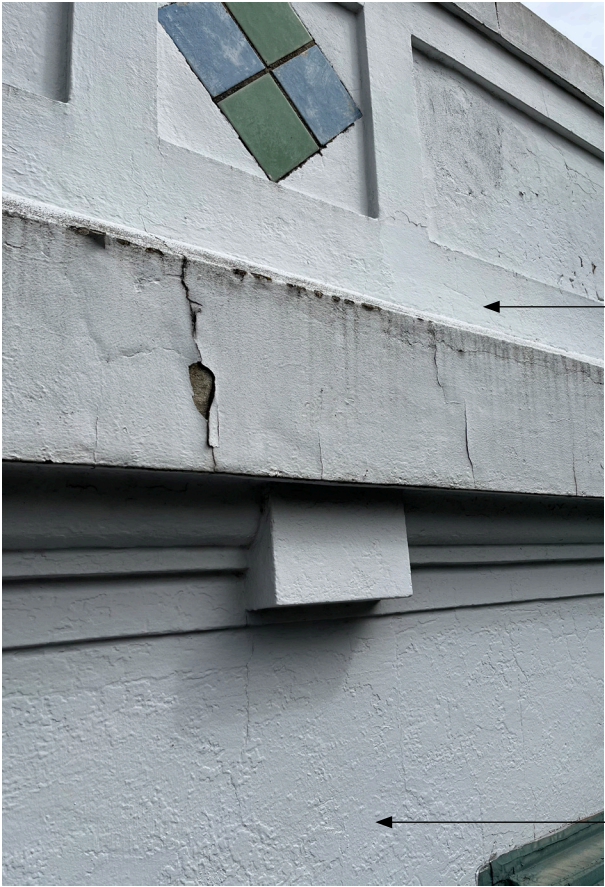
TYPICAL BANDING; PAINT OVER CEMENTITIOUS BLOCK
