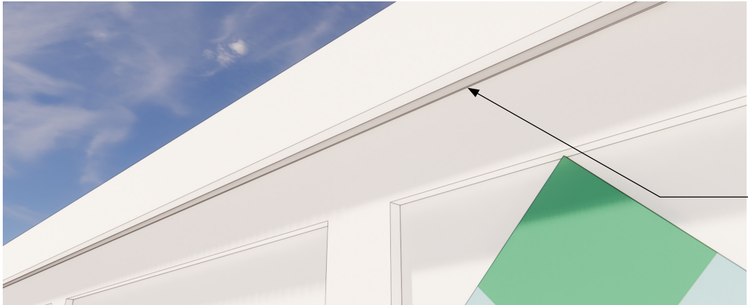
CLOSE-UP OF COPING FLASHING
