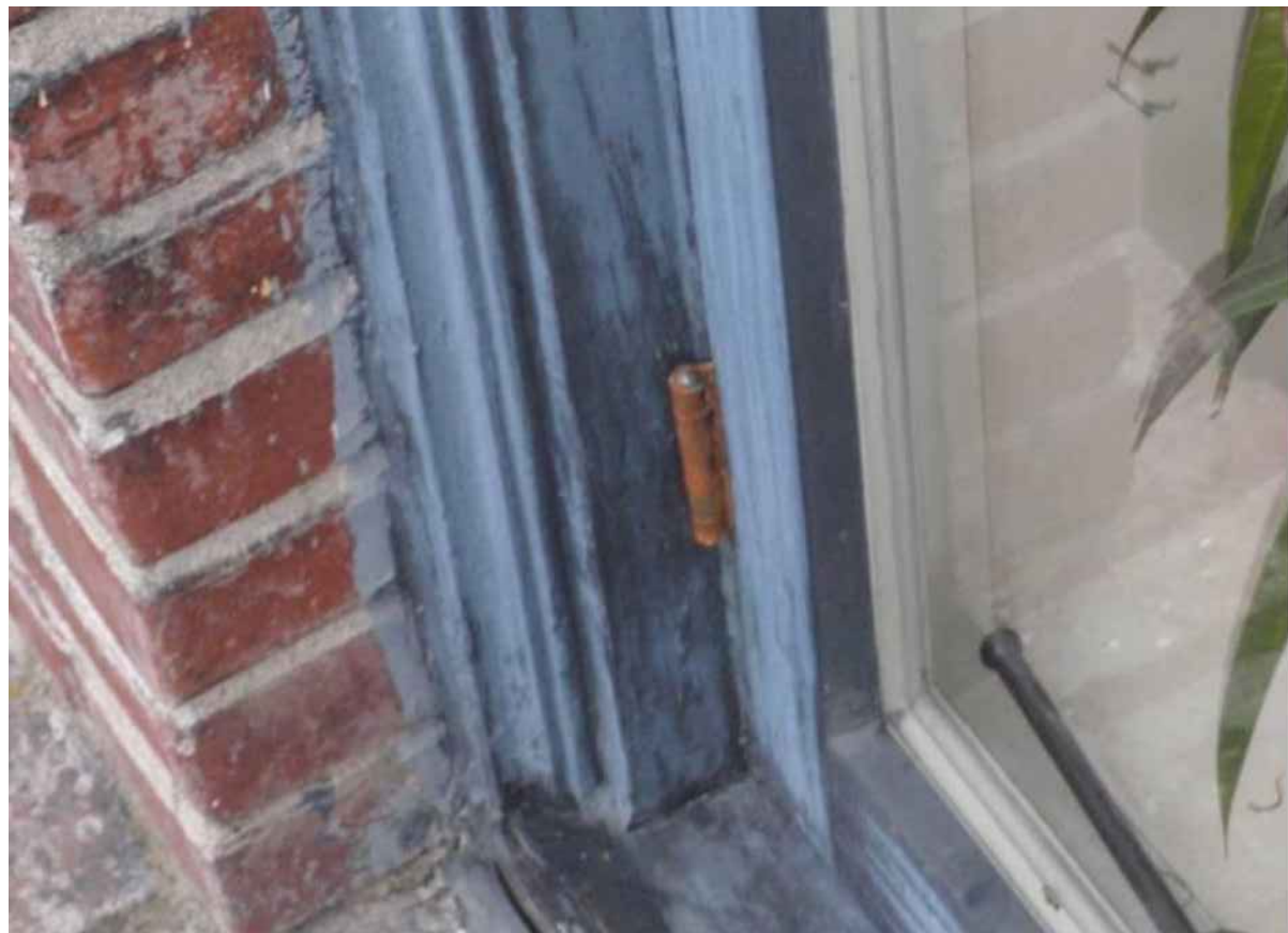
8 RUSTING WINDOW/DOOR HARDWARE EXAMPLE
