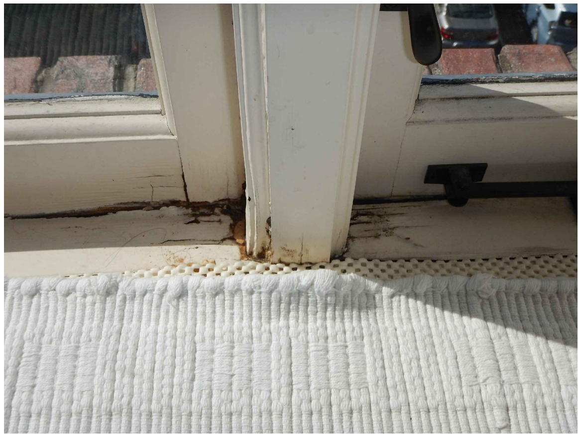
4 INTERIOR FRAME DAMAGE EXAMPLE
