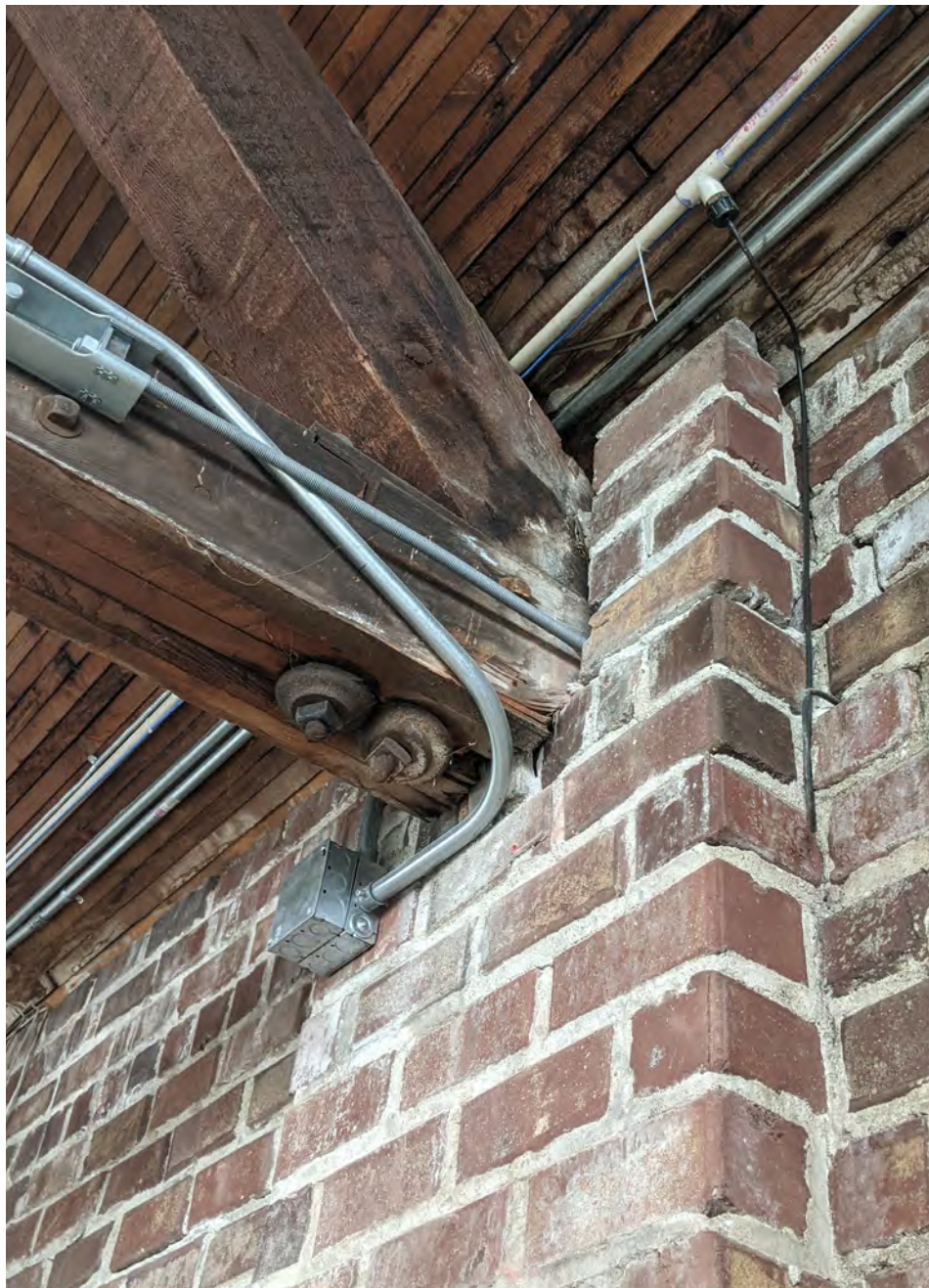
Existing interior conditions - truss, NLT roof and brick
