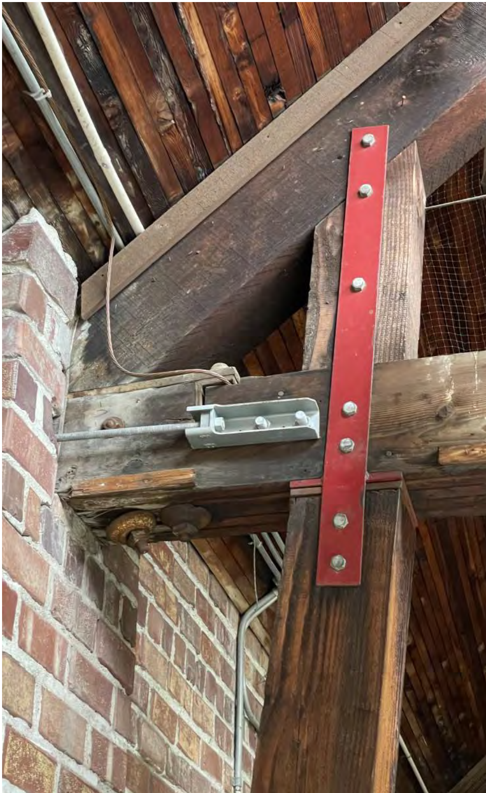
EXISTING TRUSS TIMBER SUPPORT AT PILASTER
