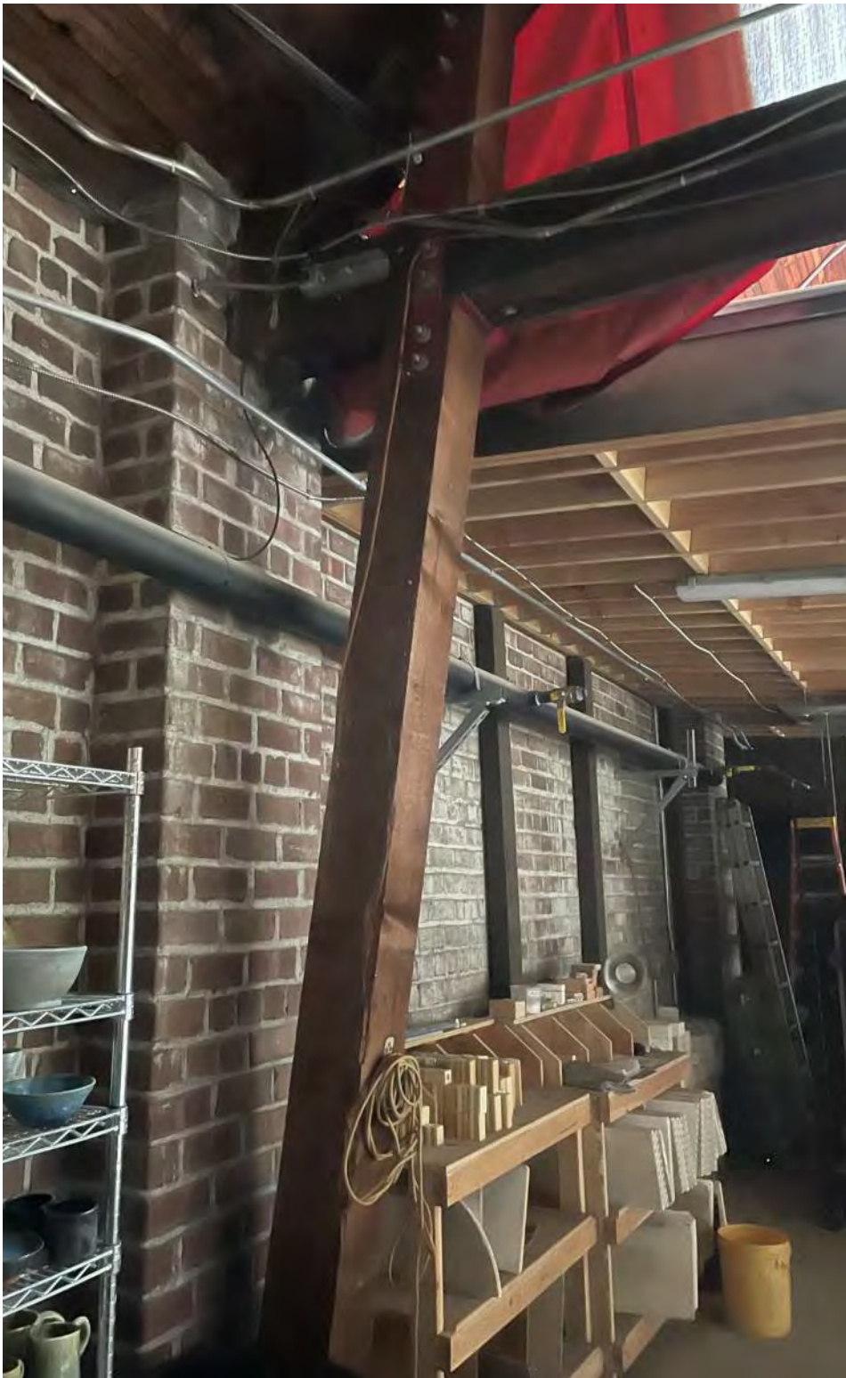
EXISTING TRUSS TIMBER SUPPORT
