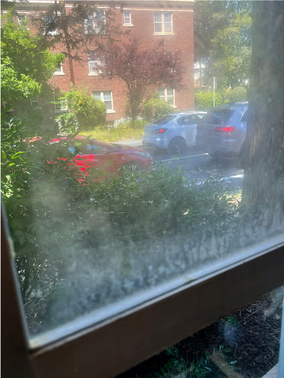
Example of condensation between panes of an existing non-original window.
