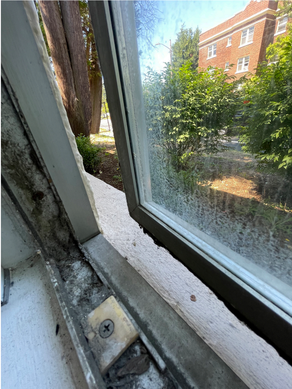
Example of degraded frame condition at an existing non-original window.
