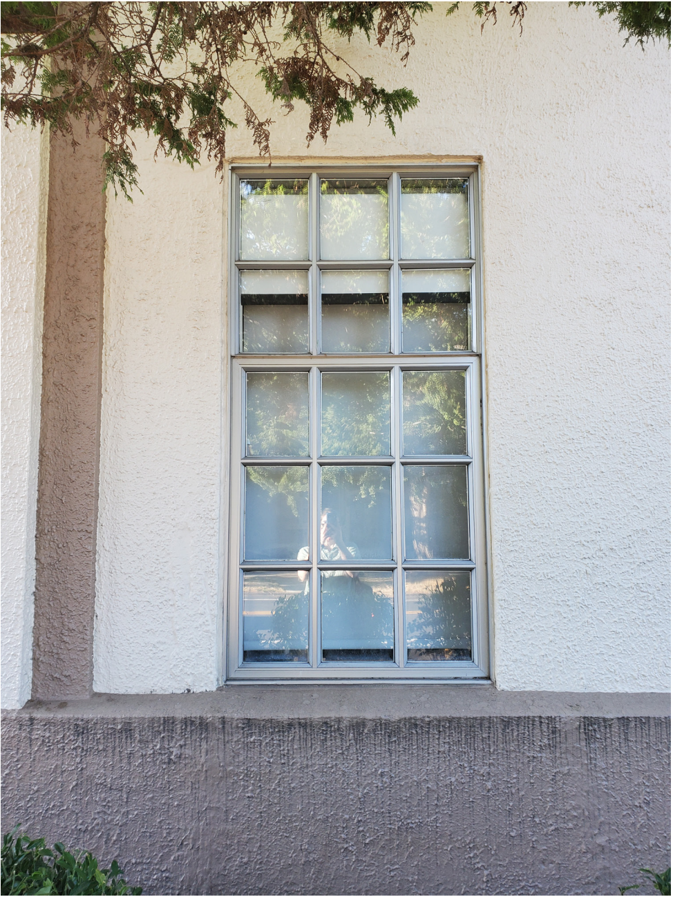
Close-up of a typical non-original window to be replaced.
