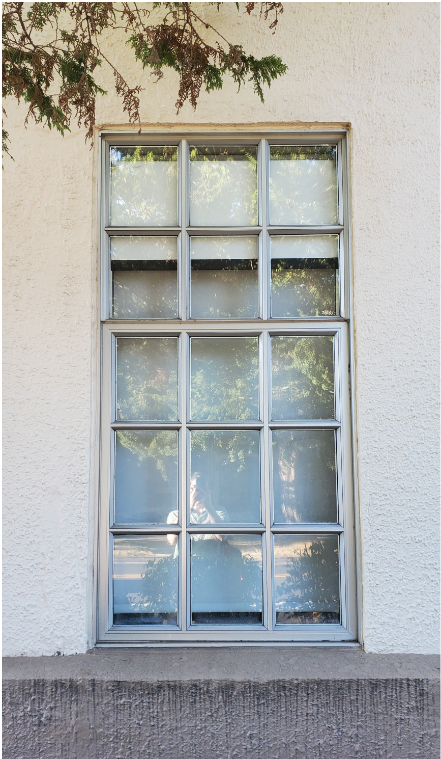
IMAGE 03. ACTUAL DIVIDED LITE PATTERN AND CASEMENT OPERATION OF ALL (5) NON-ORIGINAL WINDOWS TO BE REPLACED.
