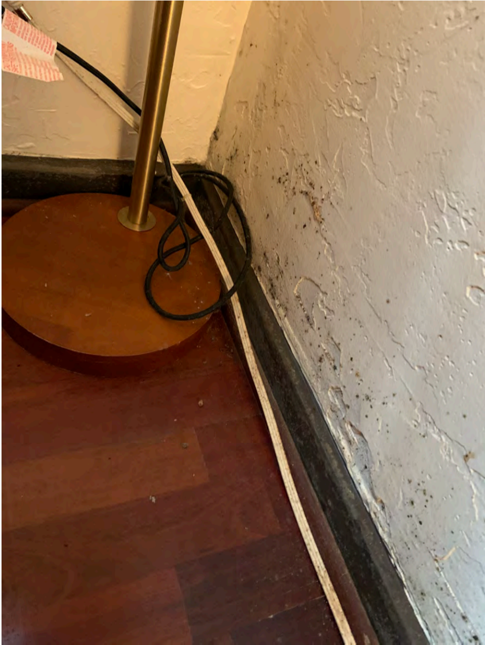
Mold growth at Northwest corner of Unit 107
