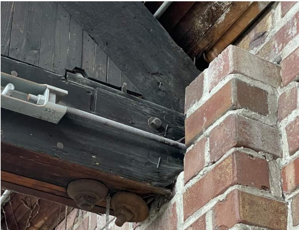
Existing truss condition at courtyard
