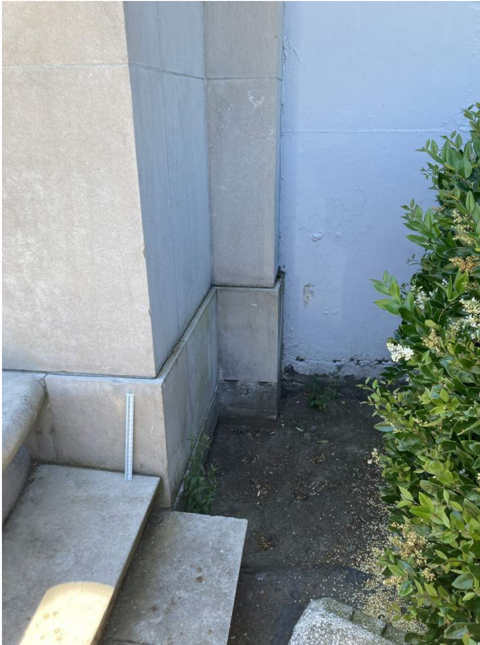
North Memorial Stone Wall and Stadium Concrete Wall at Grade - Chipping at Exposed Slab and Corner
