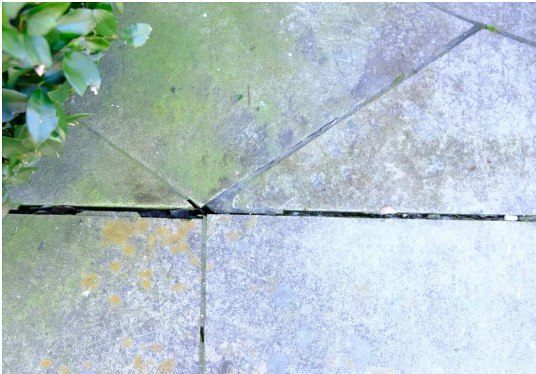
Areas of mortar loss, surface dirt, organic growth at walking surface pavers
