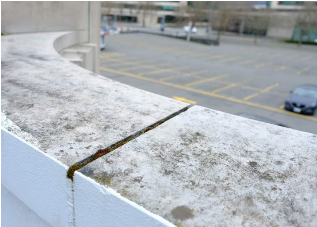
Mortar loss and organic growth at sky-facing mortar joints
