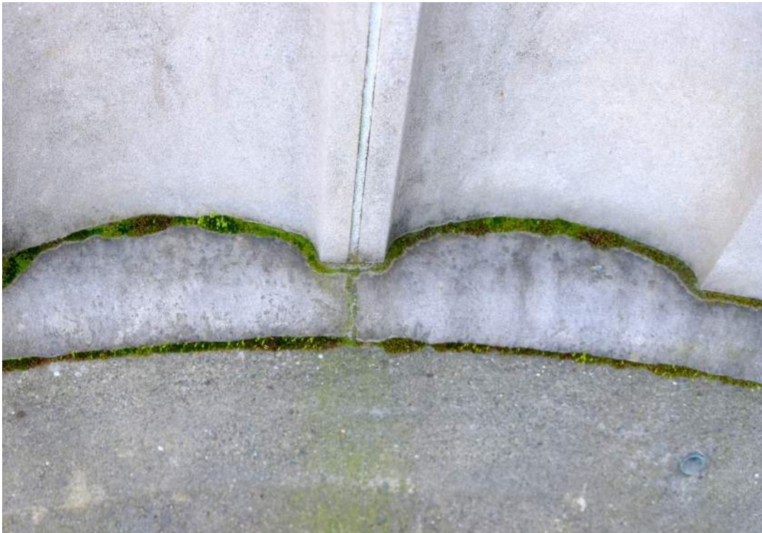
Areas of surface damage, organic growth, and dirt
