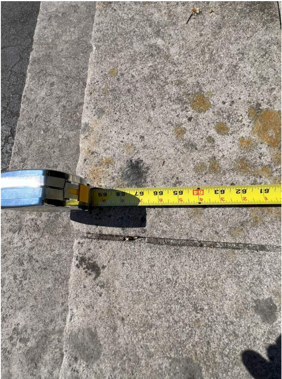
Memorial Steps - Stone Joint, Discoloration, and Moss
