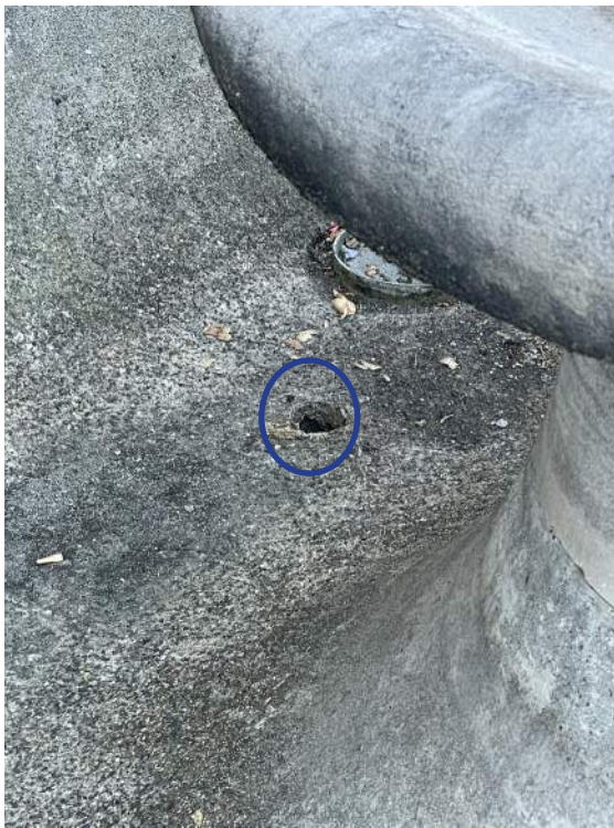
Water Outlet at Basin Low Point
