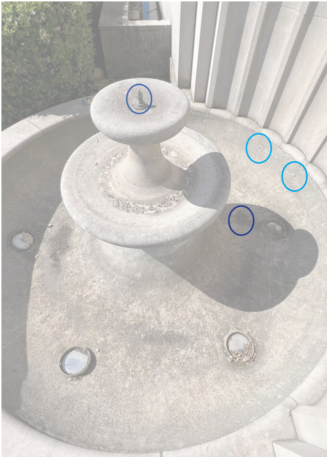
North Fountain Basin - Water Inlet and Outlet Locations
