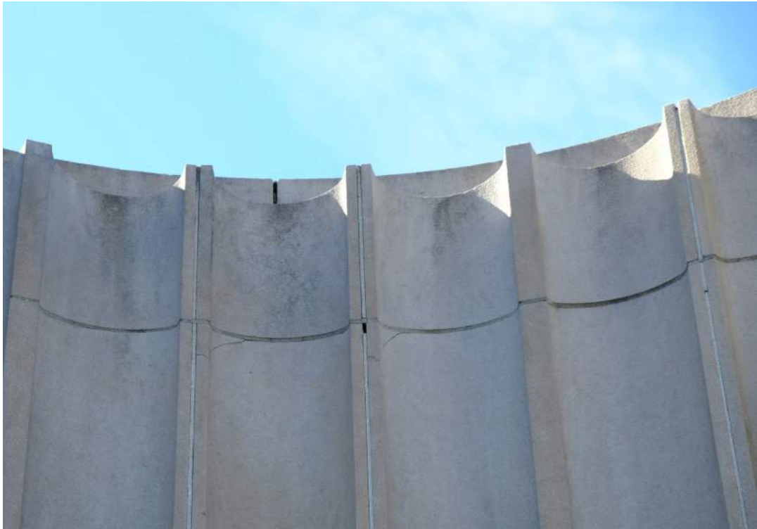
Areas of mortar loss, stone cracking, and surface dirt
