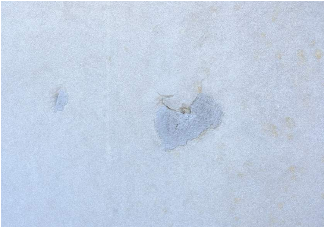
Surface damage with a previous repair patch that has failed
