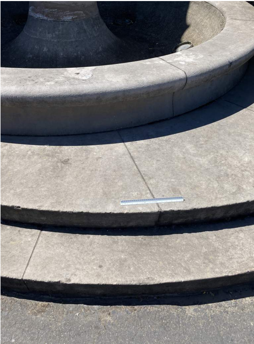
South Basin Steps - Nosing Chips and Discoloration
