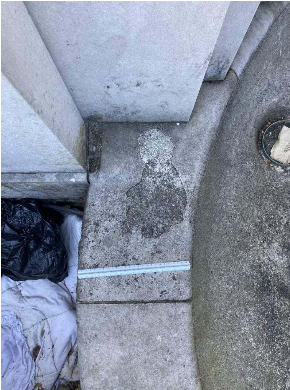
South Fountain Basin Edge - Stone Deterioration
