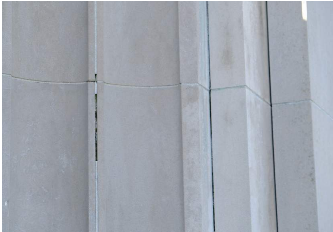
Areas of mortar loss
