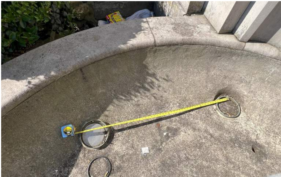
North Fountain Basin Lights - Fixture Hardware Condition
