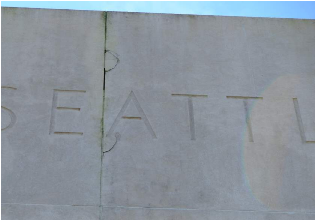
Areas of mortar loss, surface damage, and organic growth
