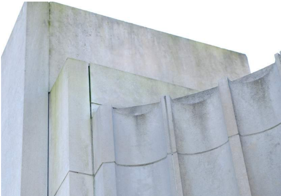
Areas of mortar loss, surface dirt, and organic growth
