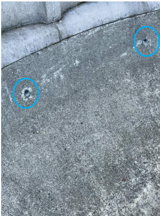
Water Overflow Pipes at Rim
