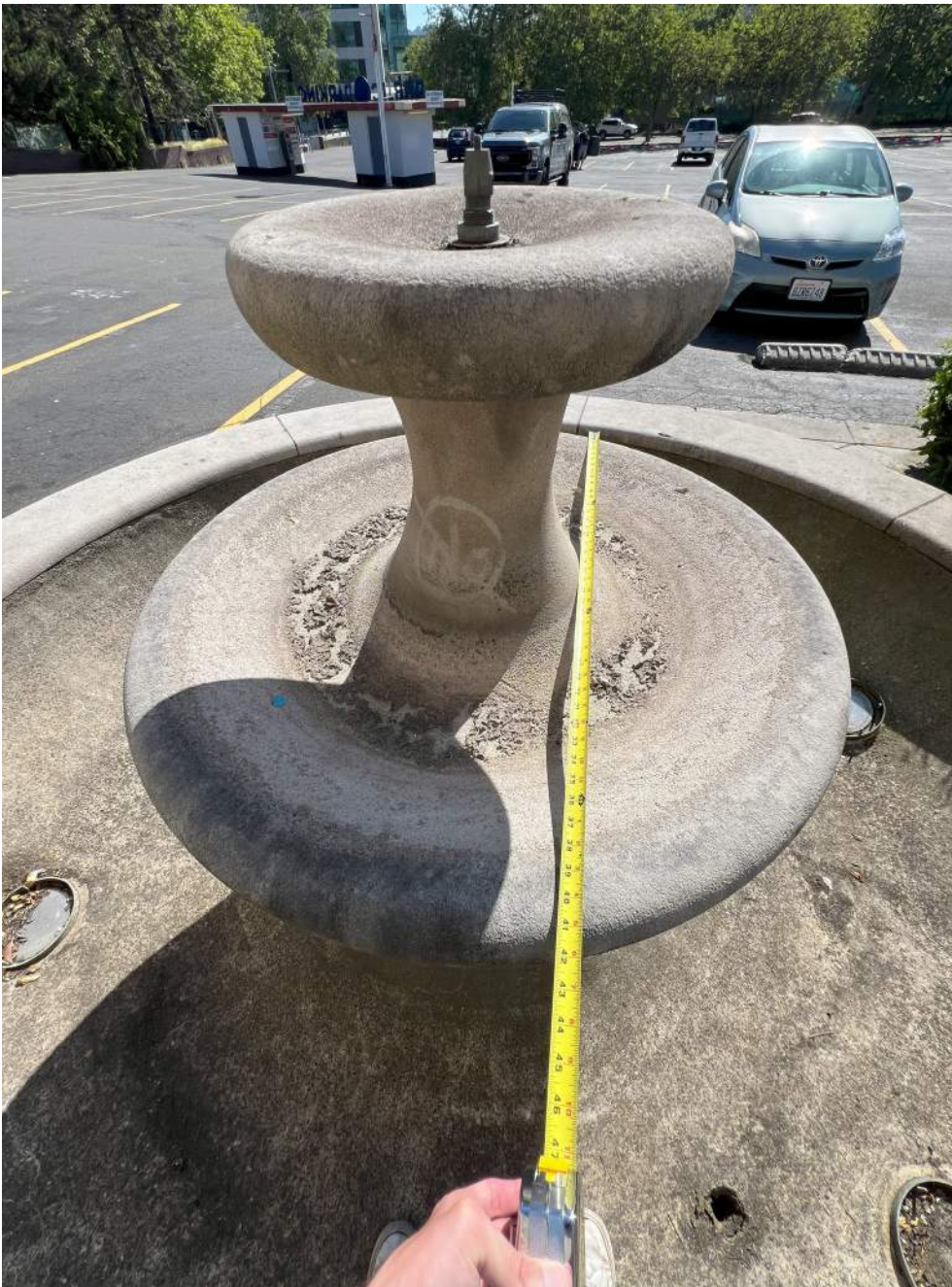
South Fountain Basin Tower - Stone Markings and Discoloration
