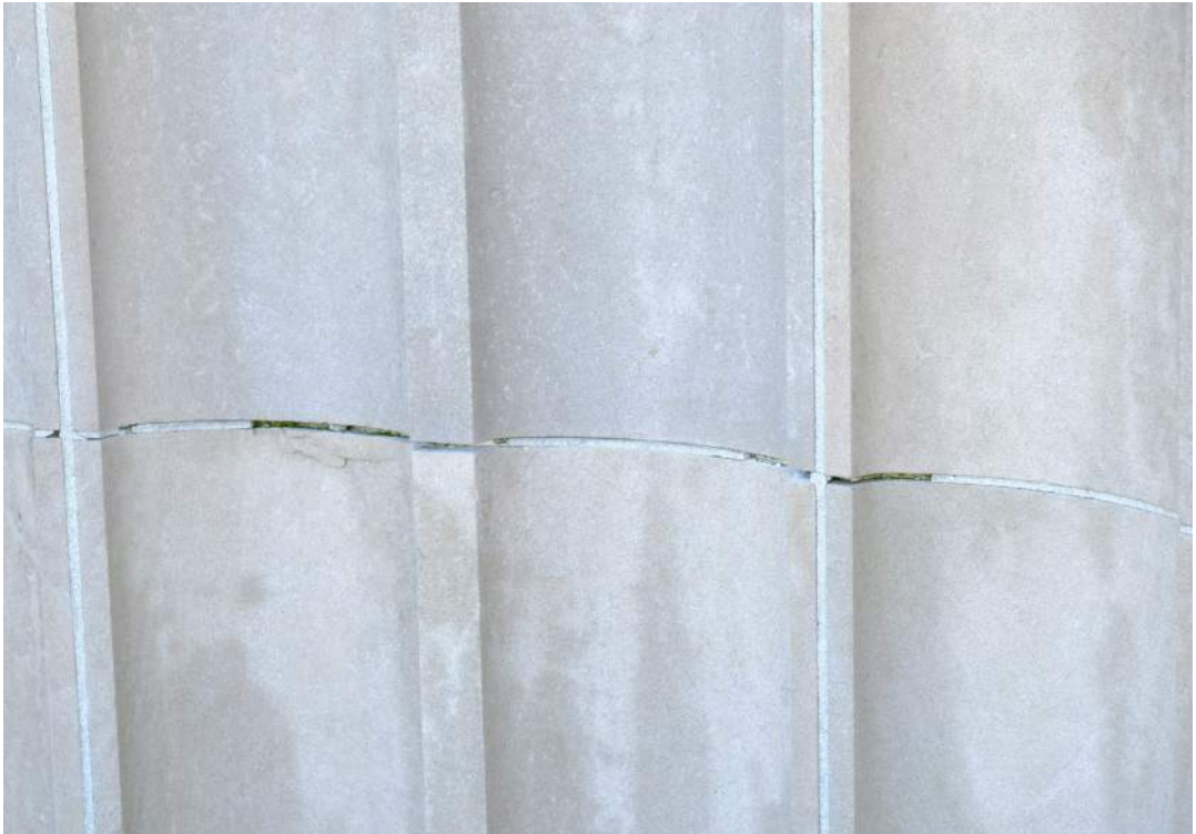
Areas of mortar loss
