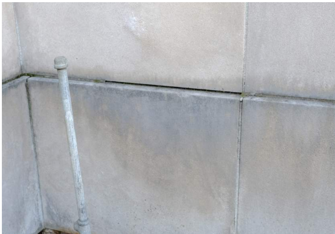
Areas of mortar loss and surface dirt
