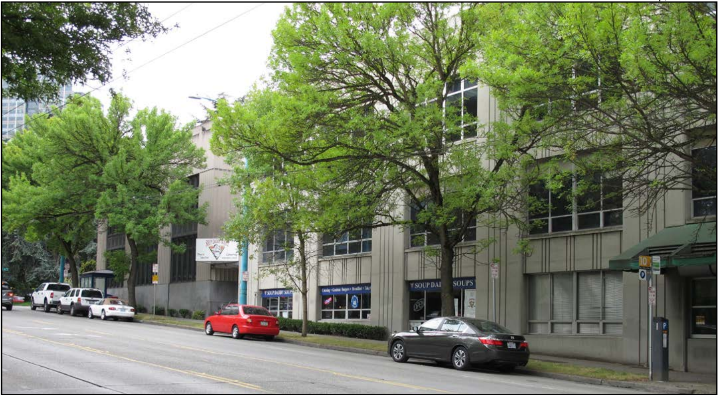
Figure 12 • Seattle Times Building Complex, Printing Plant and Office Building viewing southwest on Fairview Avenue N
