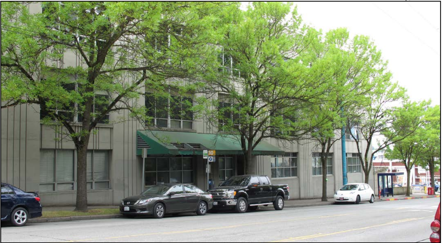
Figure 14 • Seattle Times Building Complex, Printing Plant viewing southwest on Fairview Avenue N
