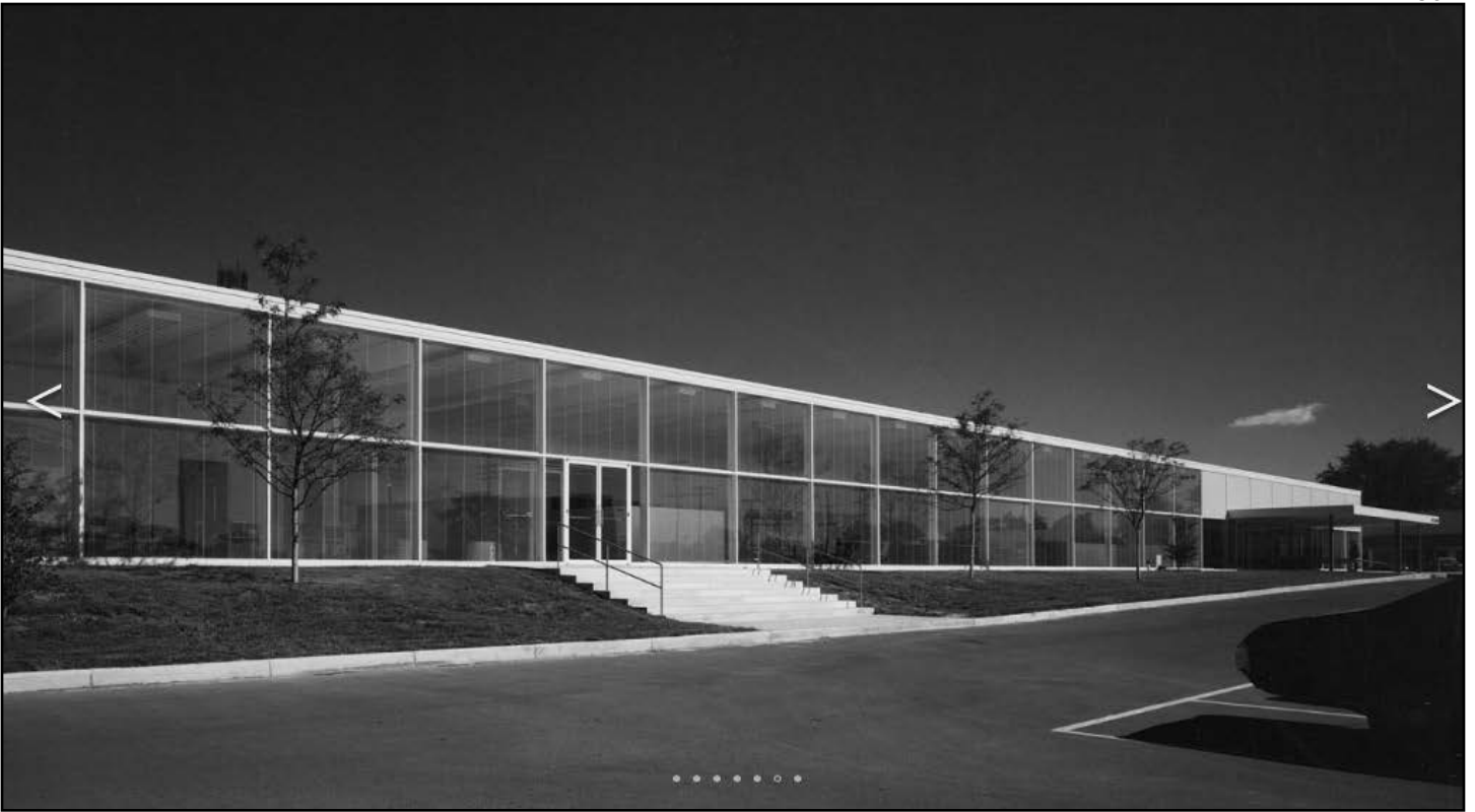
Figure 82 • Republic Newspaper Plant and Office, Columbus, Indiana (1971, SOM)
