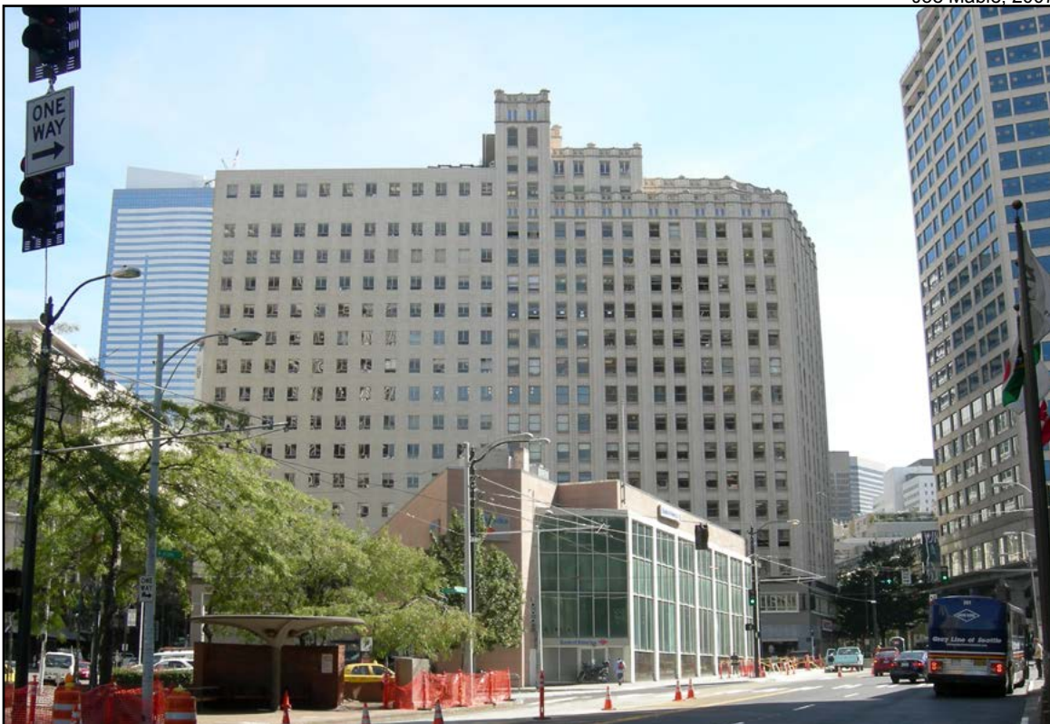
Figure 96 • Addition (left) to Seattle's Medical Dental building (1949, Wililam H. Fey for the Metropolitan Building Company)
