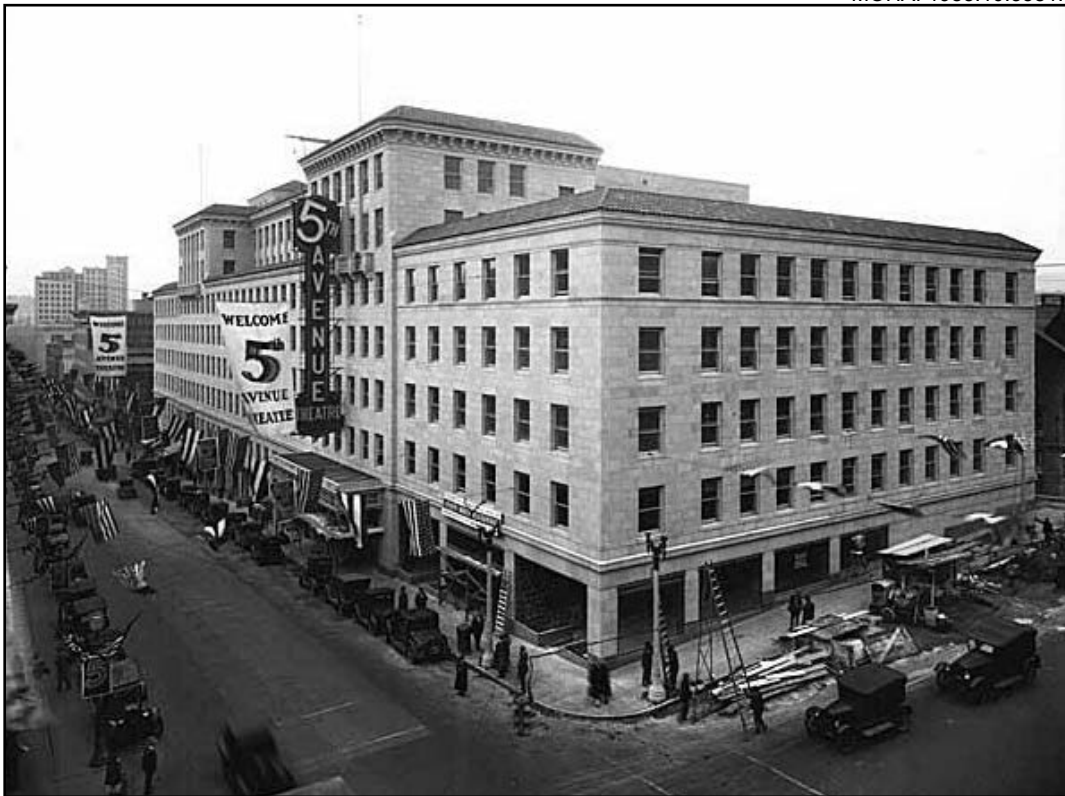
Figure 90 • Skinner Building, Seattle (1925-26, Robert C. Reamer, Teufel & Carlson, contractors)
