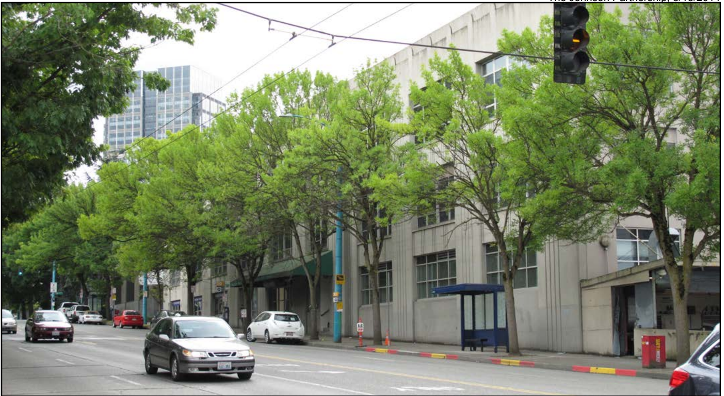
Figure 11 • Seattle Times Building Complex, Printing Plant, viewing southwest on Fairview Avenue N
