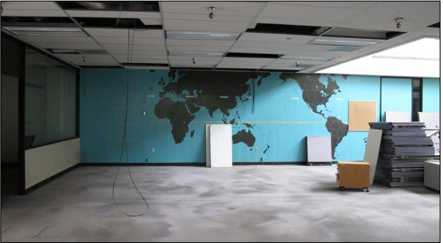
Figure 24 • Seattle Times Building Complex, Printing Plant, pressroom
