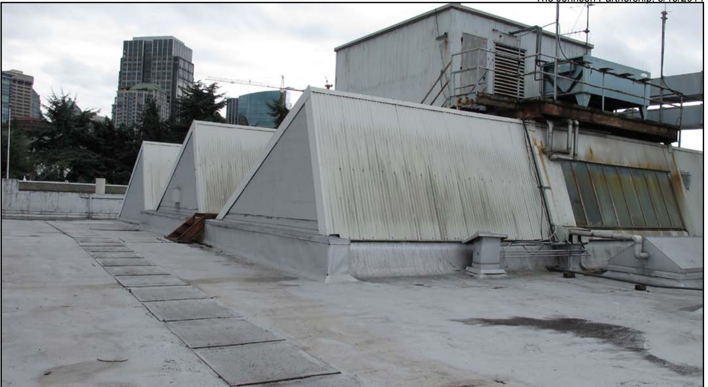
Figure 19 • Seattle Times Building Complex, Printing Plant skylight roof monitors
