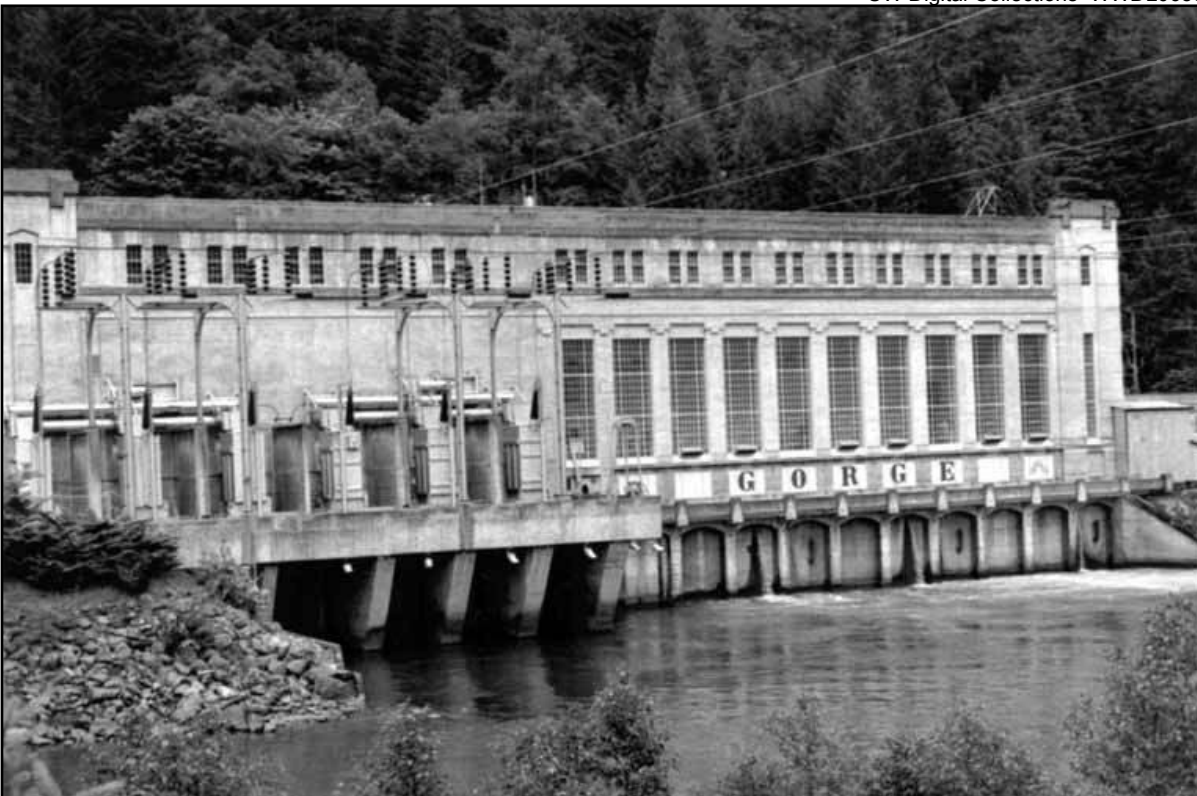
Figure 100 • Seattle City Light Gorge Powerhouse (1937, Teufel & Carlson, contractors, National Register District)
