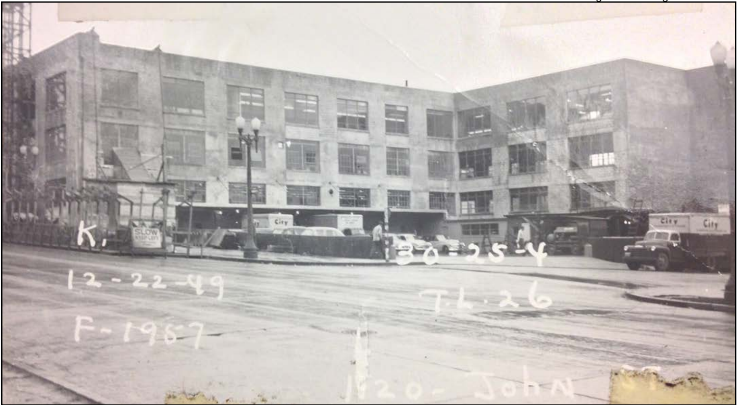
Figure 48 • Seattle Times Building Complex, Printing Plant viewing southwest, 1957
