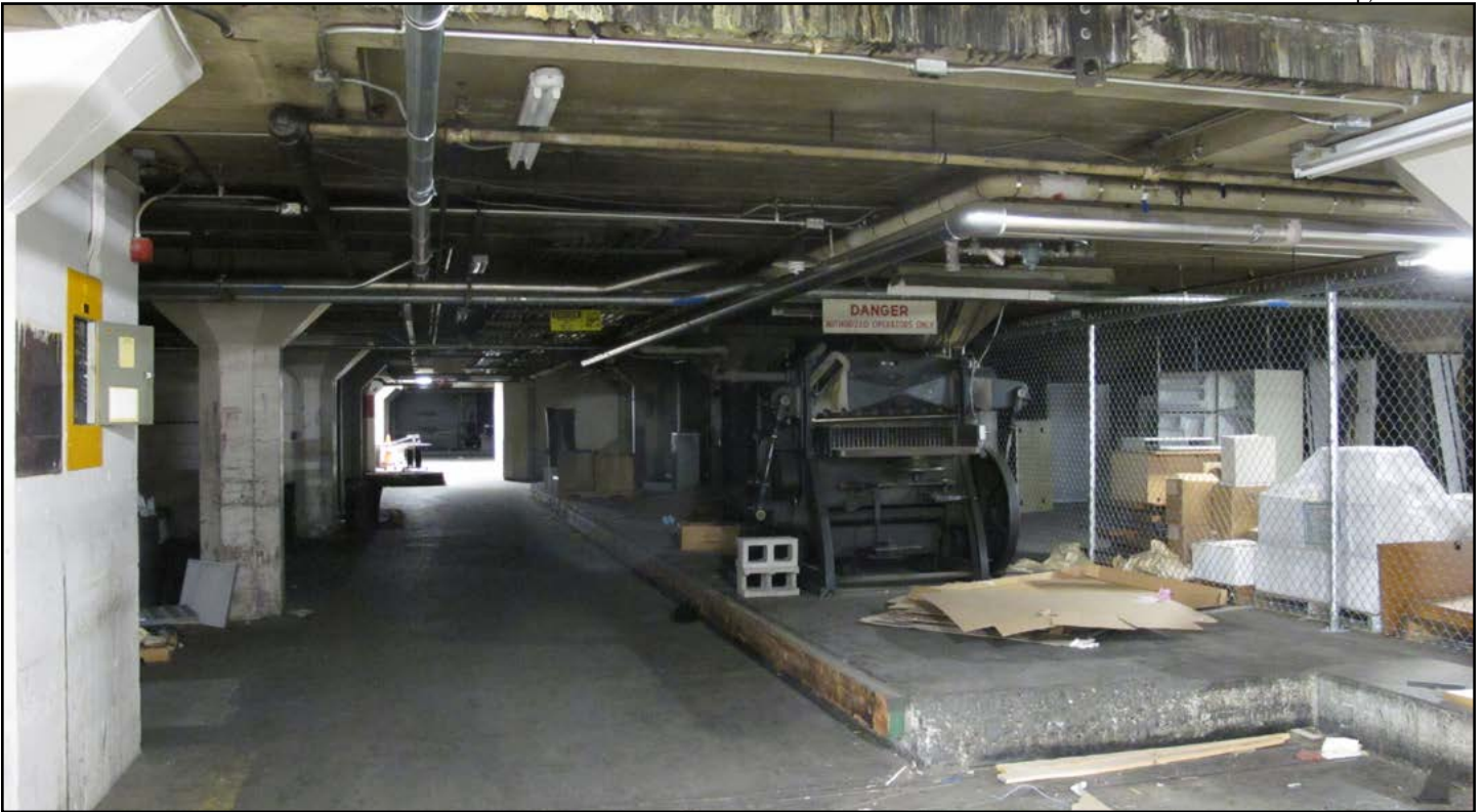
Figure 22 • Seattle Times Building Complex, Printing Plant , basement
