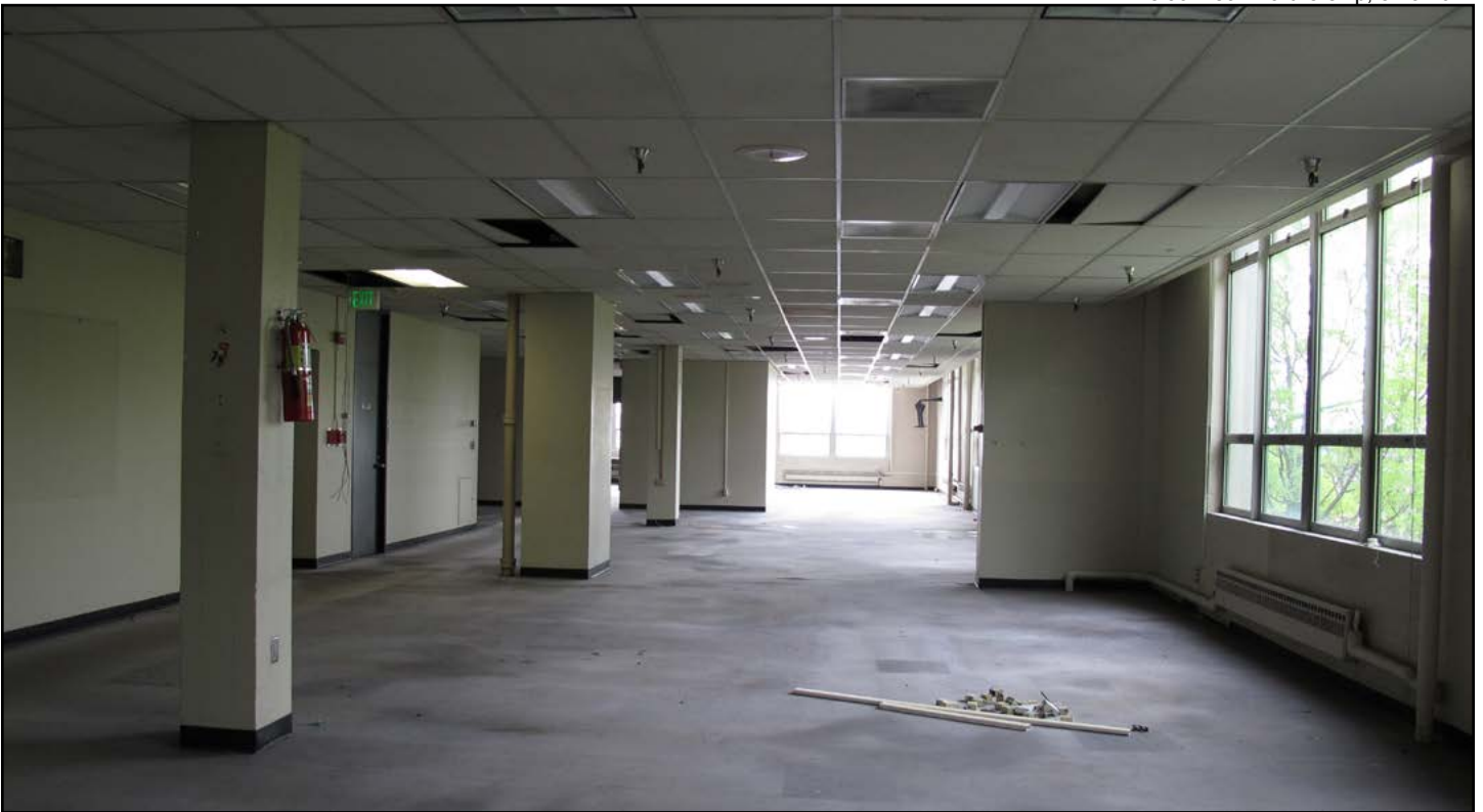
Figure 23 • Seattle Times Building Complex, Printing Plant, newsroom, southeastern corner
