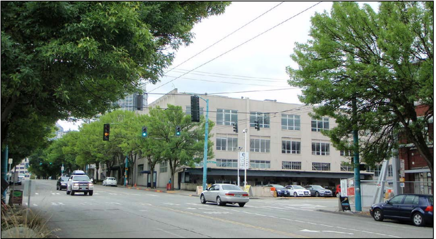
Figure 10 • Seattle Times Building Complex, Printing Plant, viewing southwest on Fairview Avenue N
