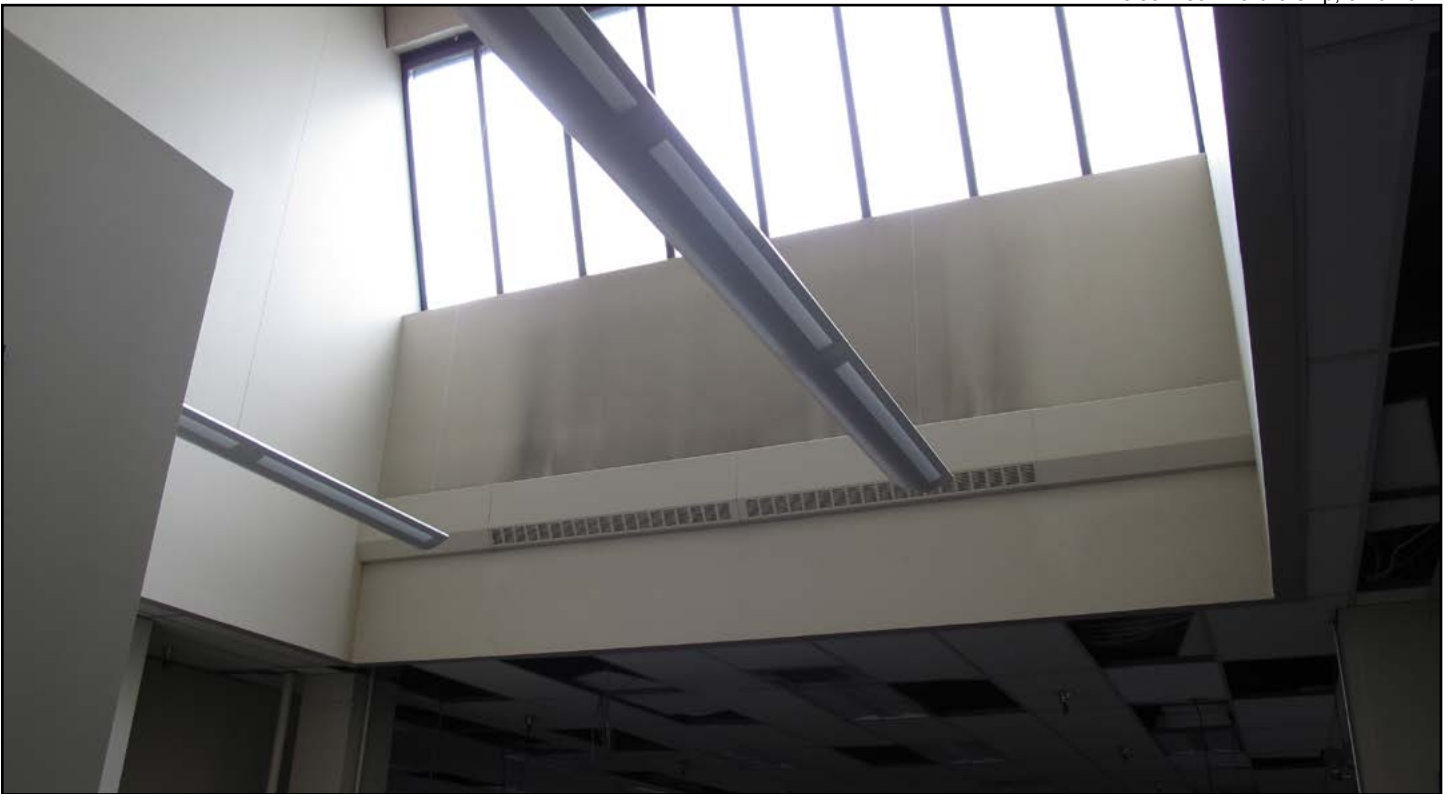
Figure 25 • Seattle Times Building Complex, Printing Plant, original interior skylights
