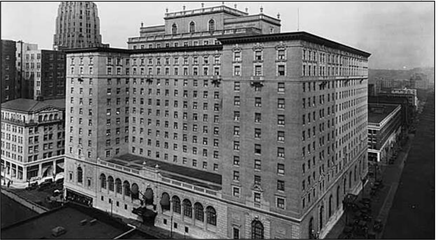
Figure 97 • Olympic Hotel (1924, George P. Post & Sons, Teufel & Carlson, contractors)
