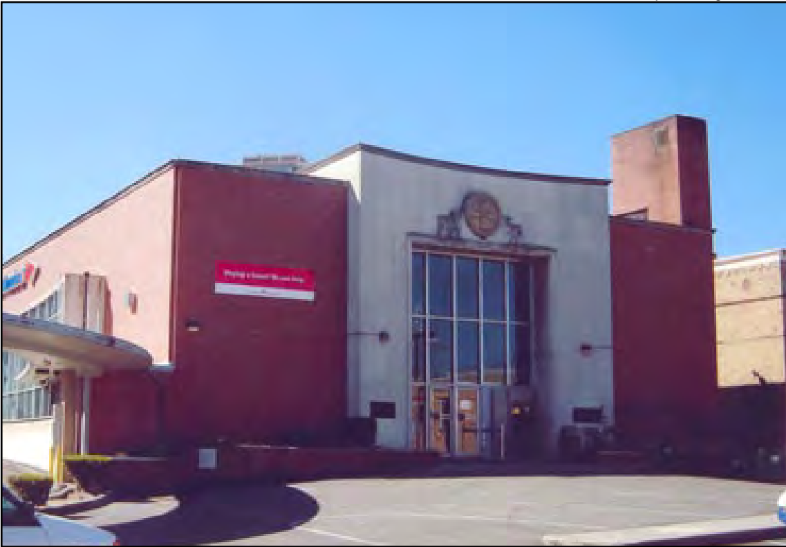
Figure 122. Seattle First National Bank, Denny Way Branch (1950, John W. Maloney Associates)
