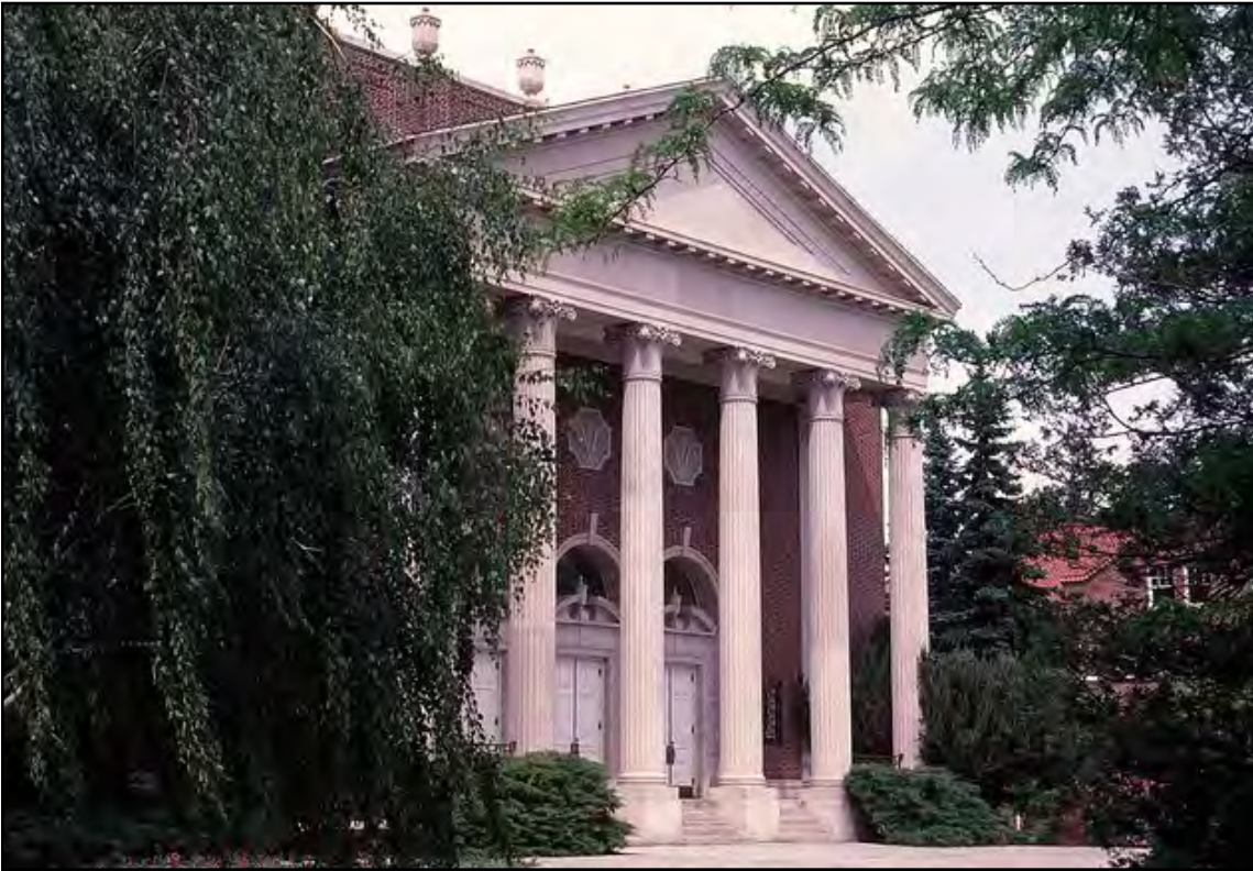
Figure 116. McConnell Auditorium, Central Washington University, Ellensburg, WA (1934-35, John W. Maloney Associates)
