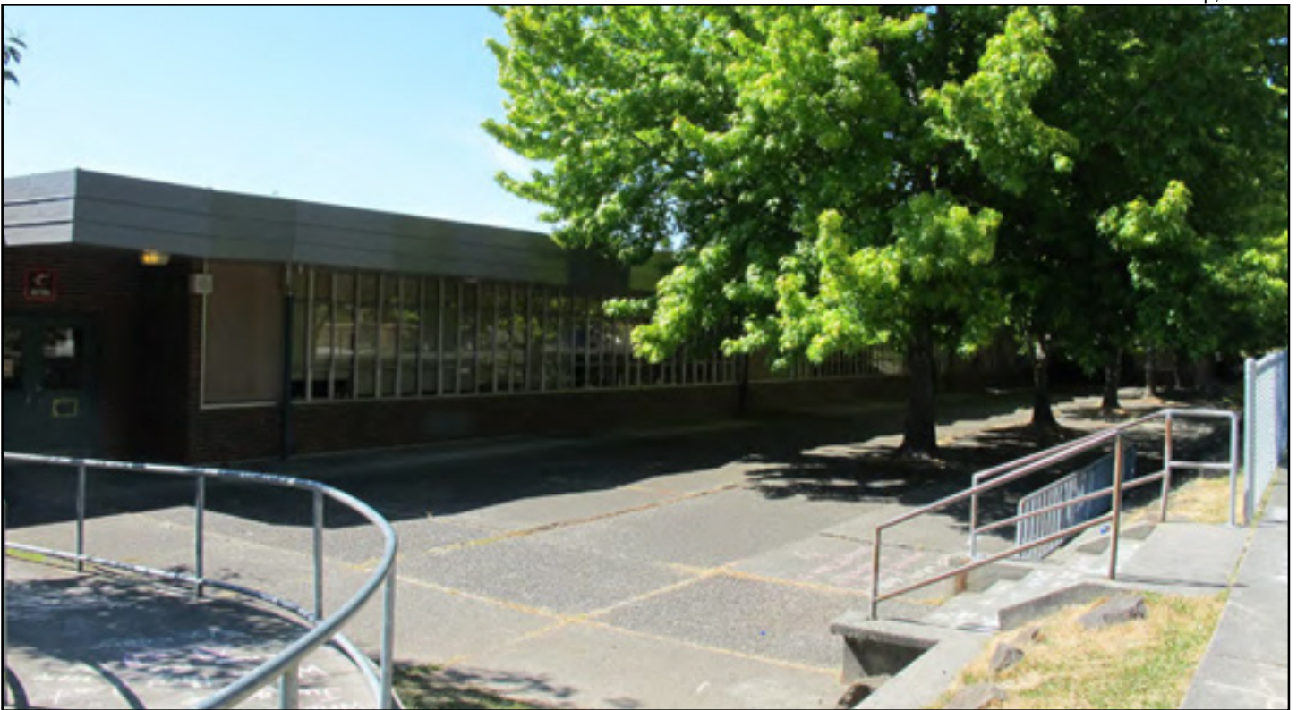
Figure 33. Edmund S. Meany Junior High, 1962 addition, Unit A, eastern façade viewing north (1962 Mahlum Addition)
