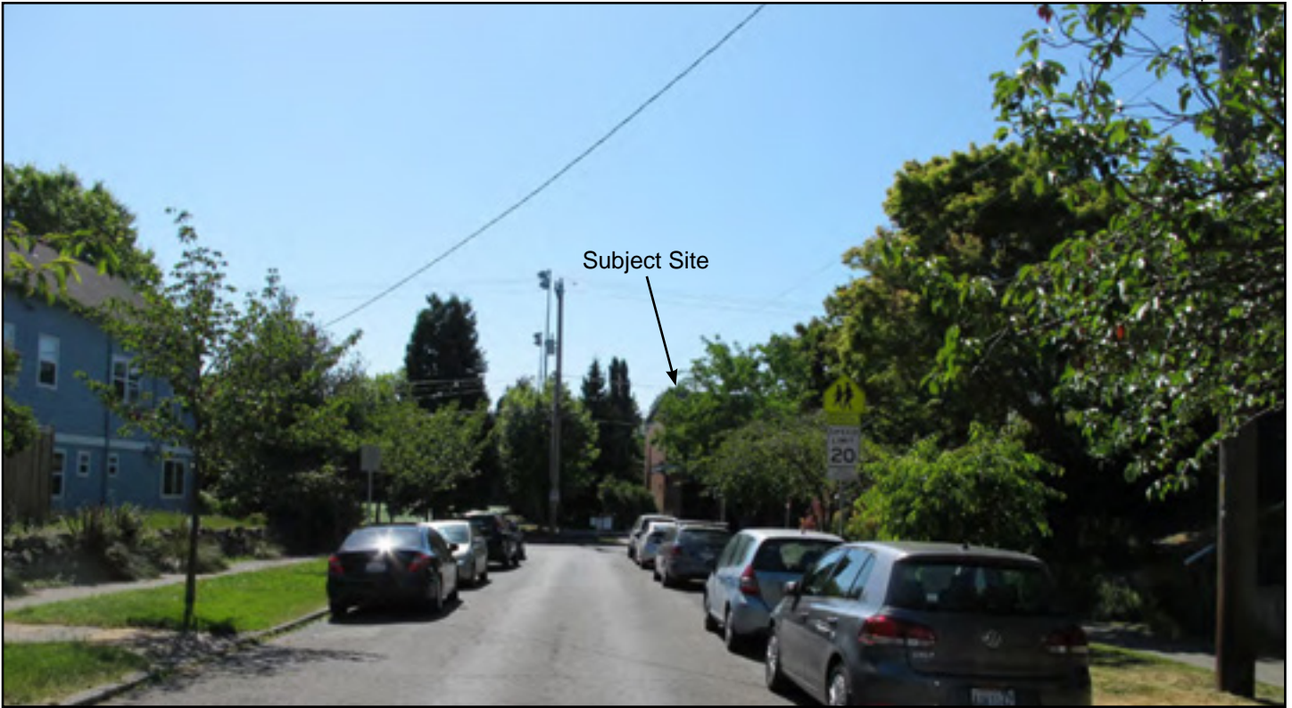
Figure 9. View E—Viewing west on E Thomas Street
