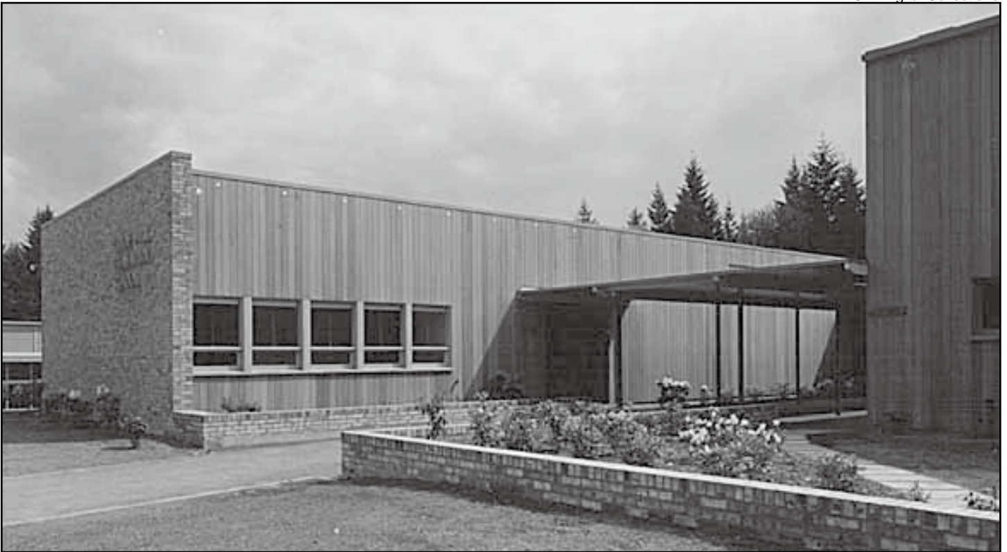
Figure 111. Clyde Hill Elementary School (1953, NBBJ)
