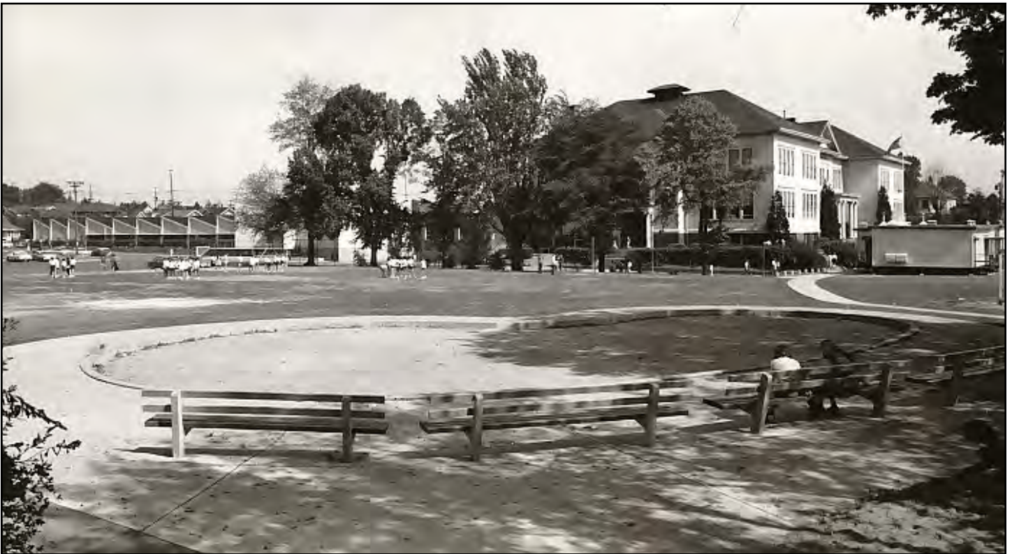
Figure 81. Edmund S. Meany School, viewing from the southwest, Maloney addition on the north, ca. 1955
