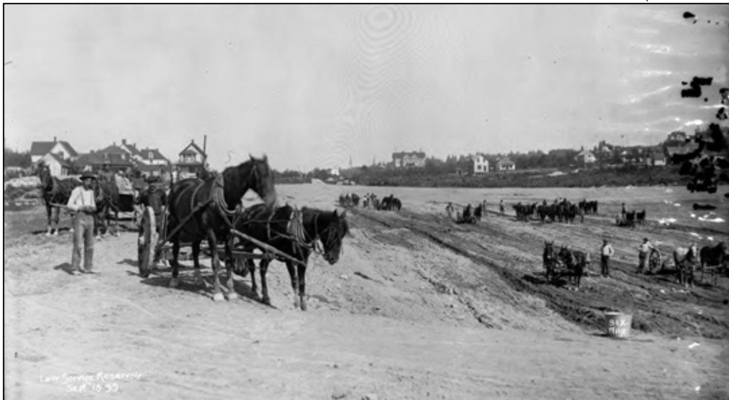
Figure 70. Lincoln Reservoir under construction, September, 18, 1899
