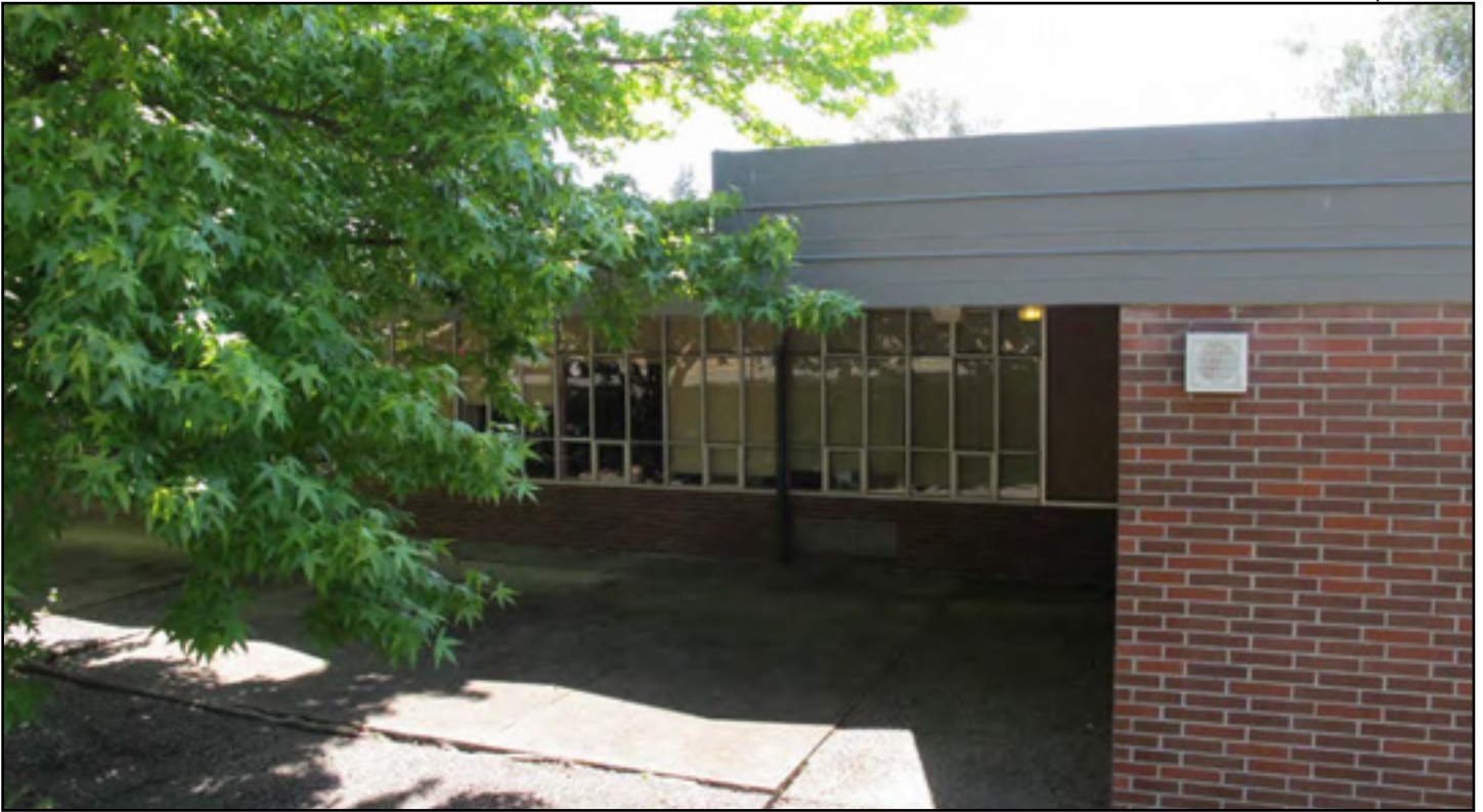
Figure 32. Edmund S. Meany Junior High, 1962 addition, Unit A, eastern façade, northern end (1962 Mahlum Addition)
