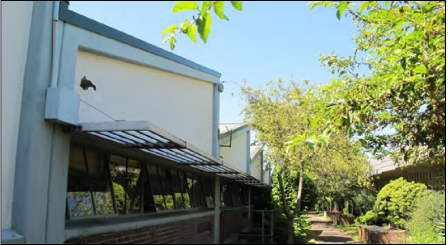
Figure 26. Edmund S. Meany Junior High, 1955 addition, viewing north at northern courtyard (1955 Maloney Addition)
