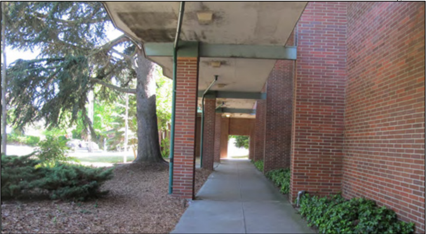
Figure 52. Edmund S. Meany Junior High, 1962 addition, Unit C, viewing south at eastern façade (1962 Mahlum Addition)
