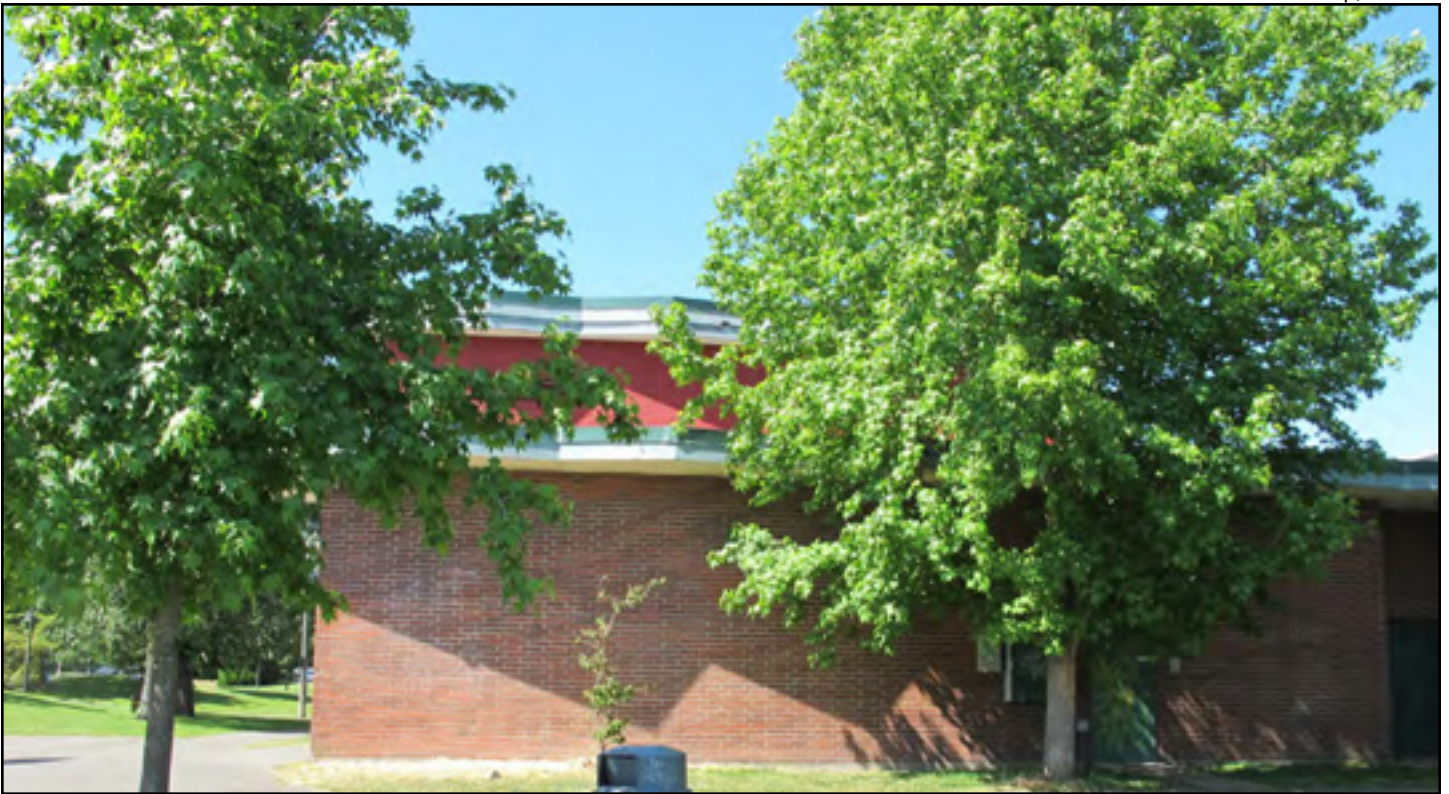
Figure 65. Edmund S. Meany Junior High, 1962 addition, Unit E, southern façade (1962 Mahlum Addition)
