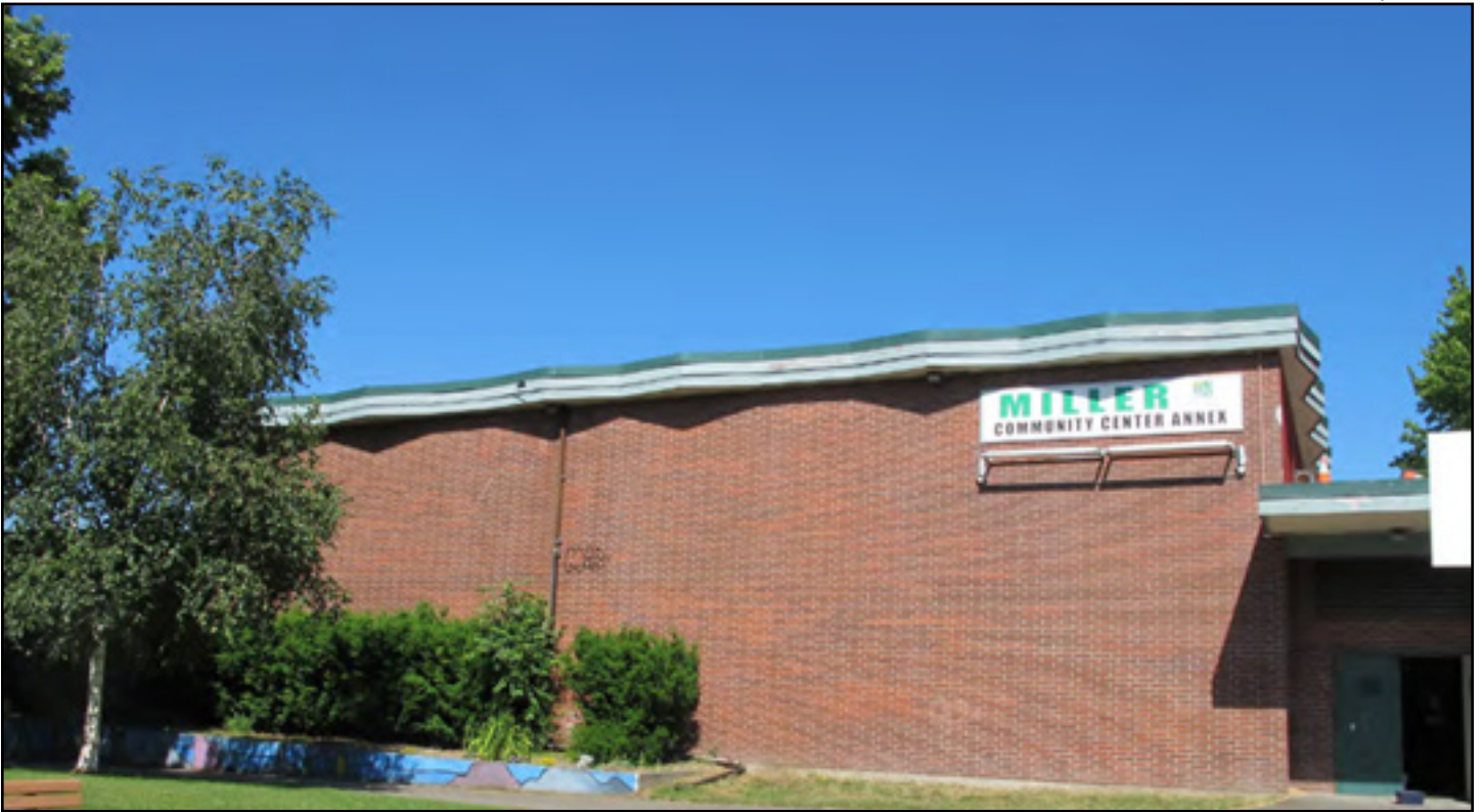
Figure 64. Edmund S. Meany Junior High, 1962 addition, Unit E, western façade (1962 Mahlum Addition)
