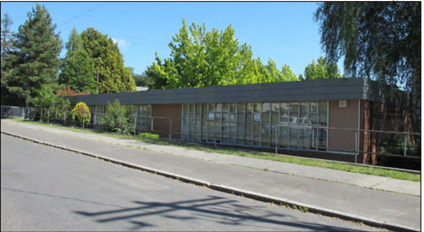
Figure 31. Edmund S. Meany Junior High, 1962 addition, Unit A, northern façade (1962 Mahlum Addition)
