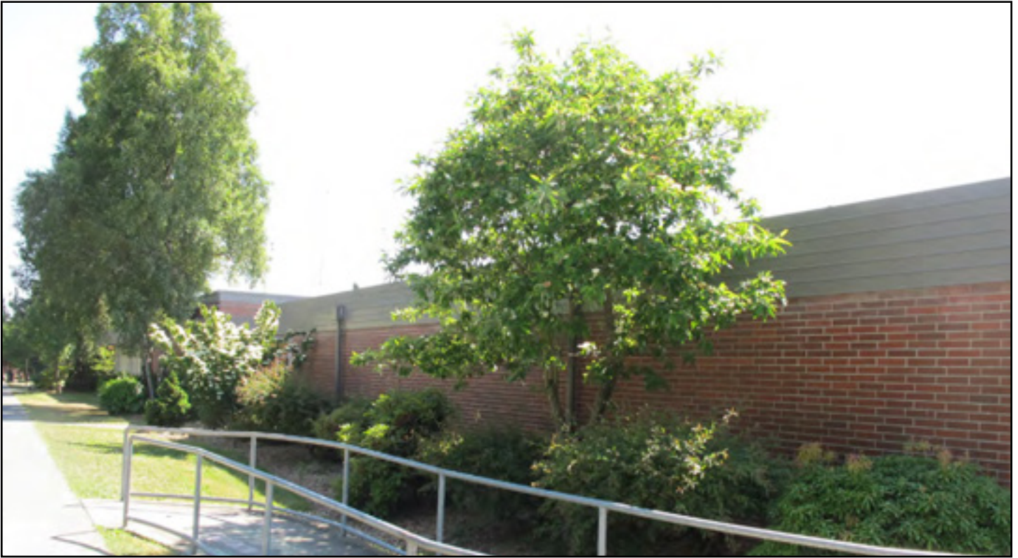
Figure 38. Edmund S. Meany Junior High, 1962 addition, Unit B, eastern façade (1962 Mahlum Addition)
