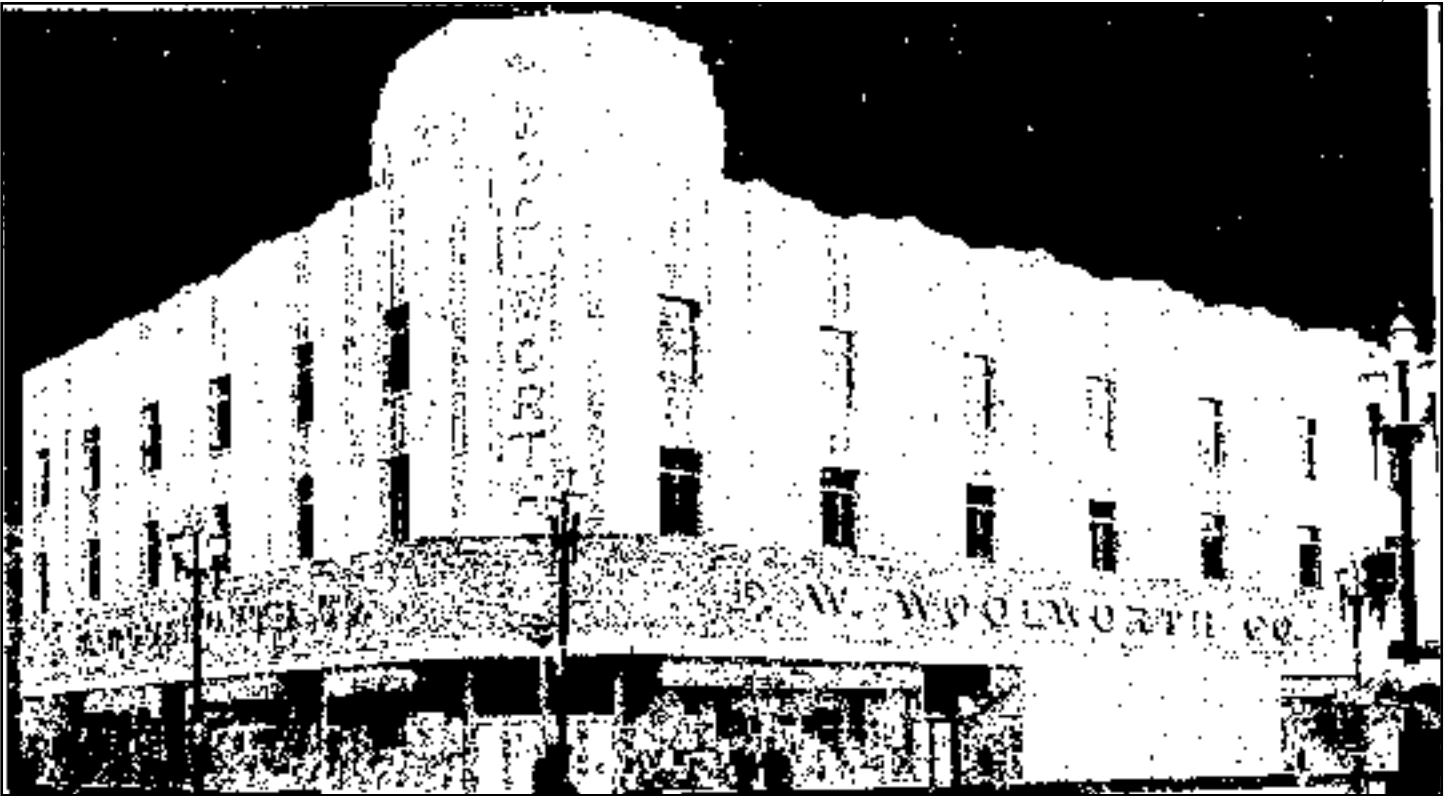
Figure 134. Woolworth store at Third Avenue and Pike Street, Seattle (1940, J.B. Warrack, contractors)
