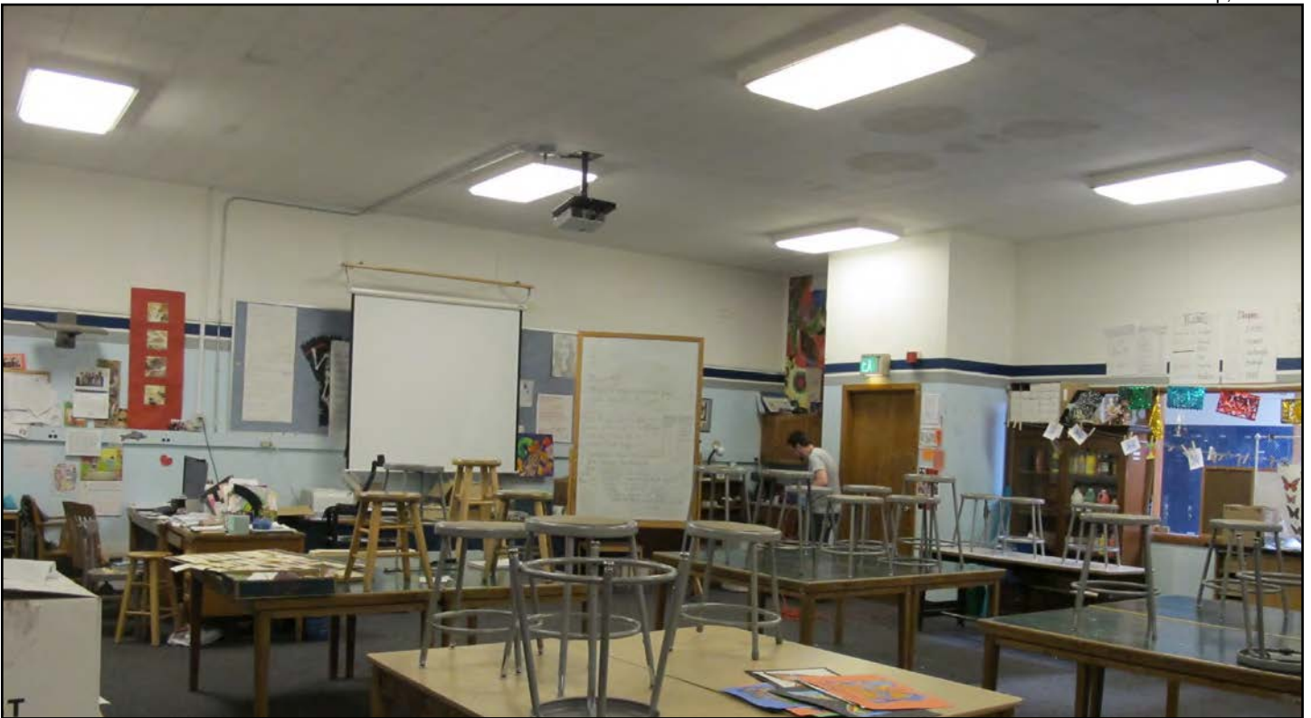
Figure 47. Edmund S. Meany Junior High, 1962 addition, Unit B, typical classroom (1962 Mahlum Addition)
