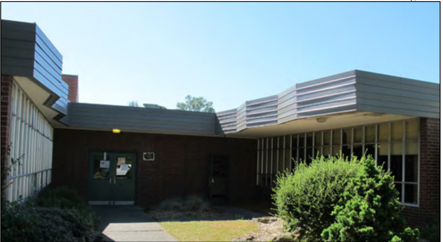
Figure 39. Edmund S. Meany Junior High, 1962 addition, Unit B, eastern façade courtyard (1962 Mahlum Addition)
