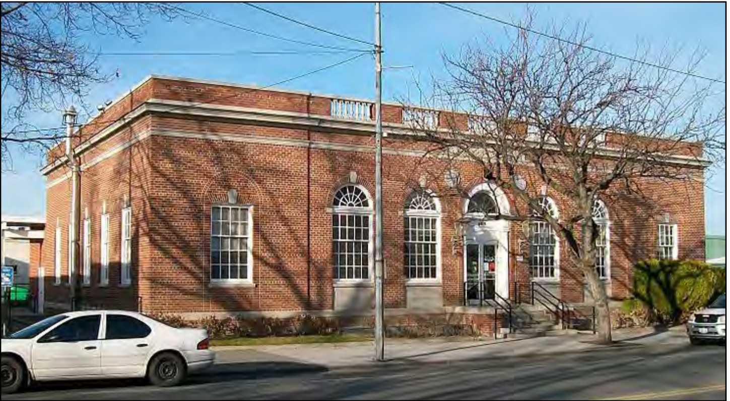
Figure 137. U.S. Post Office, Pasco, WA (1932, Louis A. Simon, architect for U.S. Department of the Treasury; Hedeem Construction Co., contractor)
