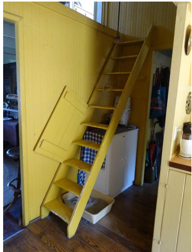
C31. (Left) View east, showing the ship's ladder to the second floor. The first-floor hall accesses the bathroom and another bedroom. (July 10, 2020)
