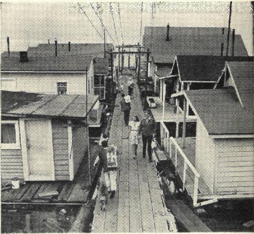
FLOATING BOARDWALK runs between houseboats. Gas and water pipes, beneath walk, are hooked to houseboats by hoses. Electric wires run overhead.
