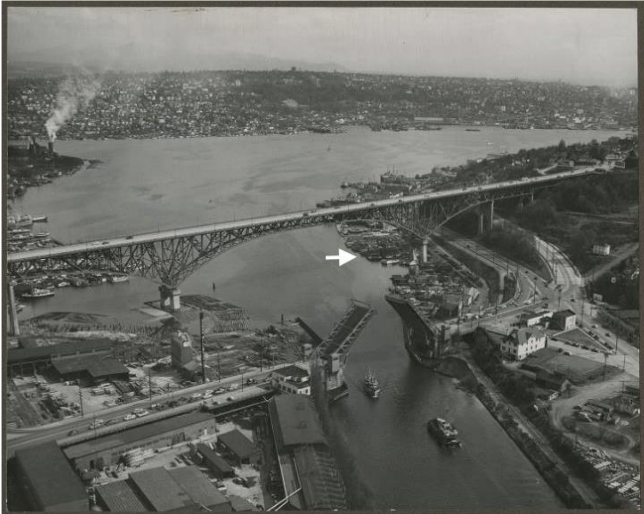
A10. Aerial Photograph of George Washington Memorial Bridge (Aurora Avenue), 1950. The arrow points to the Wagner Houseboat (close-in view is below). The camera is facing east. Source: Seattle Public Library, Seattle Historical Photograph Collection, 20061.
