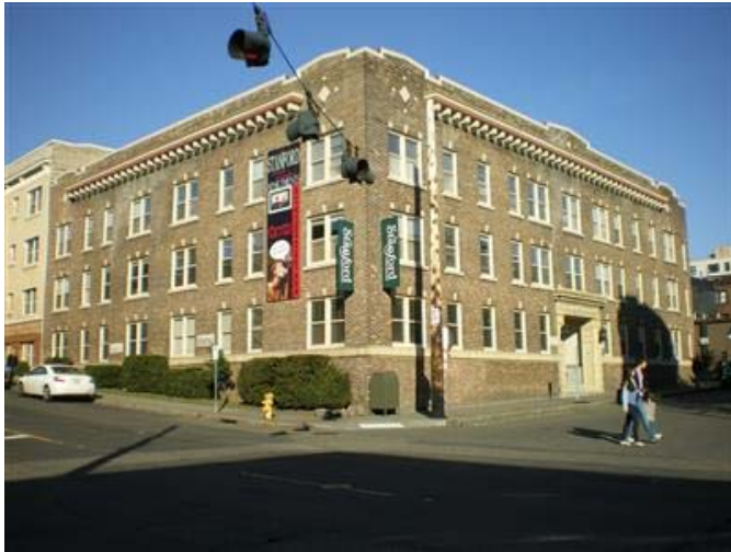
Figure 60. Above, the nearby Smart/Sanford Apartments, 1305 NE 43 rd (King County Assessor). This is one of a half-dozen apartment buildings in the University District designed by Roberts in the 1920s.
