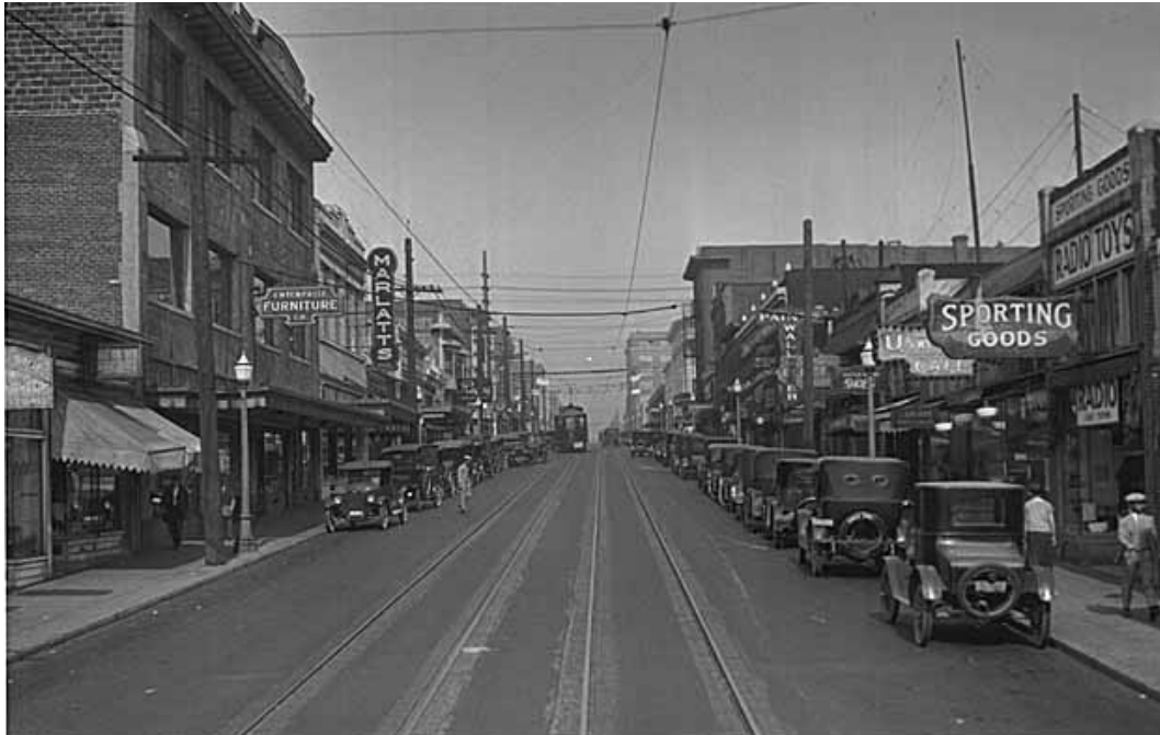
Figure 8. Above, looking north on University Way NE in ca. 1925 (MOHAI, 3409).
