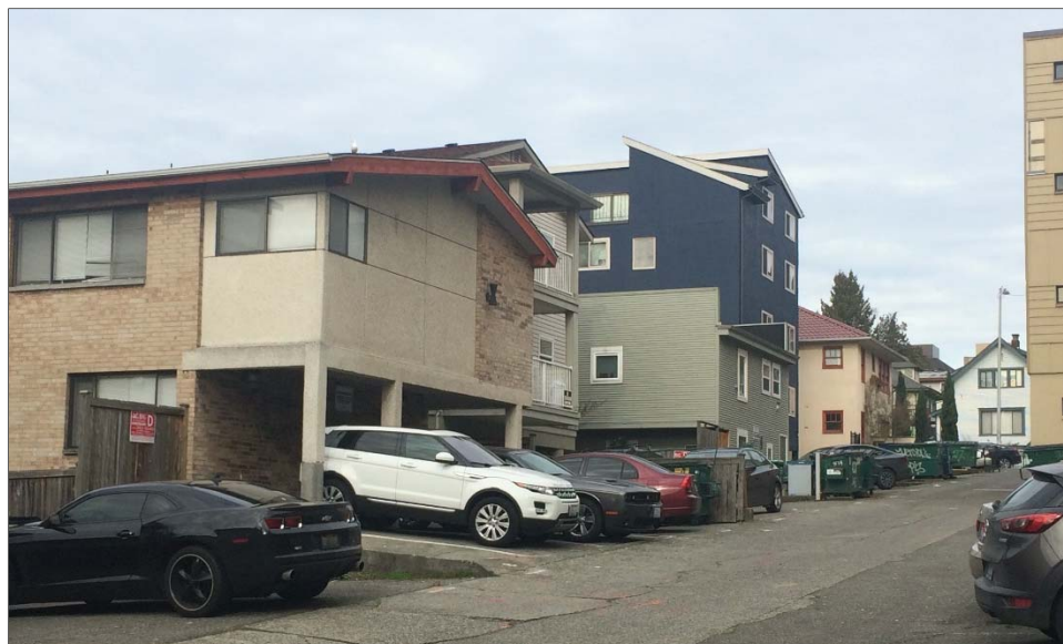
Figure 30. Below, looking generally north along the alley between 12 th and Brooklyn Avenues NE. A portion of the Villa Camini is visible at the end, on the west (left) side of the alley.
