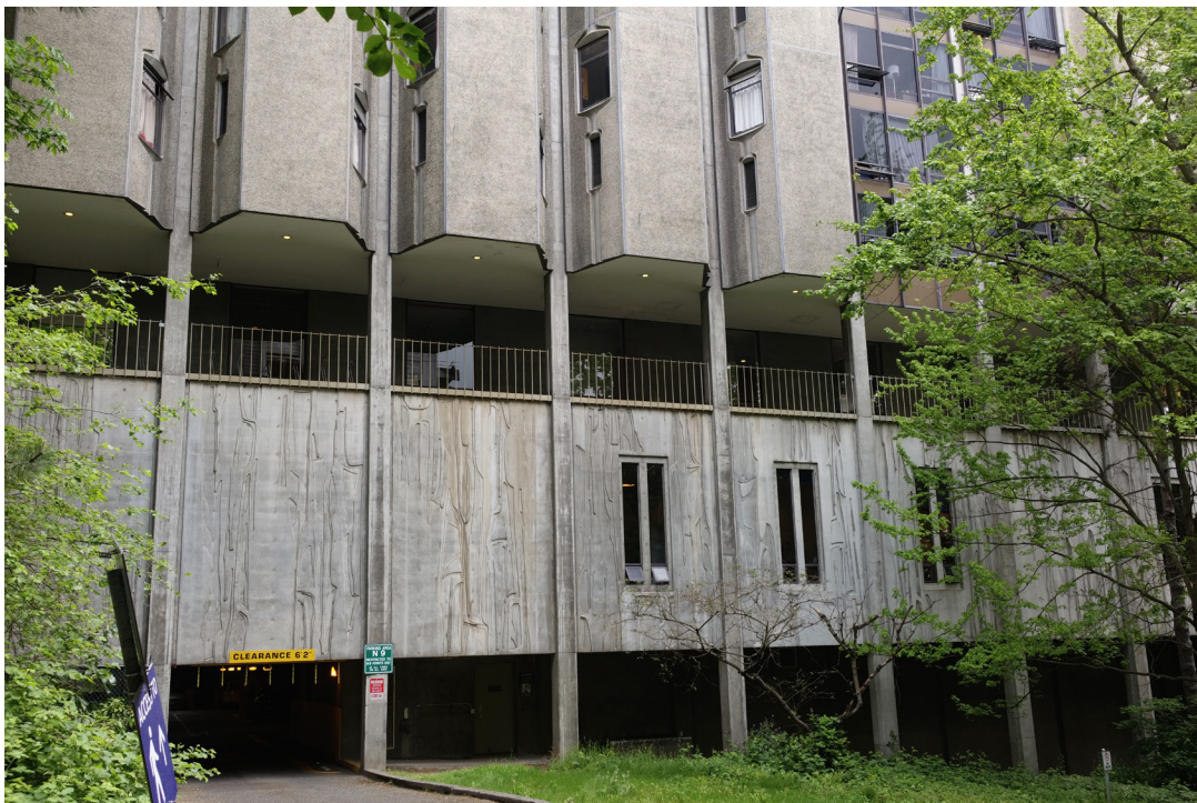
Figure 23. View of the base pre-cast concrete panels (south elevation) and an entrance to parking located under the south tower.
