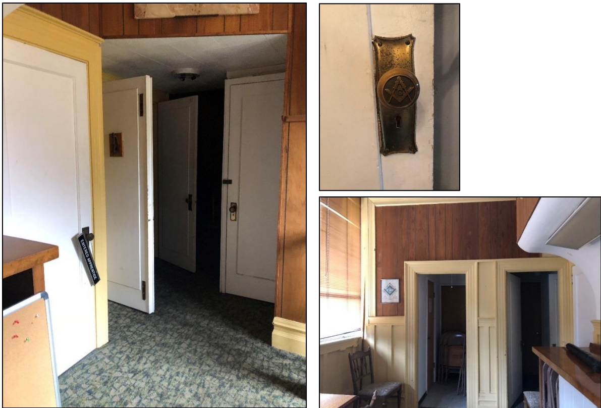
Figures 52 & 53. Above left and right, the second floor vestibule space outside of the Lodge Room. Figure 54. Top right, a standard doorknob with the iconography.
