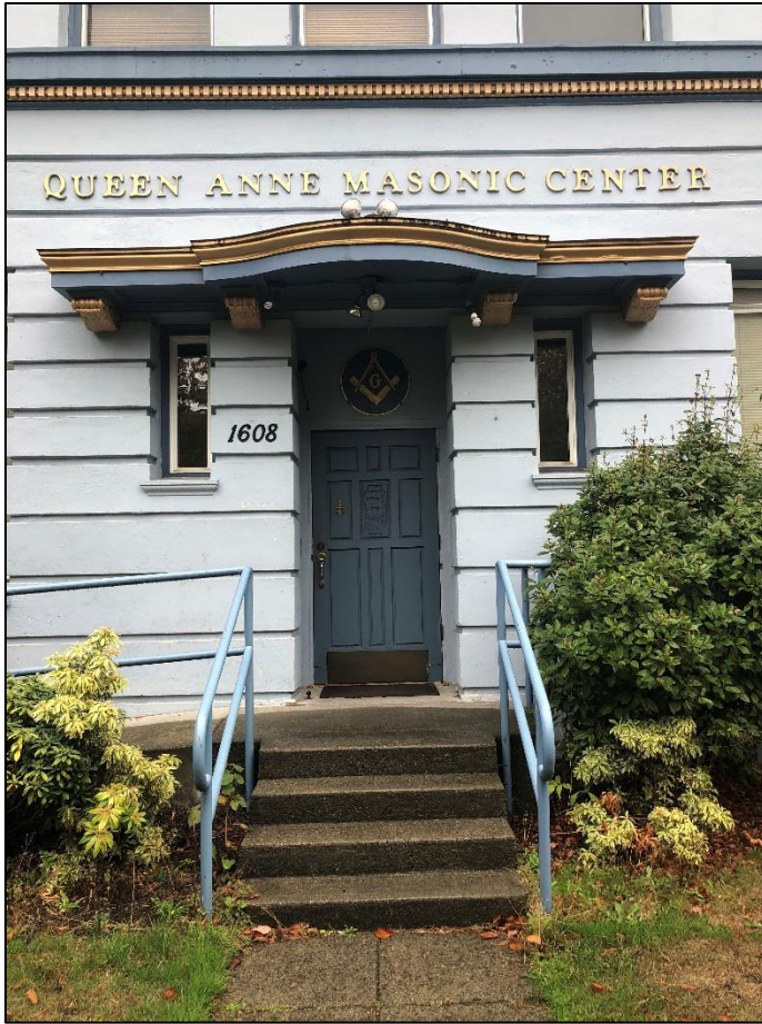
Figure 42. Left, a detail view of the primary entry.
