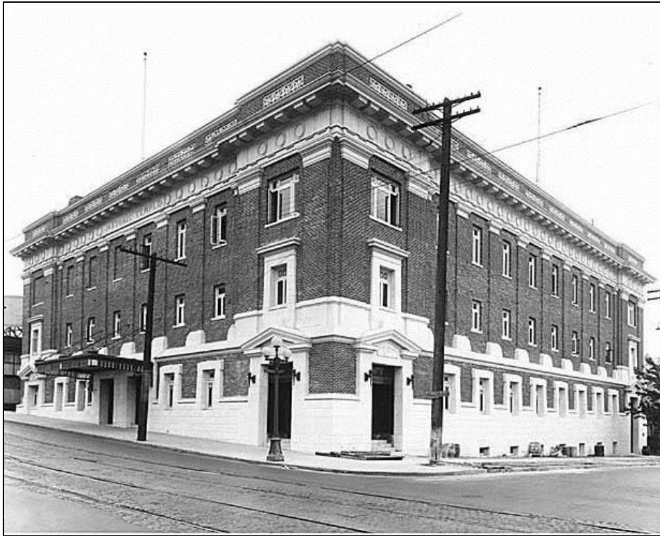
Figure 26. Above, the Masonic Temple (currently the Egyptian Theatre) at the corner of Harvard Avenue and E Pine Street, in ca. 1916 (MOHAI no.1983.10.10333).
