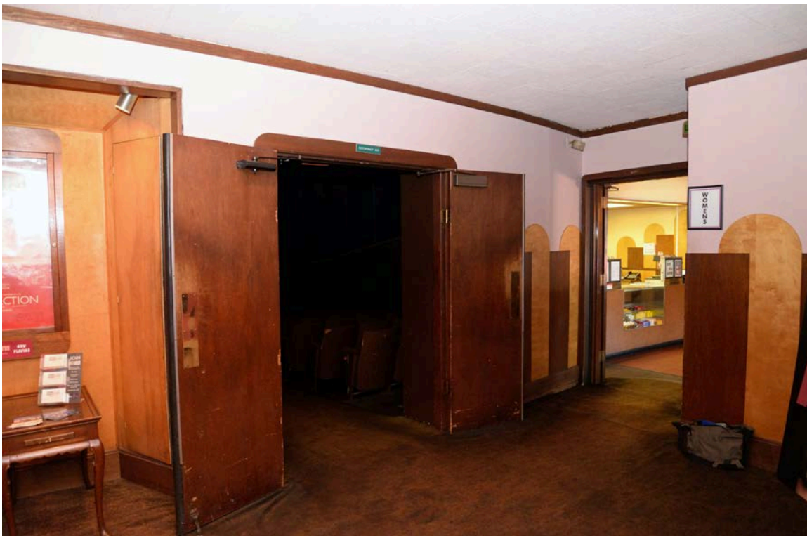
Figure 37. Interior – West Auditorium and Concession Doors at South Wall of Lobby, View Southwest
