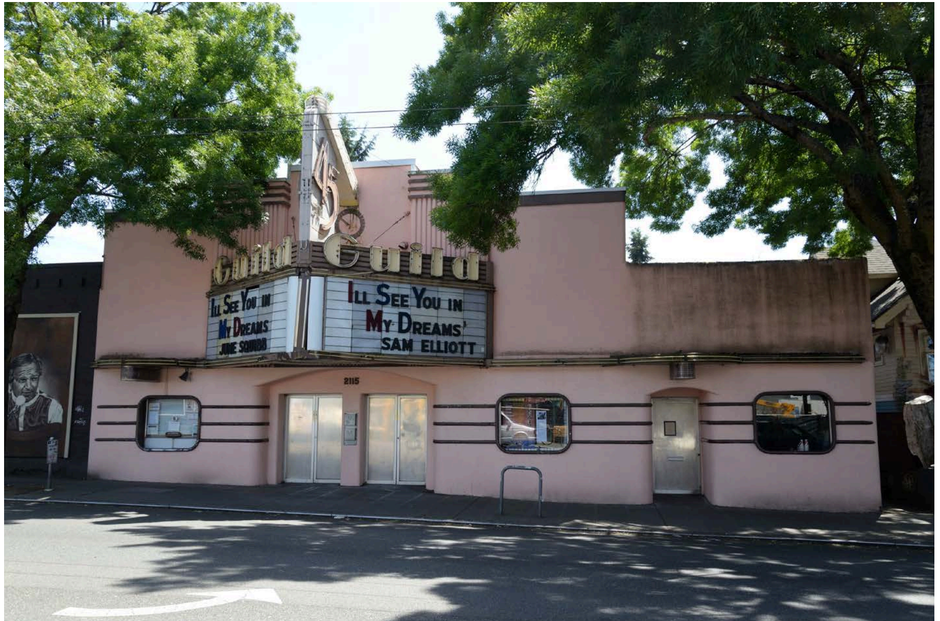
Figure 15. Exterior – North Elevation, View South
