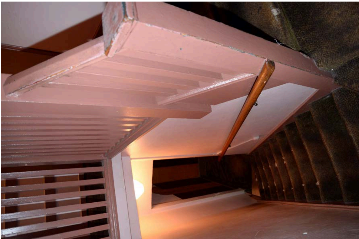
Figure 40. Interior – Staircase to Second Floor Men’s Restroom, View South
