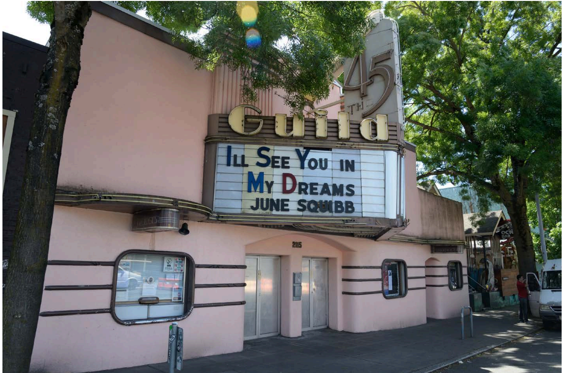
Figure 14. Exterior – North Elevation, View Southwest
