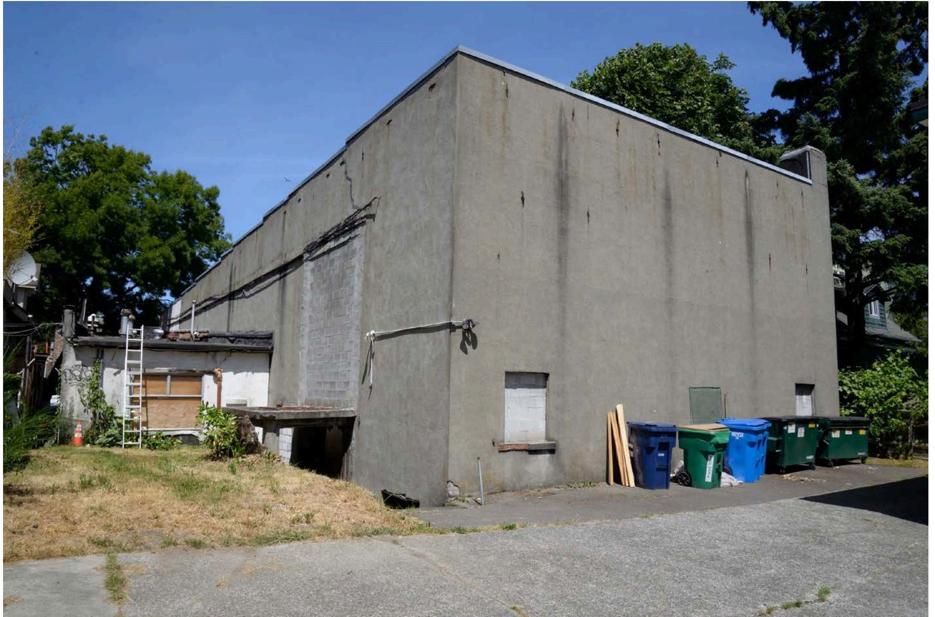
Figure 20. Exterior – West and South Elevations, View Northeast
