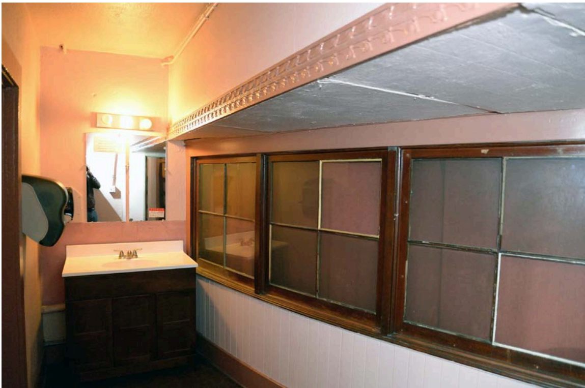
Figure 51. Interior – Second Floor Women’s Restroom (former lounge), View East
