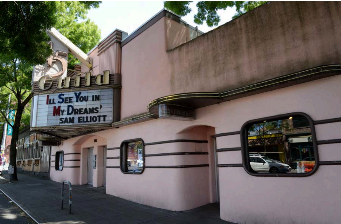
Figure 29. Exterior – North Elevation, View Southeast
