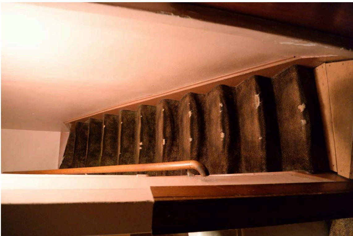
Figure 39. Interior – Staircase to Second Floor Men's Restroom, View North
