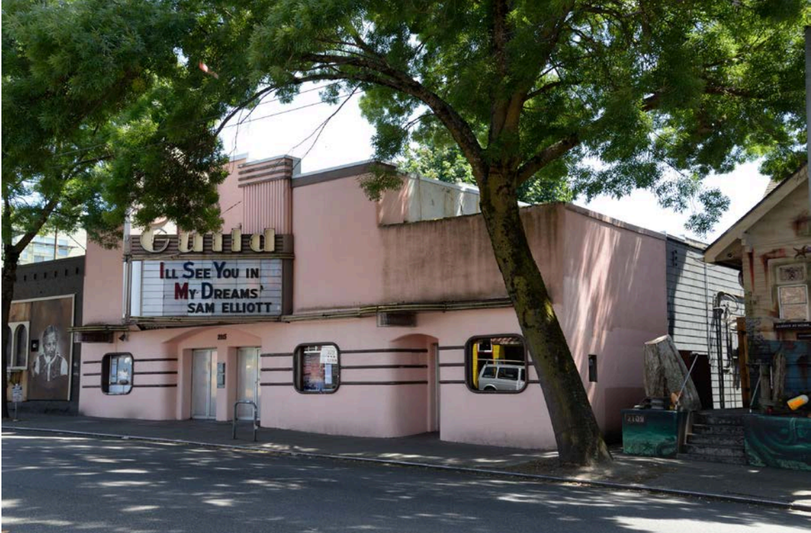
Figure 28. Exterior – North Elevation, View Southeast
