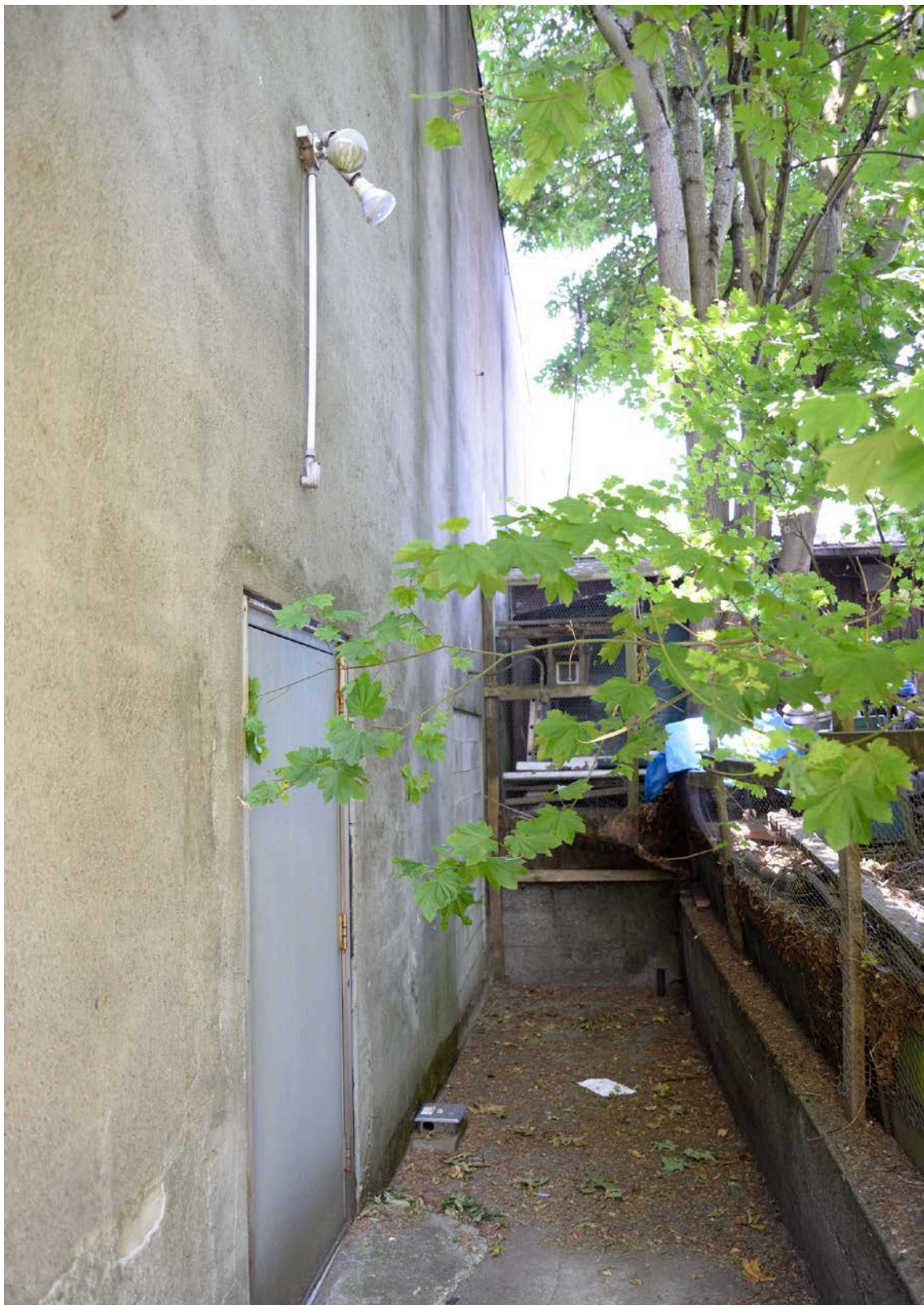
Figure 21. Exterior – East Elevation, View North
