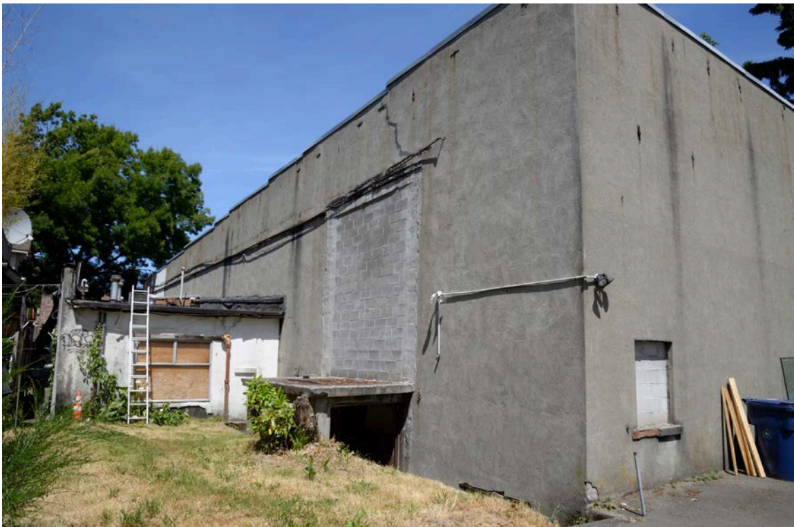
Figure 33. Exterior – South and West Elevations, View Northeast
