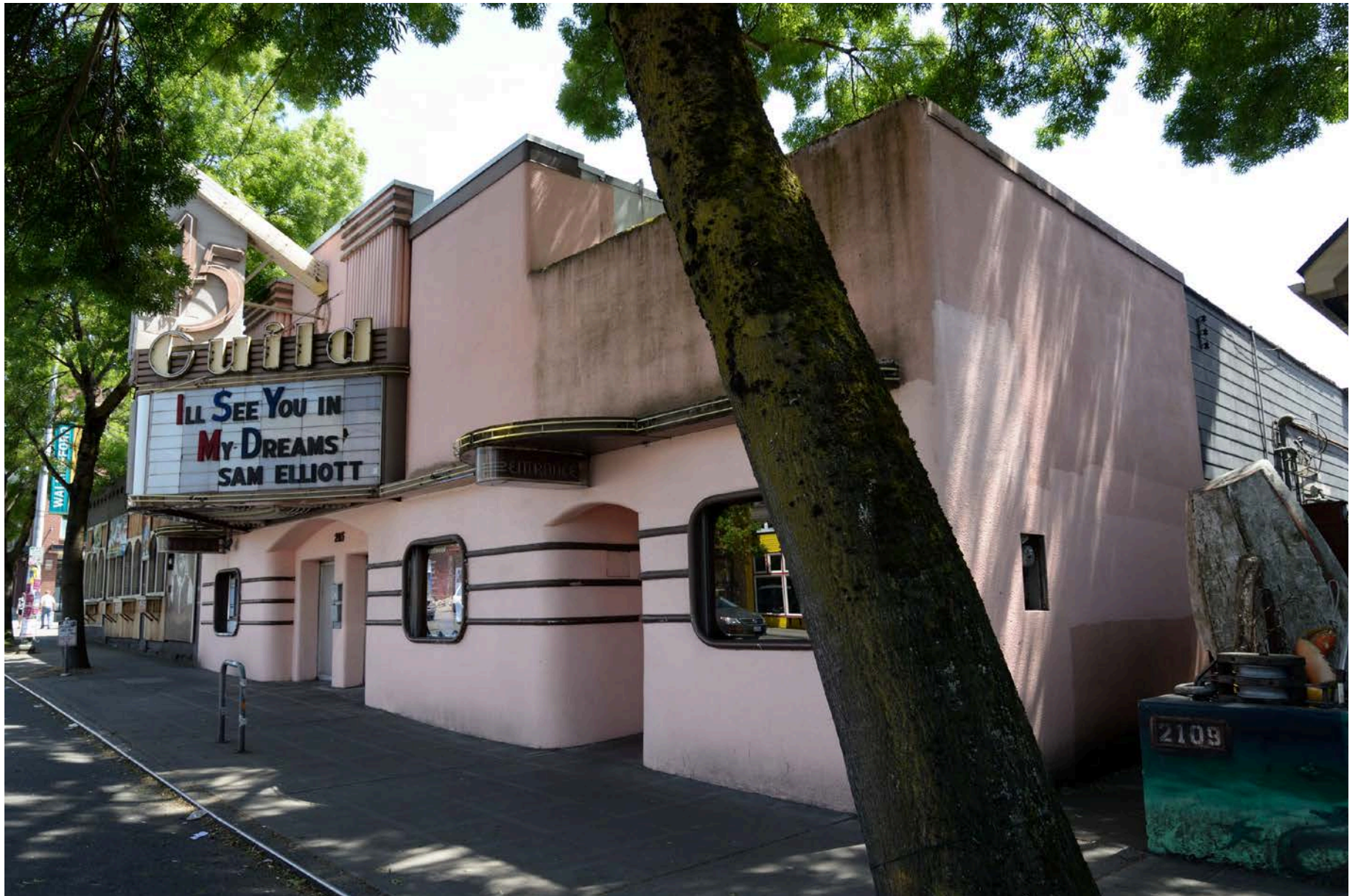
Figure 16. Exterior – North Elevation, View Southeast
