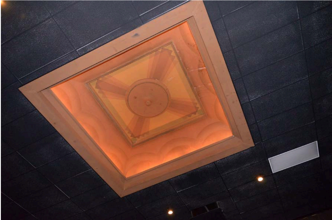
Figure 58. Interior – Ceiling Vault in Auditorium, View Southeast
