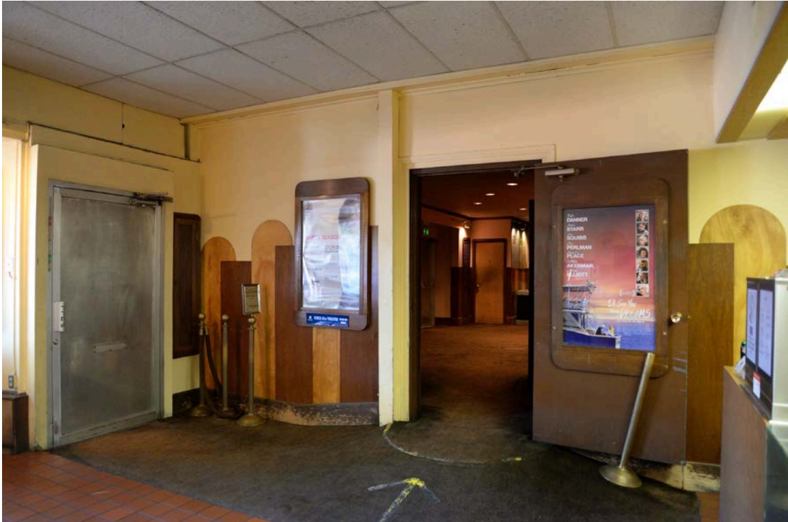
Figure 54. Interior – East Wall of the Concessions Lobby, View East
