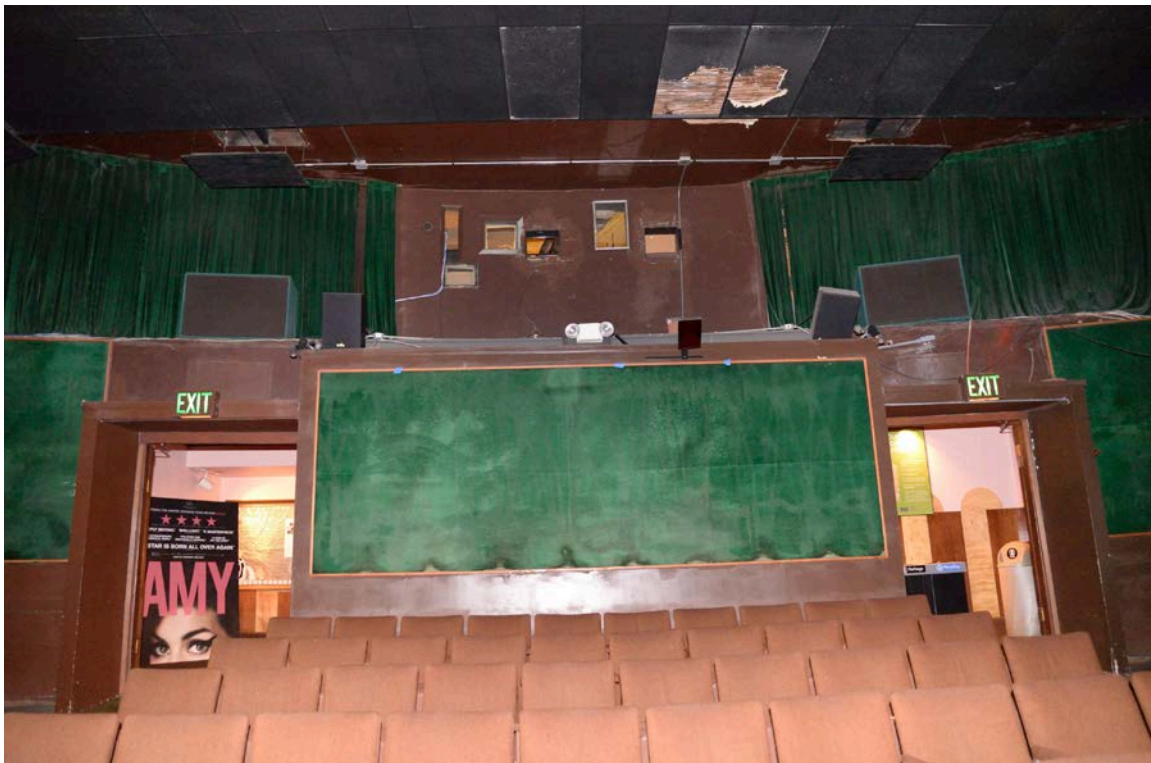
Figure 59. Interior – North Wall of Auditorium, View North
