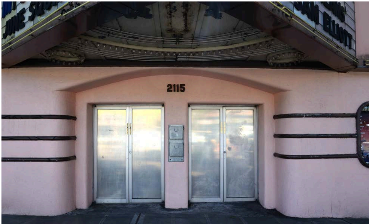
Figure 31. Exterior – Entrance Vestibule and Doors at North Elevation, View South
