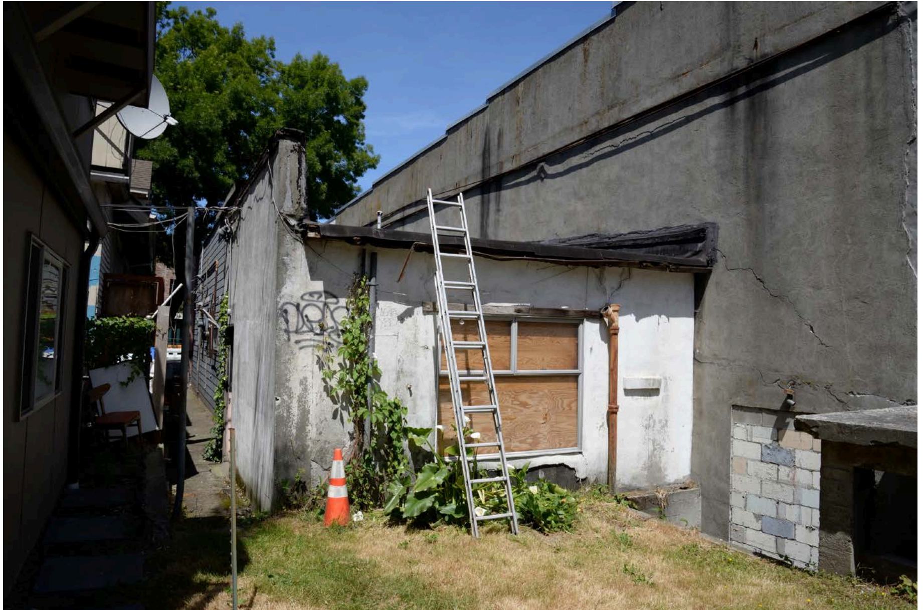
Figure 19. Exterior – West and South Elevations of 2113-2113 ½ N. 45th Street, View Northeast
