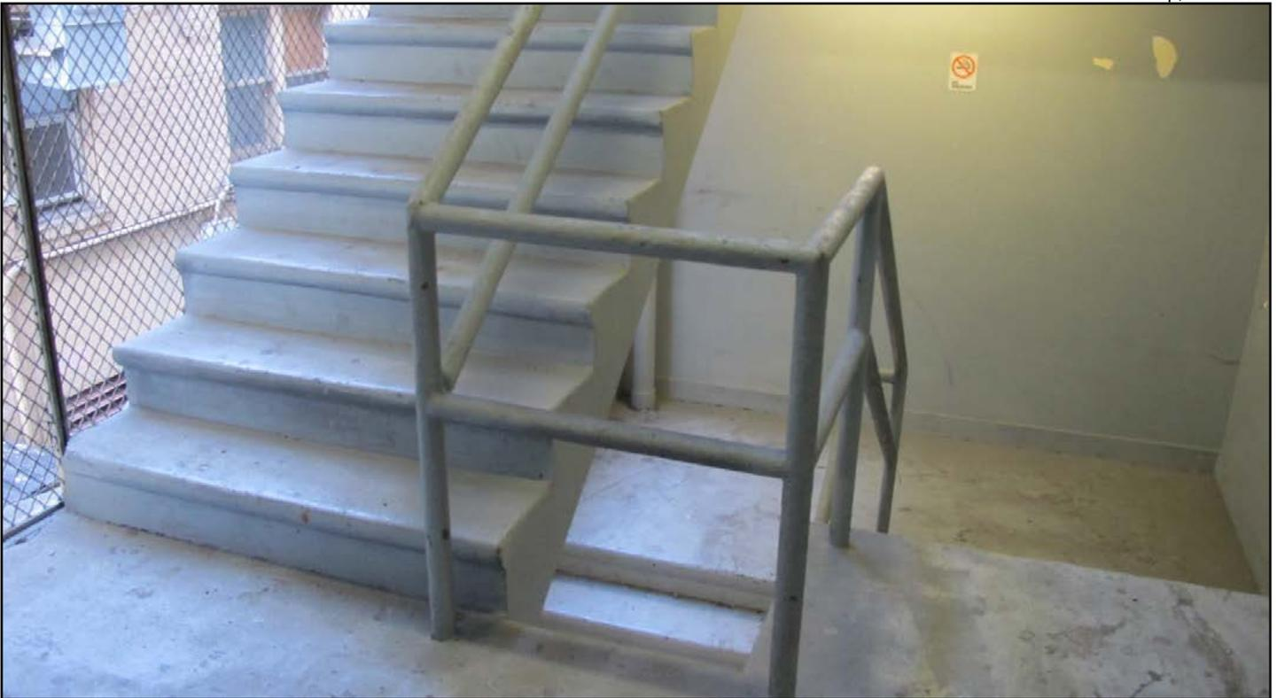
Figure 35 • 2005 Fifth Avenue, open-air fire egress stair on alley side of building
