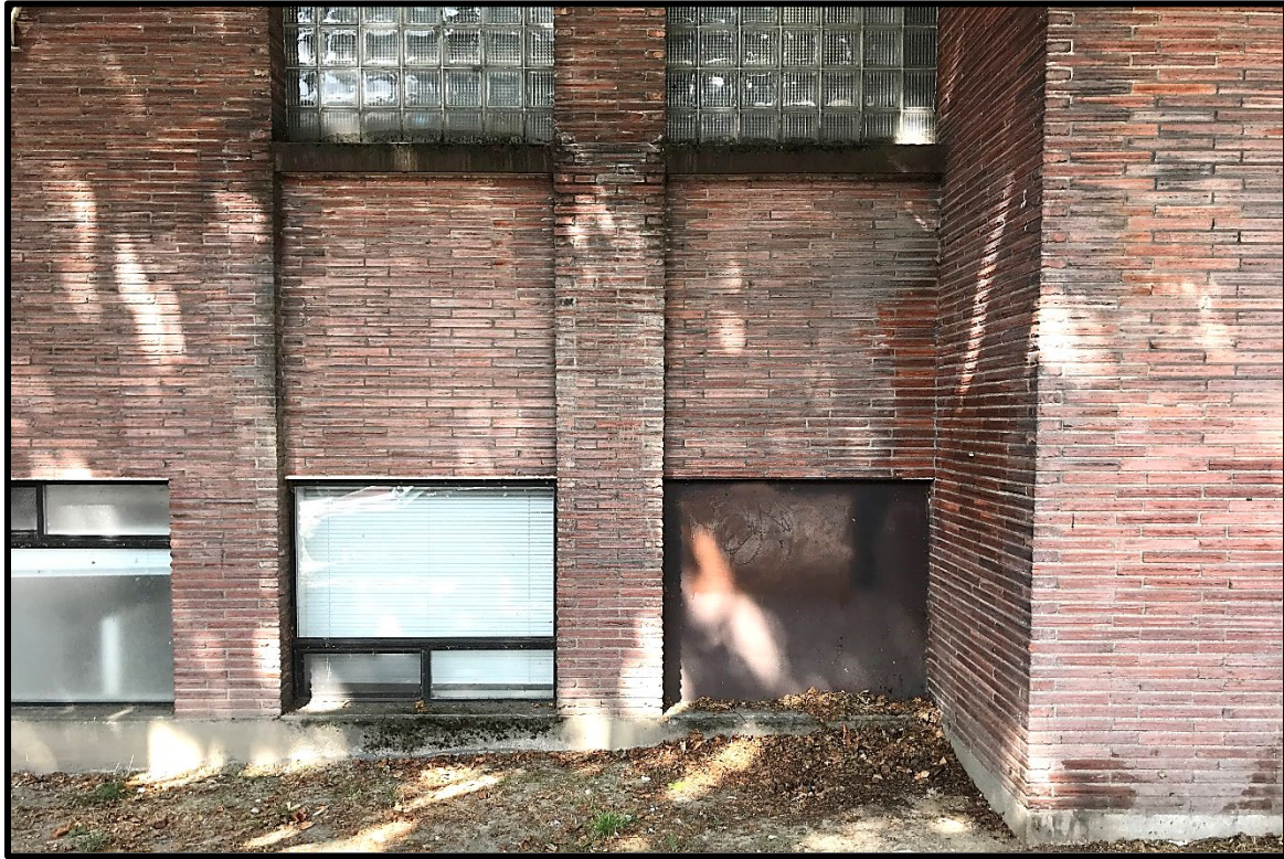
Figure 61: Detail of modified windows at east façade of subject building.
