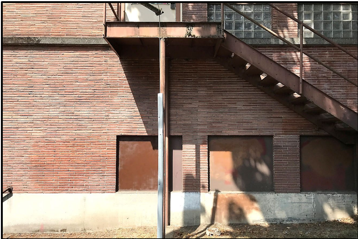
Figure 66: Detail of modified windows at east façade of subject building.
